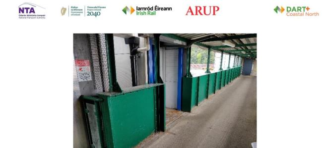
Figure 3: OBB81 modification to bridge at north-eastern end to allow access to OBB81C
