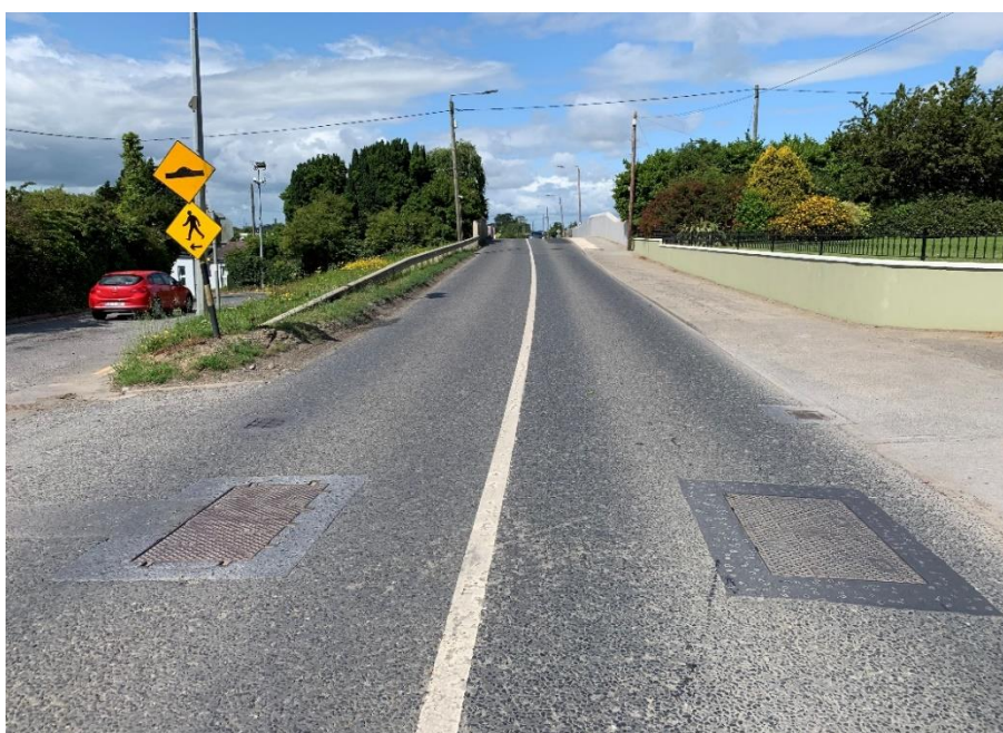
Figure 7: Approach to OBB 39 from the East (source: Iarnród Éireann)
