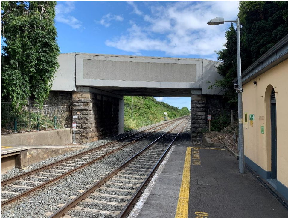
Figure 2: Bridge elevation looking towards Belfast (source: Iarnród Éireann)
