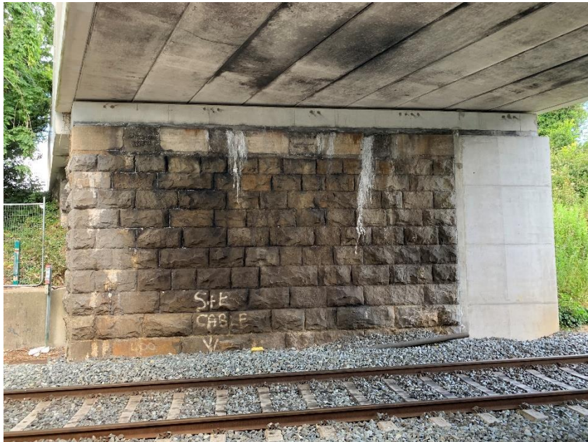
Figure 3: View of western bridge abutment (source: Iarnród Éireann)
