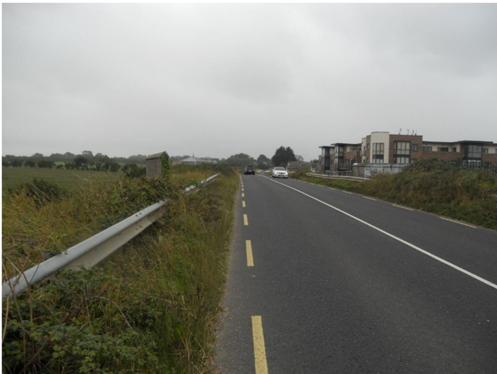
Figure 7: Approach to OBB 78 from the North East (source: Iarnród Éireann)
