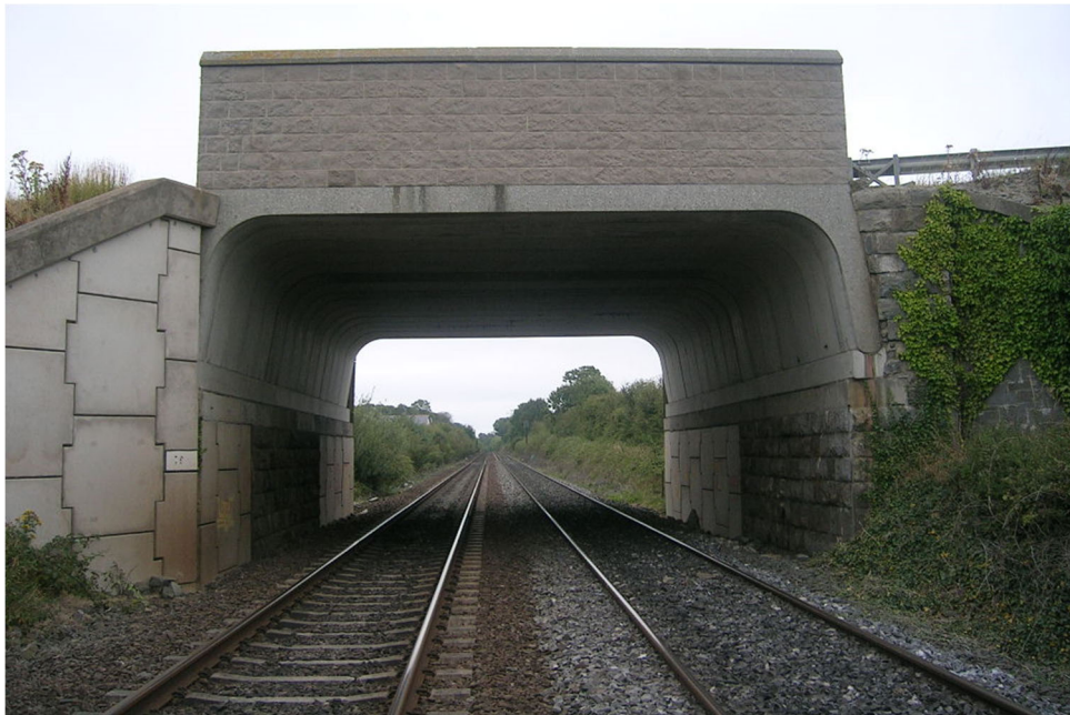
Figure 2: Bridge elevation looking towards Belfast (source: Iarnród Éireann)
