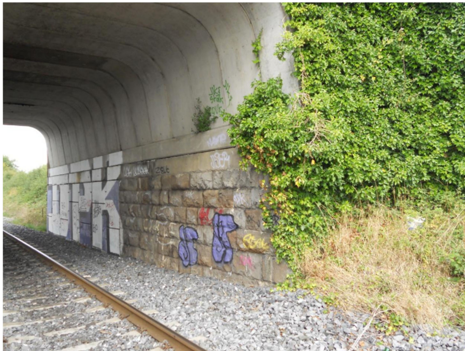
Figure 3: View of northern bridge abutment (source: Iarnród Éireann)
