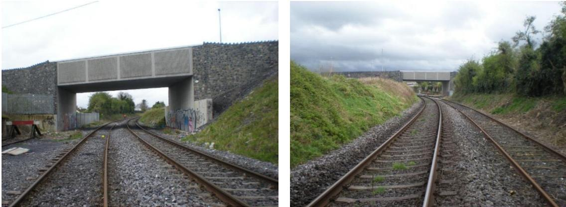
**Figure 4-26** Left photo: siding to be converted into a running line. Right photo: siding with wood sleeper and without cant
