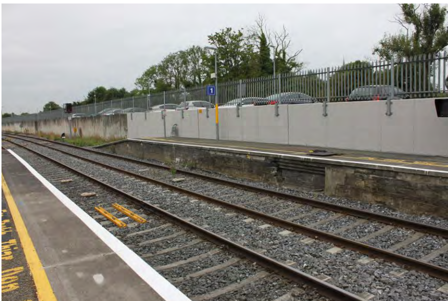
Figure 5-338 End of east platform (Platform 1)
