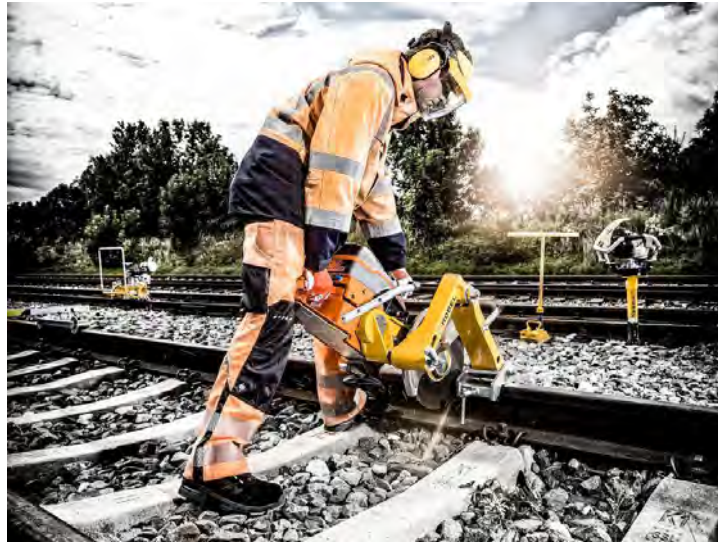
Figure 5-13 Rail cutting
