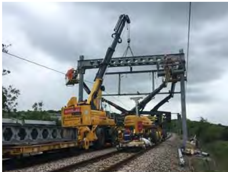
Figure 5-82 Gantry installation
