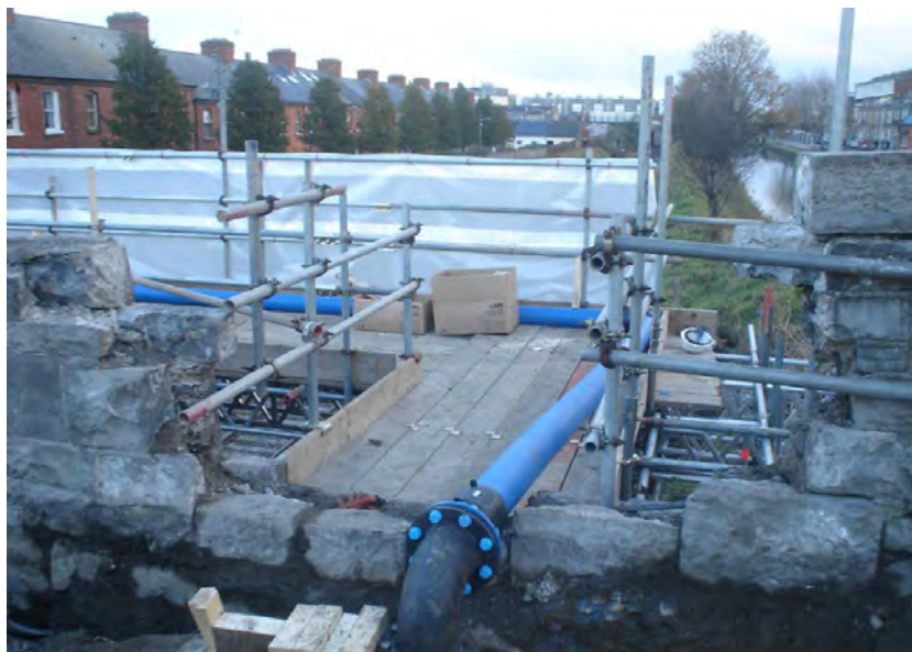
Figure 5-7 Temporary diversion along scaffolding
