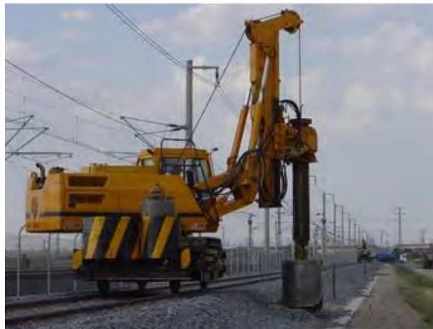
Figure 5-77 Foundation drilling
