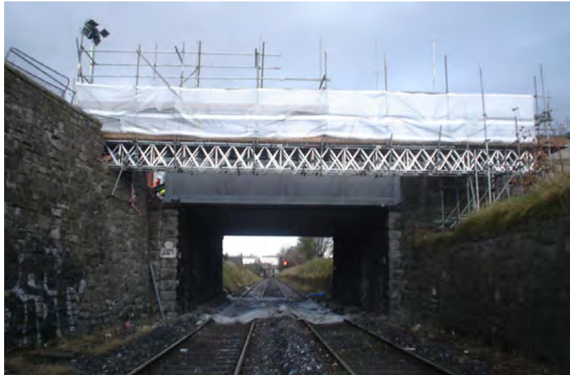
Figure 5-6 Scaffolding for temporary diversion
