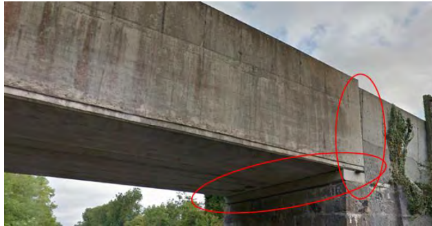
Figure 5-390 Joints to be demolished at abutment
