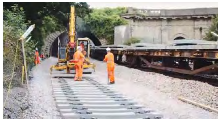
Figure 5-26 Sleeper laying
