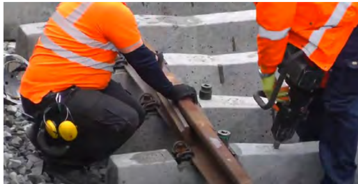
Figure 5-20 Provisional track panel joint
