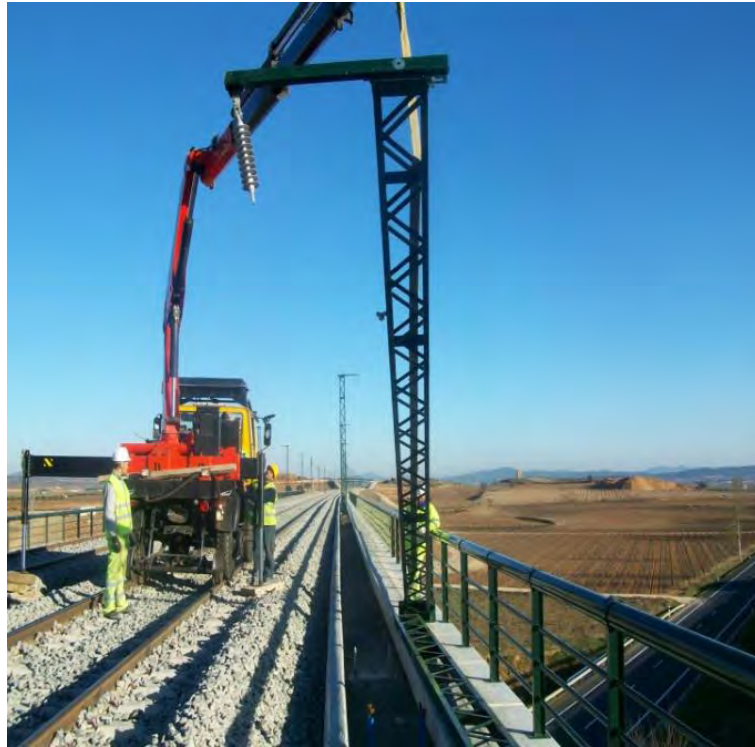
Figure 5-81 Mast installation
