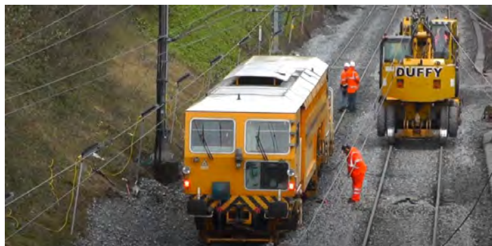
Figure 5-22 Ballast tamping
