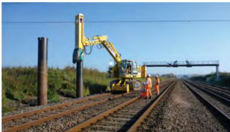
Figure 5-79 Installation of steel piles
