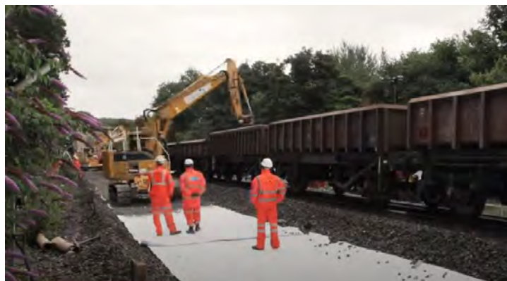
Figure 5-17 Ballast laying
