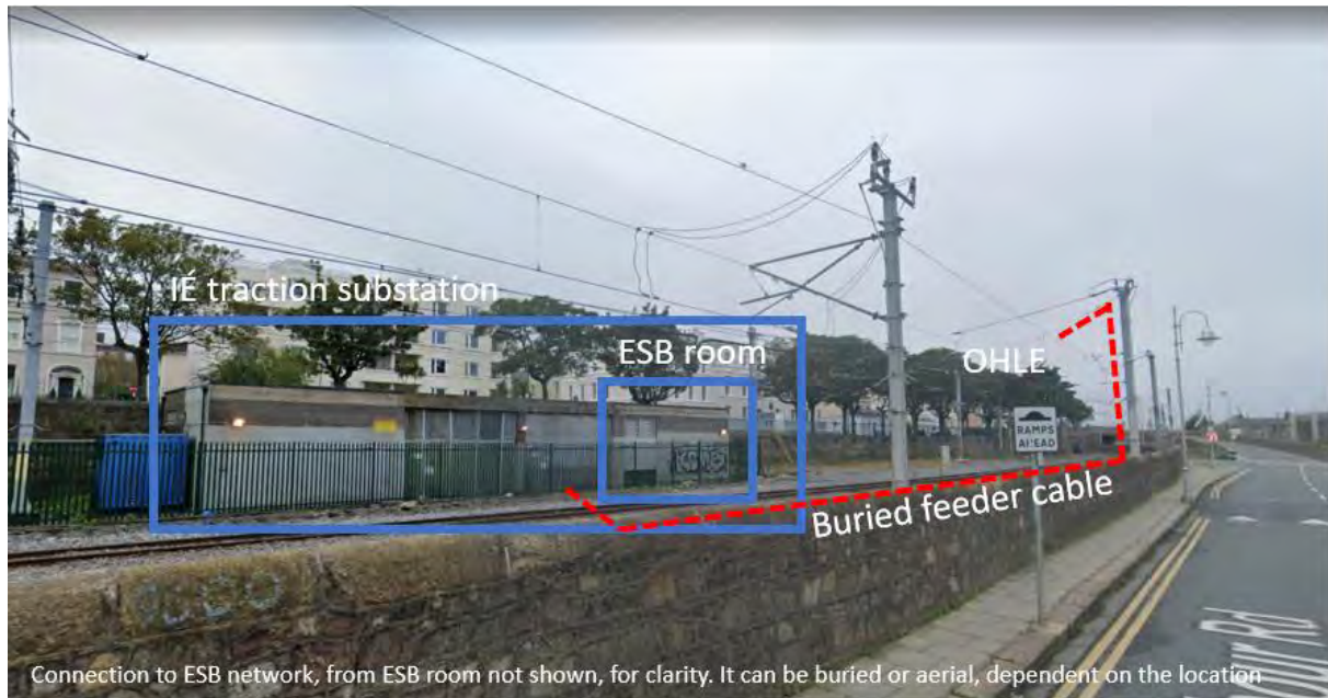
Figure 5-62 Traction substation connections
