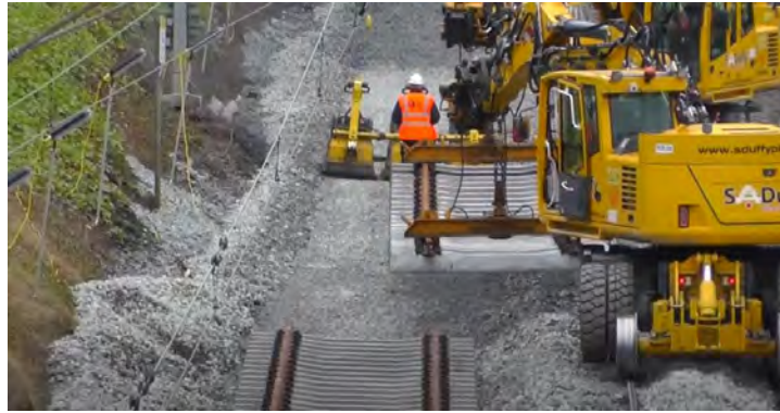
Figure 5-19 Track panel installation
