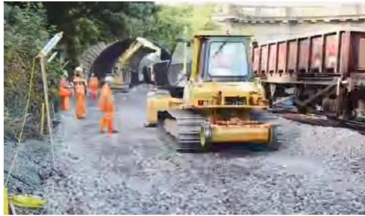
Figure 5-25 Ballast laying and compaction
