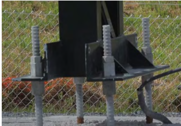
Figure 5-83 Foundation anchor for masts
