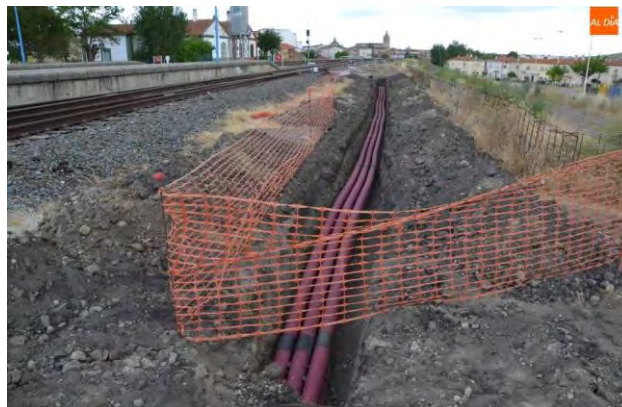
Figure 5-75 Example of buried utilities to be diverted
