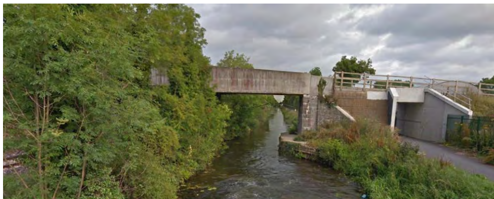
Figure 5-389 View of OBG24 from the Royal Canal
