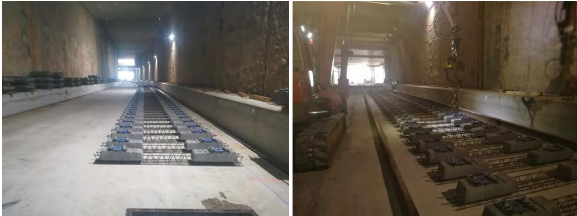
Figure 5-29 Sleeper laying on top of structural slab
