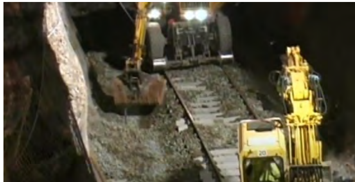
Figure 5-21 Ballast laying – second layer
