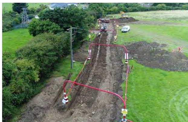
Figure 5-76 Aerial example of utilities to be diverted
