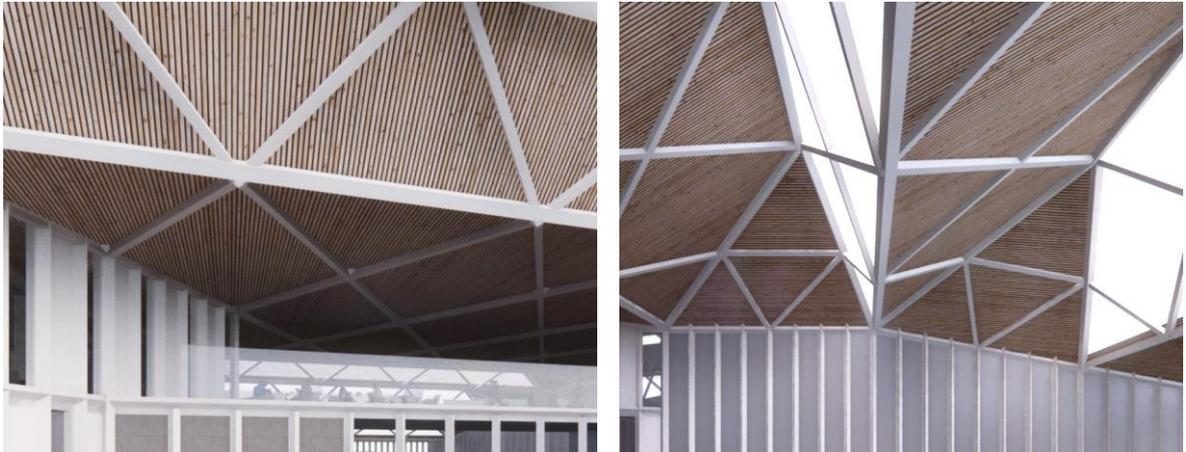
**Figure 48. Wooden slats ceiling on main entrance area (left) and opaque gables (right)**
