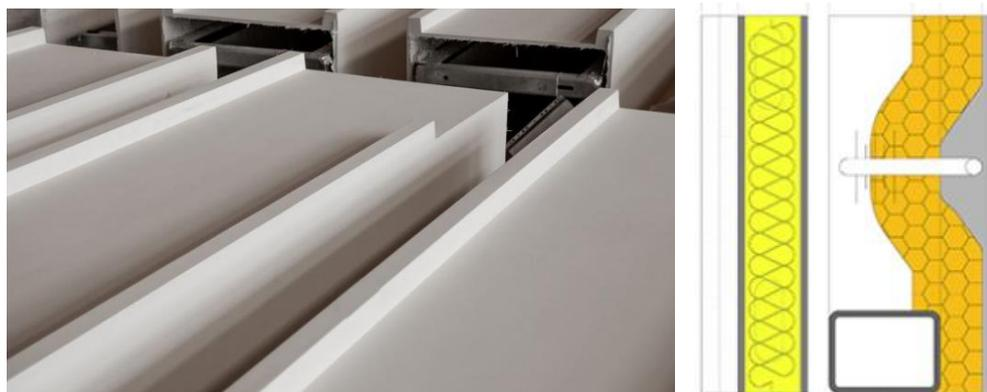
Figure 60. Mockup of GRC façade. Section detail of GRC wall
