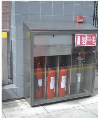
**Figure 93 Fire extinguisher and fire alarm equipment.**
