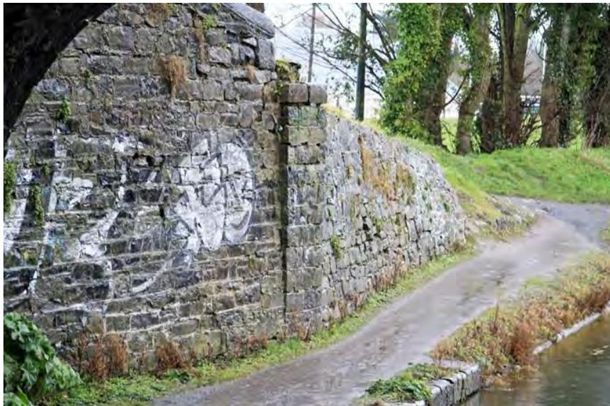
**Figure 316 Eastern wing wall on northern side of canal bridge**
