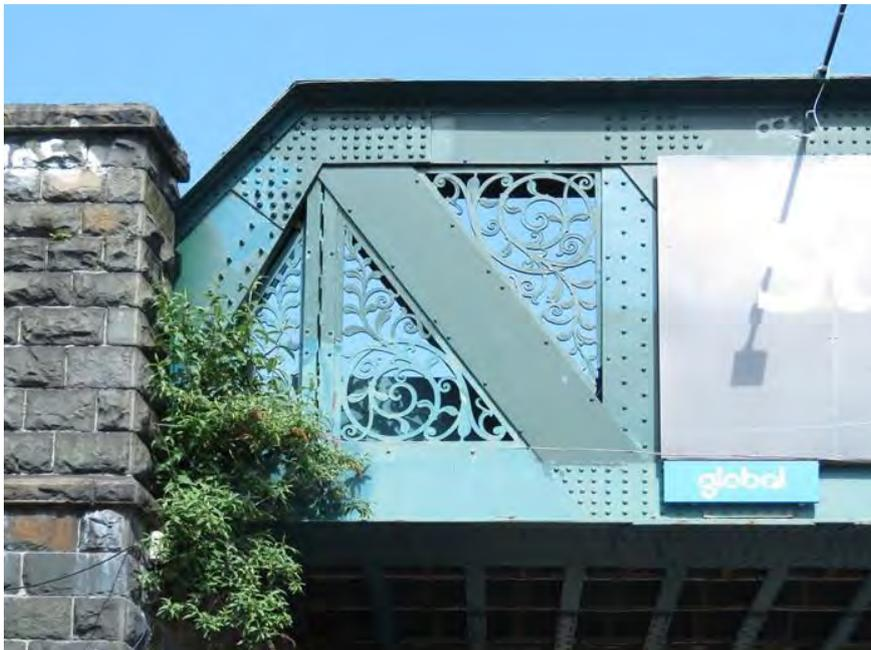
**Figure 499** Cast-iron decorative panels at western end of bridge
