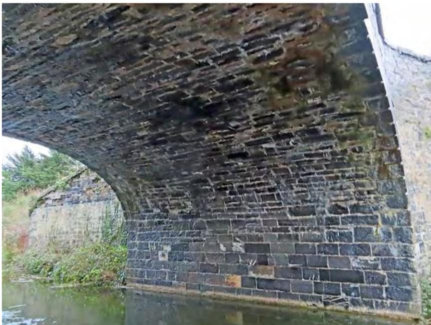
**Figure 294** Barrel of vault
