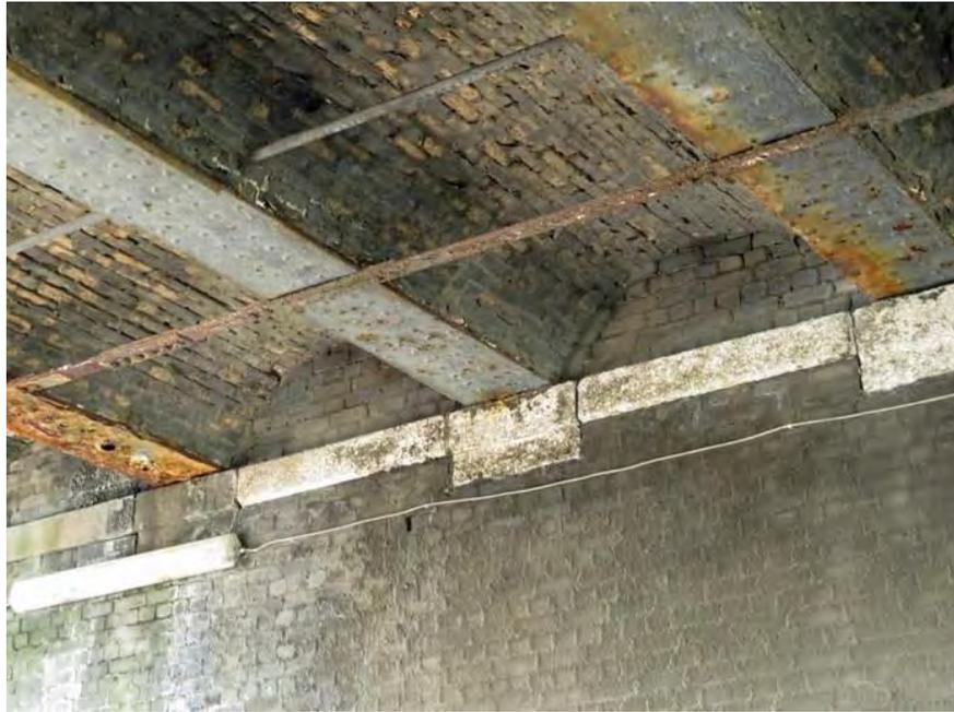
**Figure 473 Padstones and string course beneath beams**
