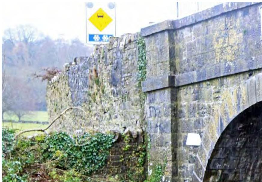
**Figure 376 Pier and retaining wall on eastern side of railway bridge**
