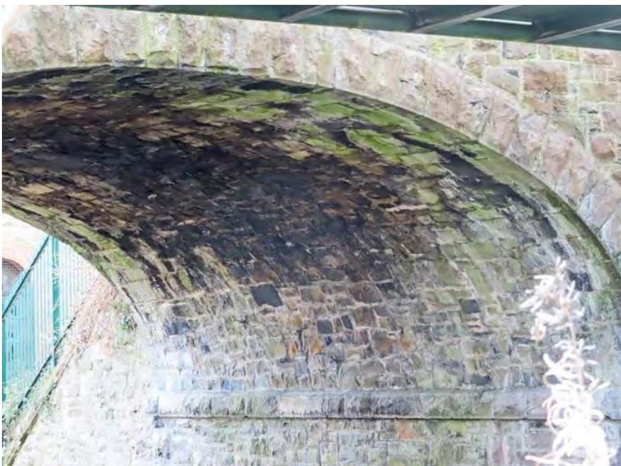
**Figure 456 The arch ring and the barrel of the vault of Dunboyne Bridge**
