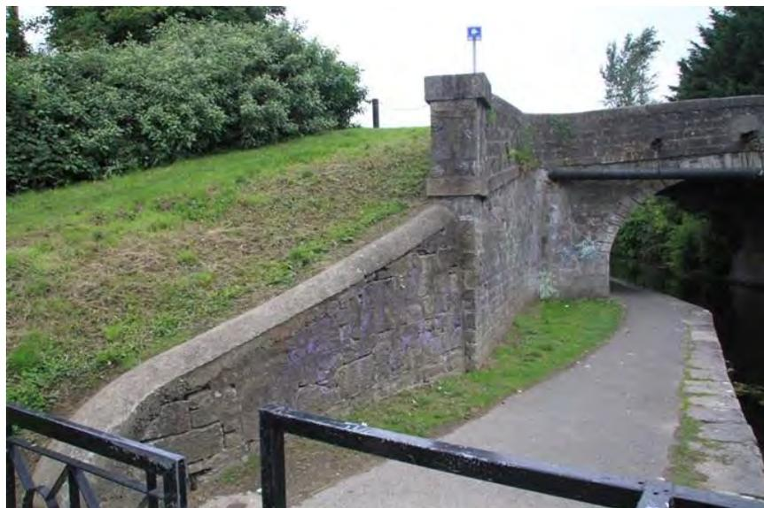
**Figure 190 Wing wall and retaining wall on southern side of canal to the east of the bridge**
