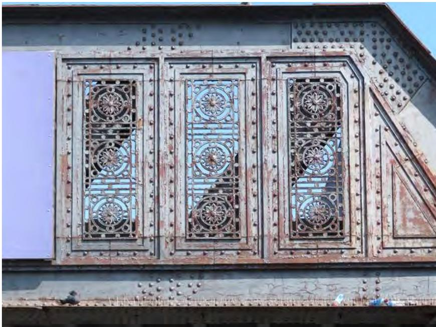
**Figure 492 Decorative cast-iron panels on bridge at Ballybough Road**
