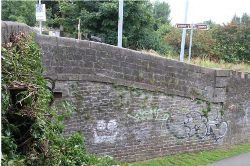
**Figure 187 Southern wing wall on western side of canal bridge**
