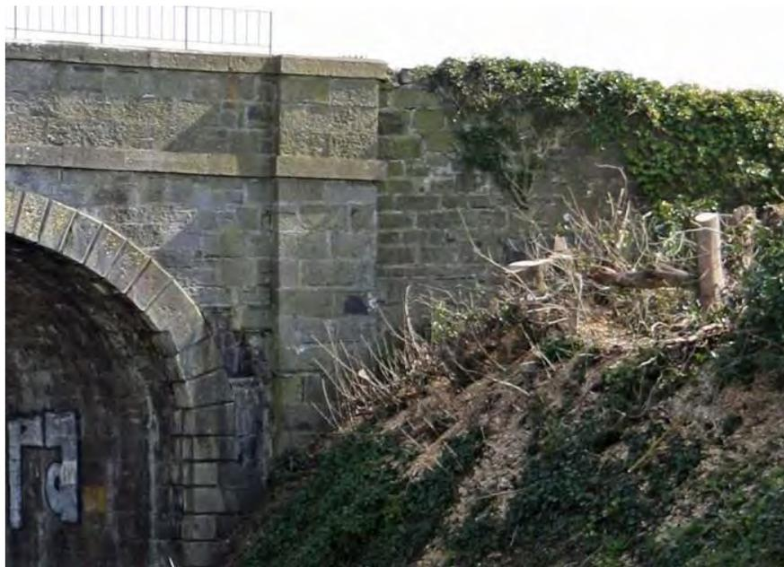
**Figure 375 Pier and wing wall on western side of railway bridge**
