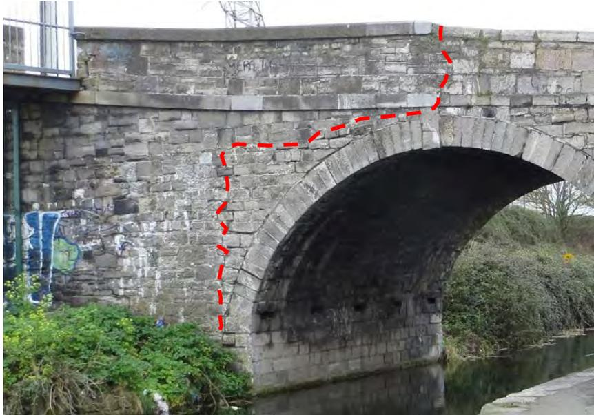
**Figure 126** Approximate line of junction between 1790s masonry and 1840s masonry
