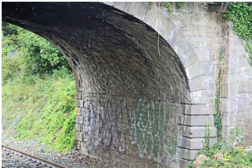
**Figure 198** Abutment and soffit of bridge on southern side
