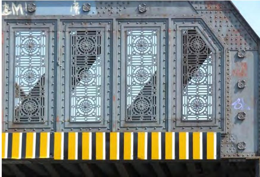
**Figure 484 Detail of cast-iron panels**
