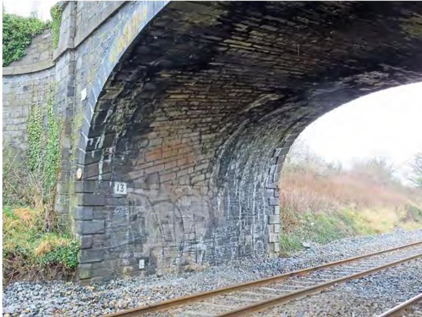
**Figure 305 Barrel of arch of railway bridge**
