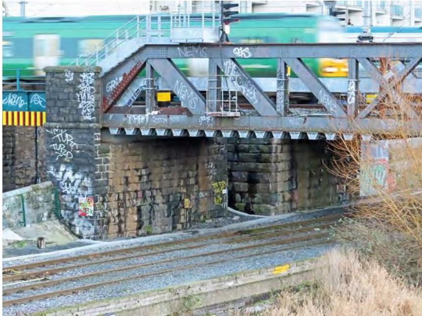
**Figure 19** Abutments of railway bridges
