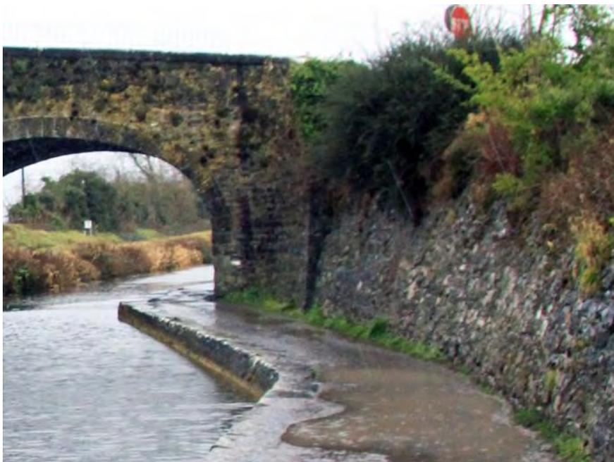
**Figure 368 Eastern wing wall and retaining wall of Canal bridge**
