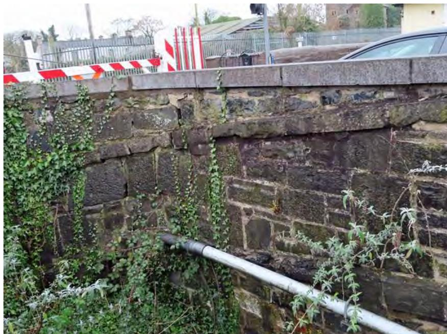
**Figure 152 Raised parapet at southern end of eastern side**
