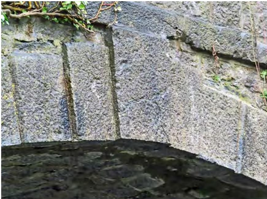
**Figure 224** Detail of keystone on eastern side of bridge
