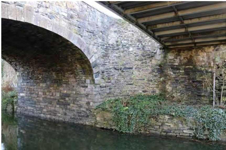
**Figure 266 Southern wing wall on western side of bridge**
