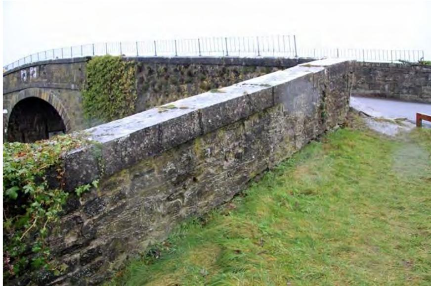
**Figure 379 Coping stones on wing wall of canal bridge**
