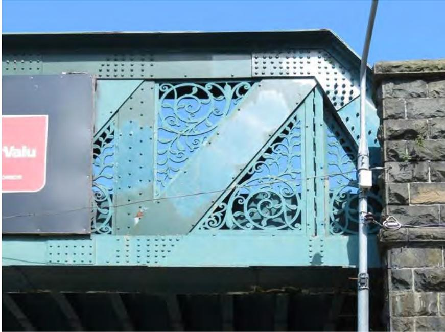
**Figure 498** Cast-iron decorative panels at eastern end of bridge
