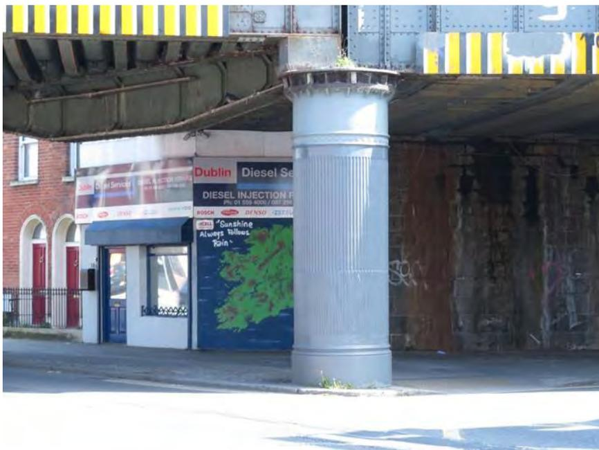
**Figure 485 Cast-iron column between the two spans**
