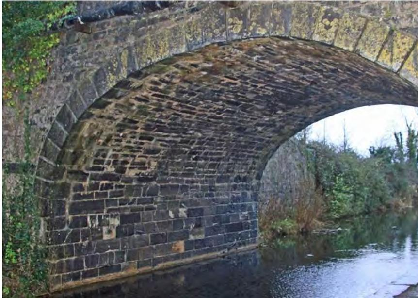
**Figure 293** View into bridge showing masonry of barrel
