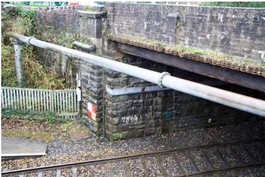
**Figure 342 Eastern abutment on northern side of bridge**
