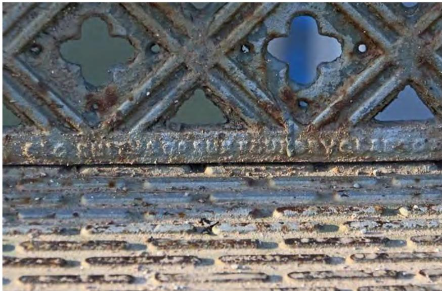
**Figure 254**      **Manufacturer's name cast into stair riser**
