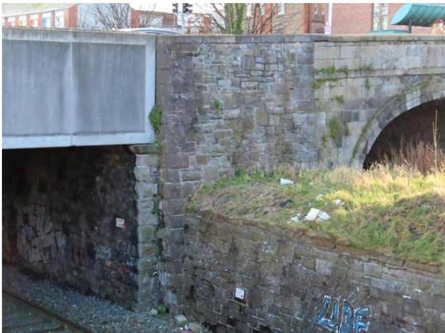
**Figure 62 Junction of abutments on western side of bridges**
