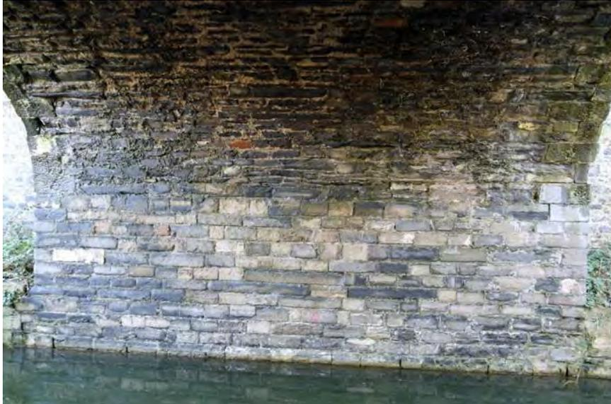
**Figure 267 Abutment and barrel of arch**
