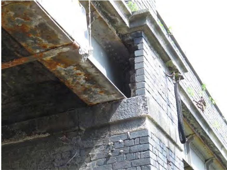
**Figure 471** Detail of side of pier adjacent to beam
