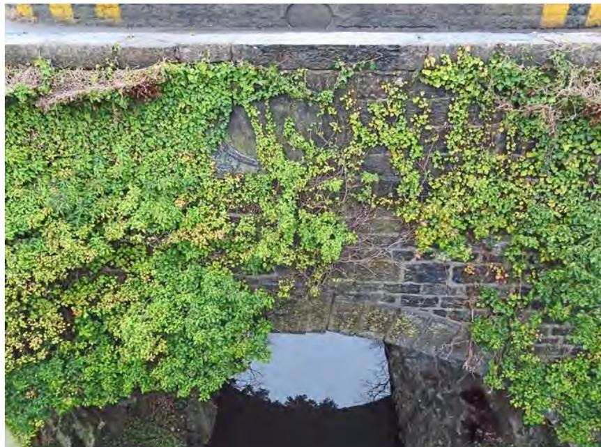
**Figure 210 Eastern keystone and parapet**
