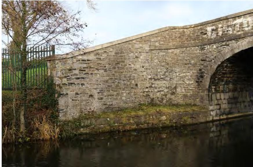
**Figure 159 Northern wing wall on western side of bridge**
