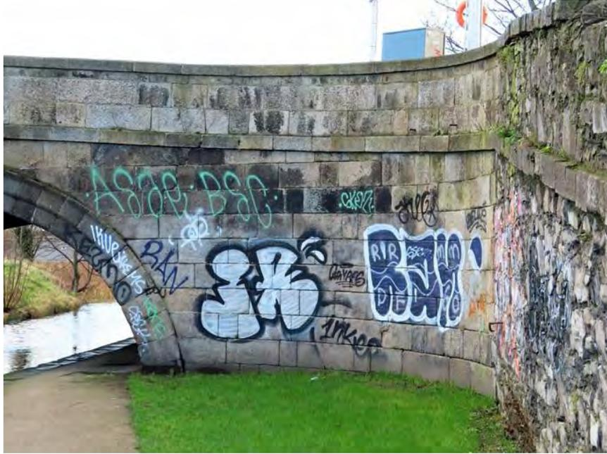
**Figure 49** Abutment and wing wall on western face of Clarke Bridge
