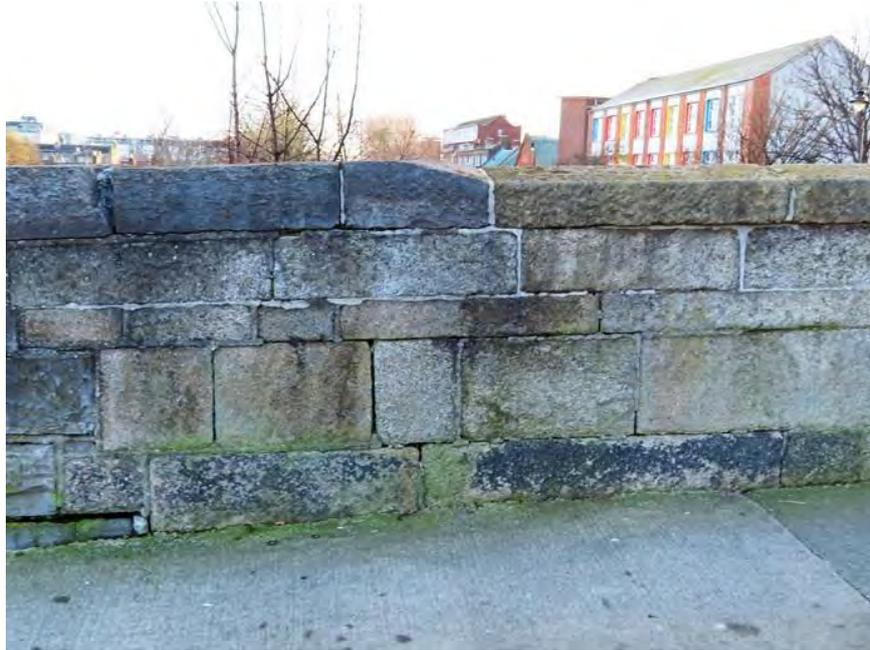
**Figure 59 Junction between parapets of canal bridge and railway bridge**
