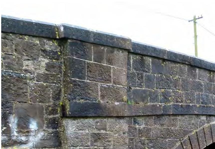
**Figure 426 Pier between railway and canal on western side, with string course and coping stones**
