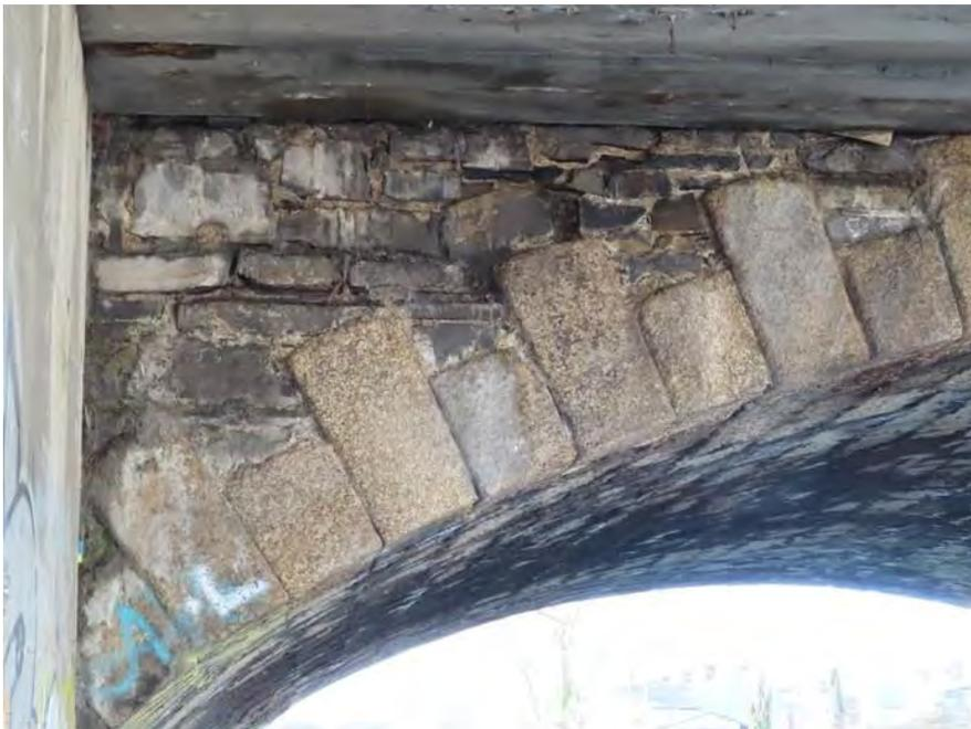
**Figure 70 Detail of voussoirs and spandrel on eastern side of Clonliffe Bridge**
