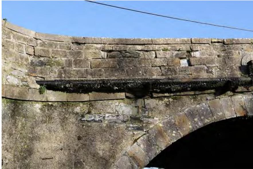
**Figure 282** Detail of spandrel and parapet
