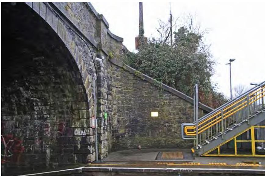
**Figure 322** Western wing wall on southern side of railway bridge
