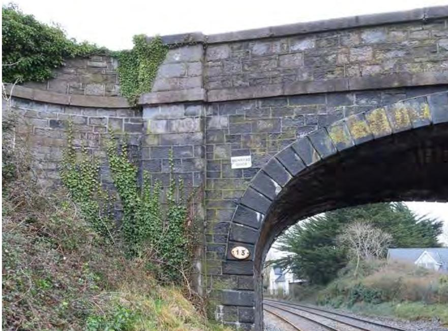
**Figure 304 Spandrel and pier on western side of bridge, northern end**
