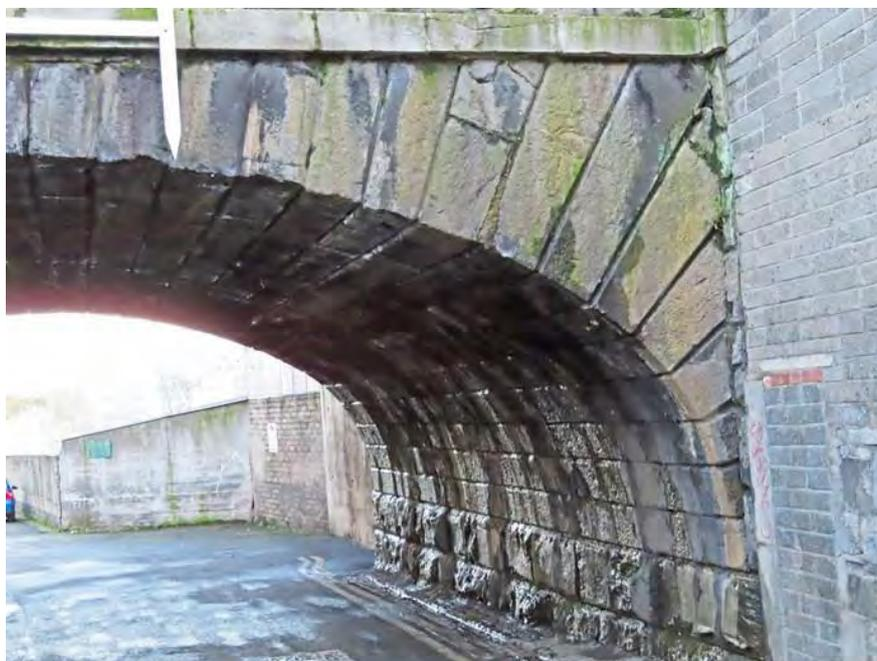
**Figure 8 Detail of spandrel and barrel of arch**
