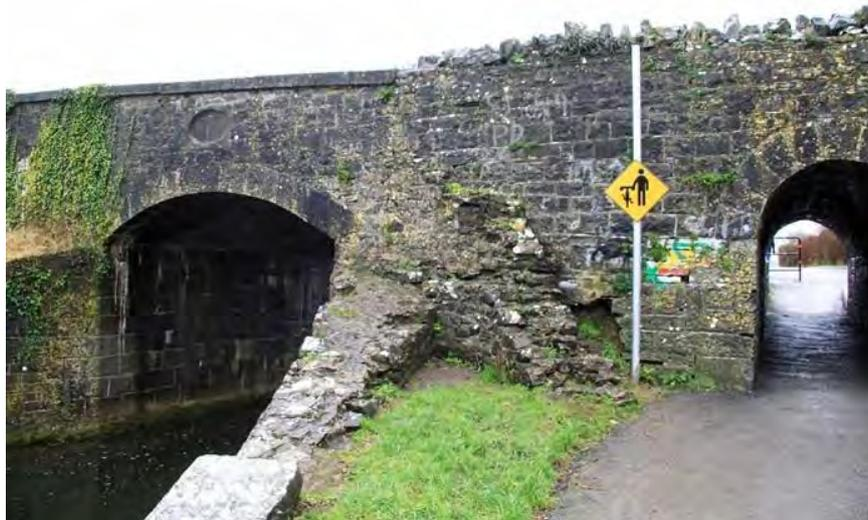
**Figure 414 Remnant of original wing wall**
