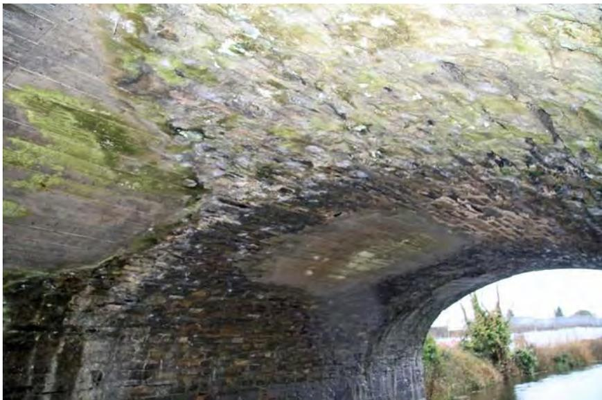
**Figure 336 Barrel of vault**
