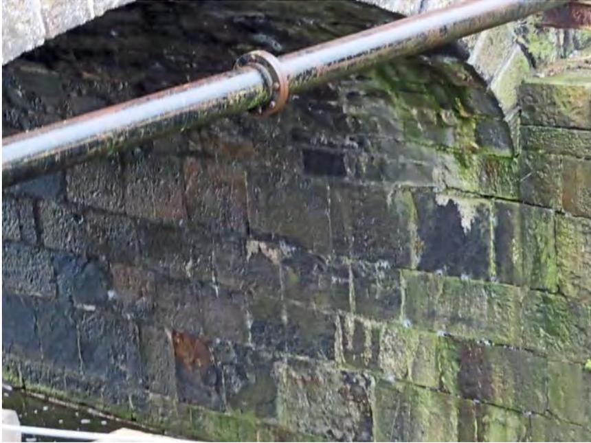
**Figure 147** Abutment and spring of arch on southern side
