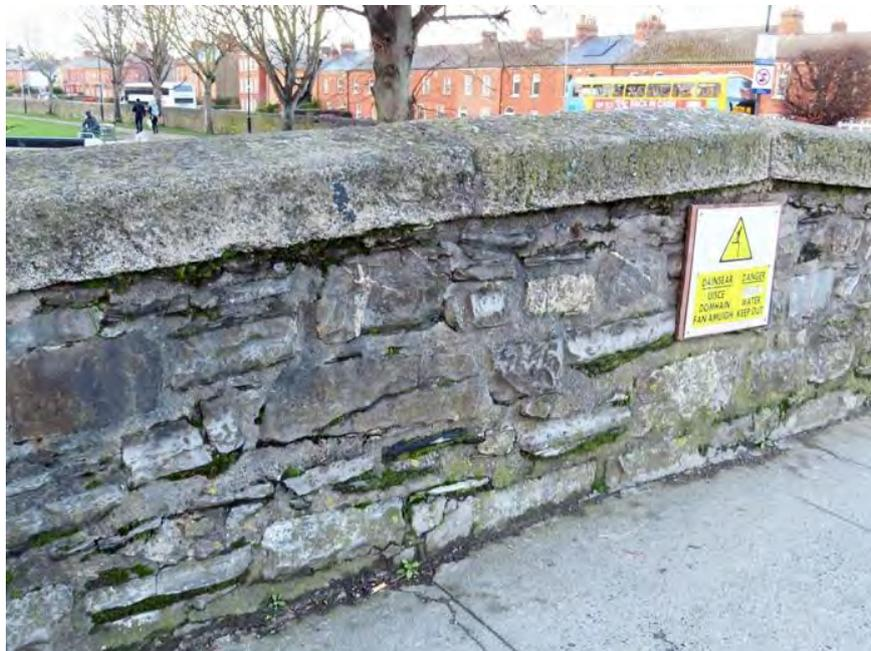
**Figure 90 Detail of parapet on western side of Binns Bridge**
