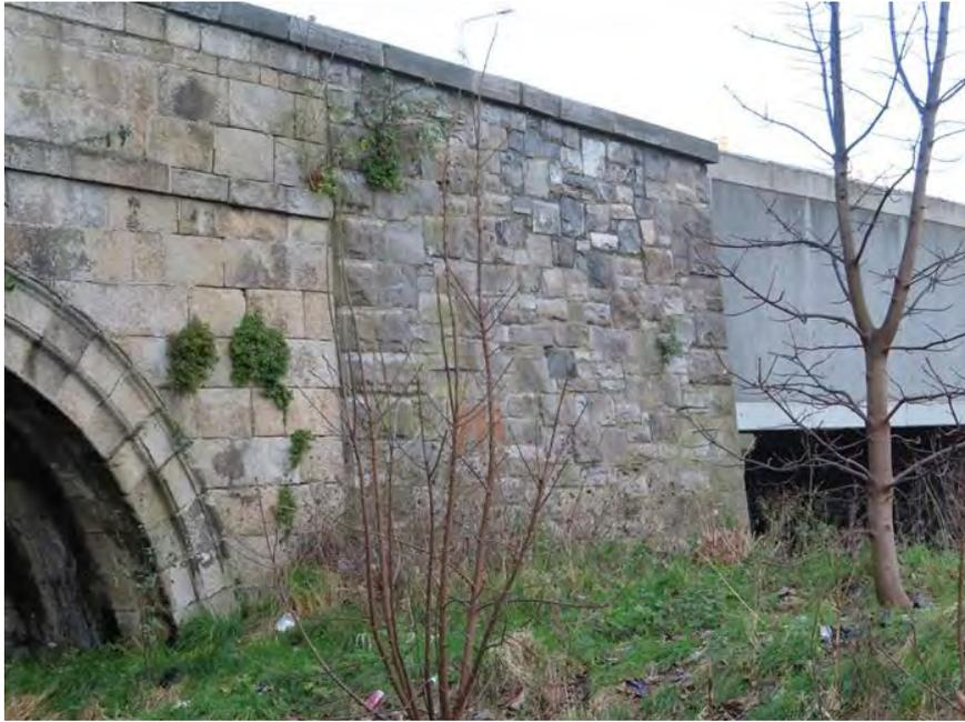
**Figure 61 Junction of abutments of canal bridge and railway bridge**
