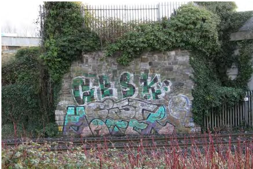
**Figure 166** Southern abutment of former railway bridge
