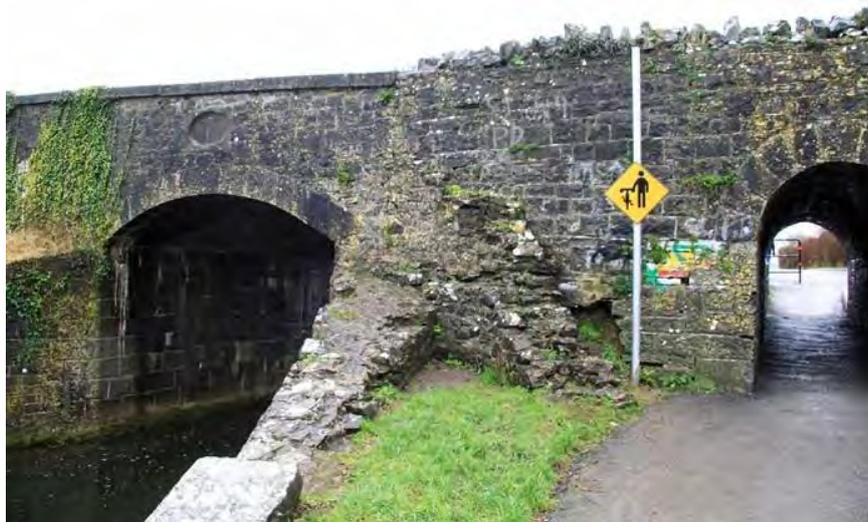
**Figure 414 Remnant of original wing wall**
