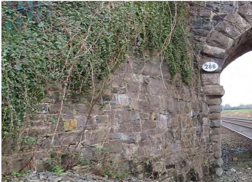
**Figure 448 Northern wing wall on western side of Barnhill Bridge**
