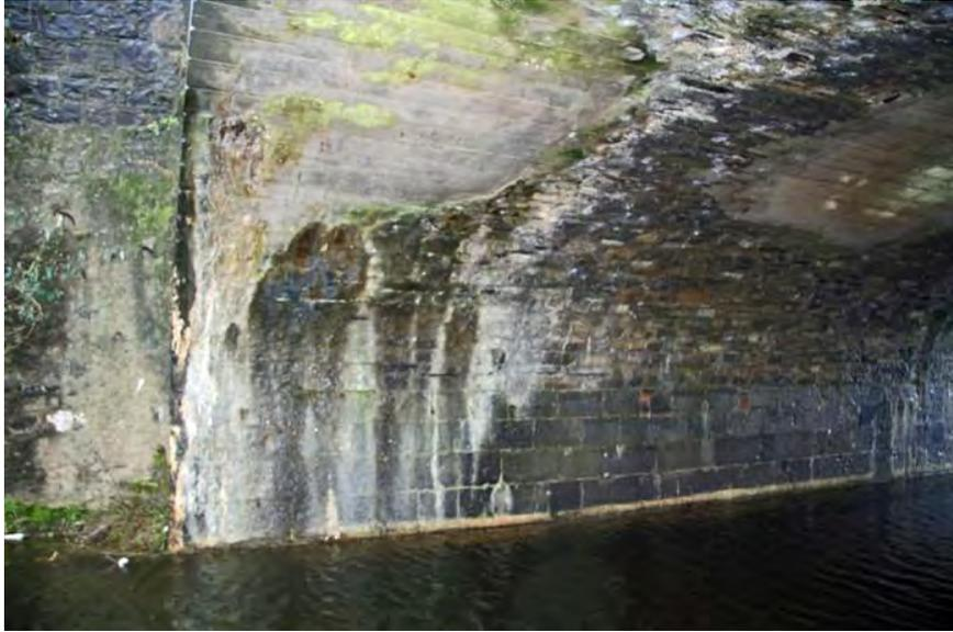
**Figure 335** Abutment and spring of vault on eastern side of bridge
