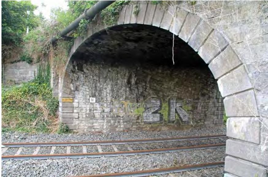
**Figure 197** Abutment and soffit of bridge on northern side
