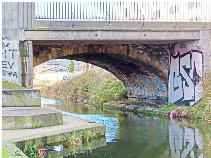
**Figure 68 Eastern elevation of Clonliffe Bridge, showing masonry arch**
