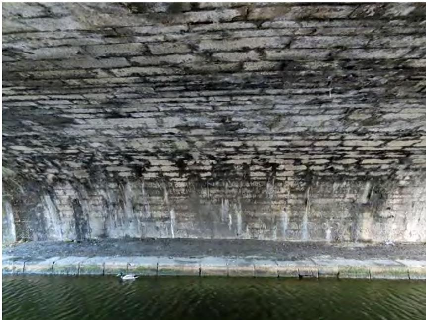
**Figure 46 Masonry in the vault of Clarke Bridge**
