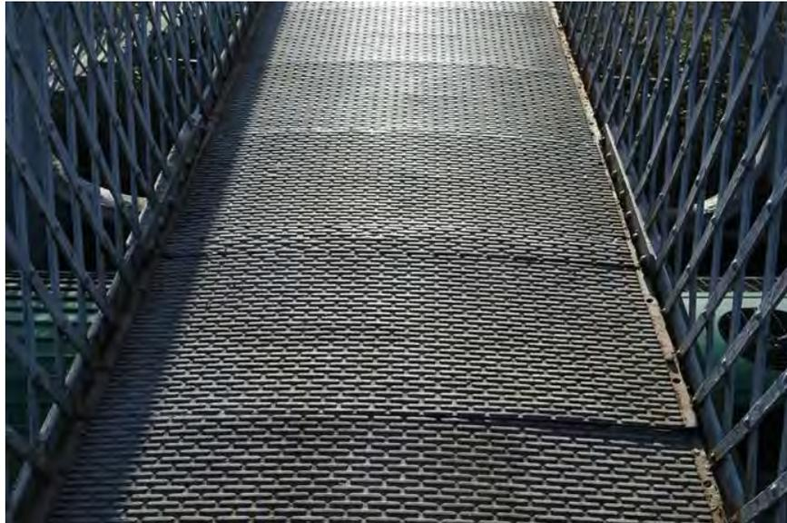
**Figure 240 Plating on bridge deck**
