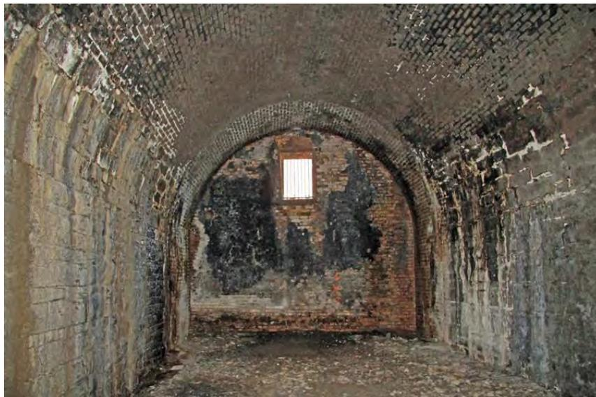
**Figure 520 Typical vault beneath Loop Line**
