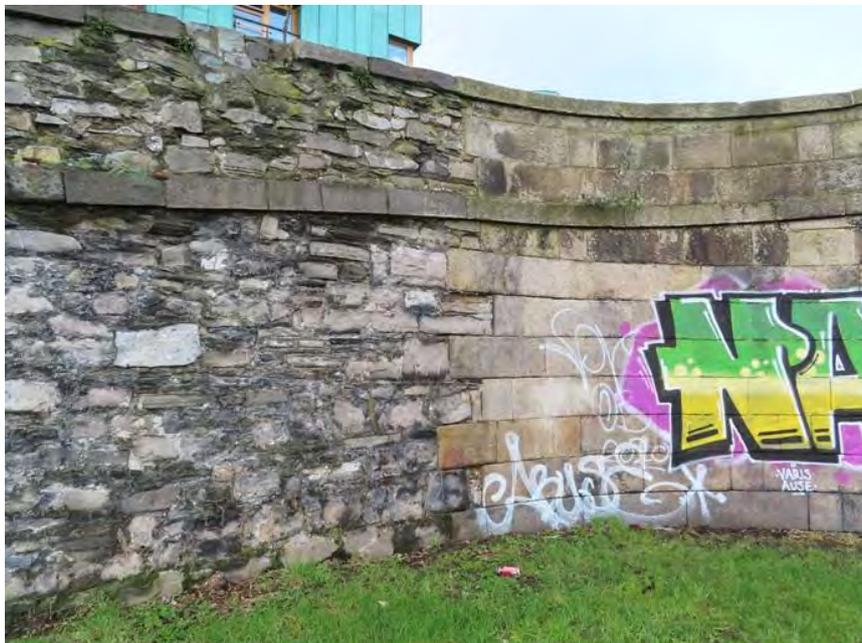
**Figure 50 Junction between wing wall and retaining wall on eastern side of bridge**
