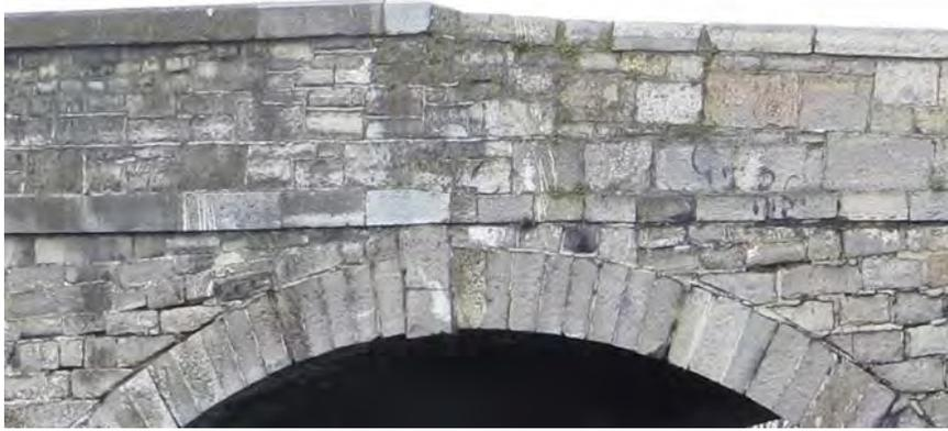
**Figure 124 Original copings and later replacements on eastern side of canal bridge**
