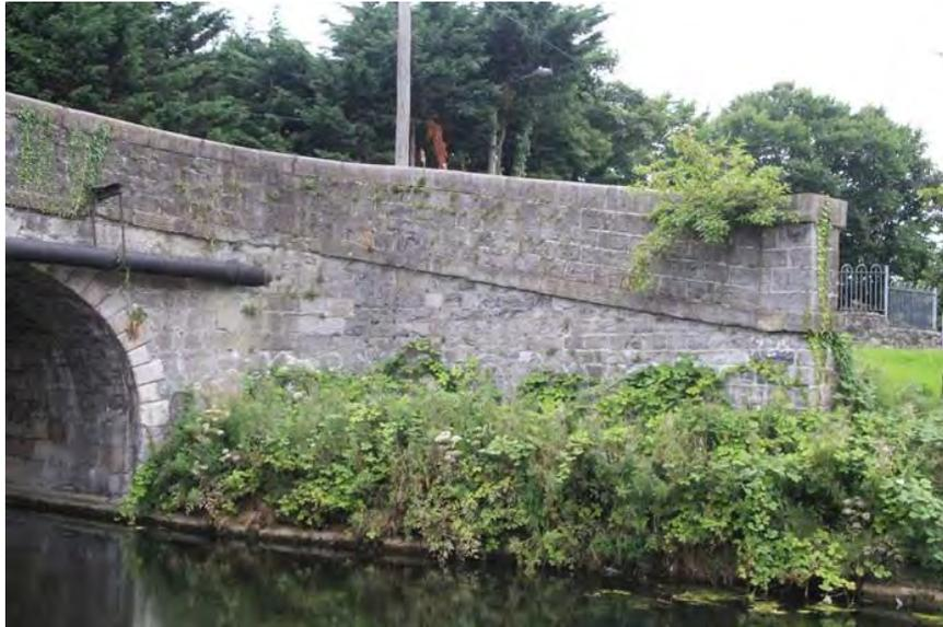
**Figure 189 Wing wall on northern side of canal to the east of the bridge**
