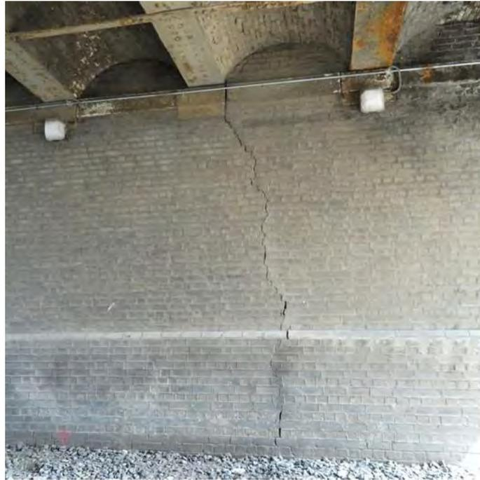
**Figure 477 Crack in sixth pier from the western end**
