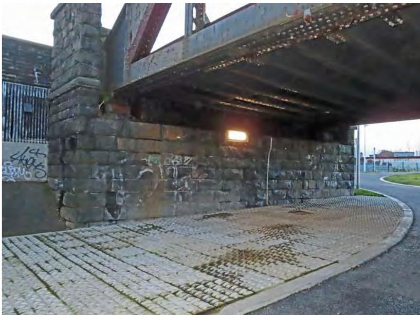
**Figure 22** Abutment at southern end of bridge
