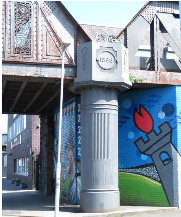
**Figure 493 Cast-iron column supporting two spans of the bridge**
