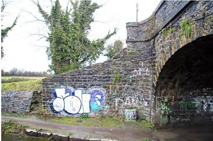
**Figure 315 Western wing wall on northern side of canal bridge**
