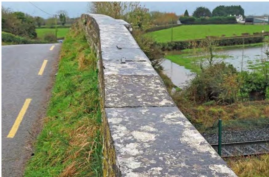
**Figure 428 Repaired section of parapet**
