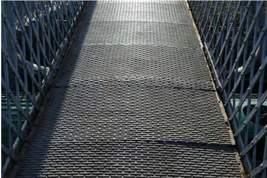
**Figure 240 Plating on bridge deck**
