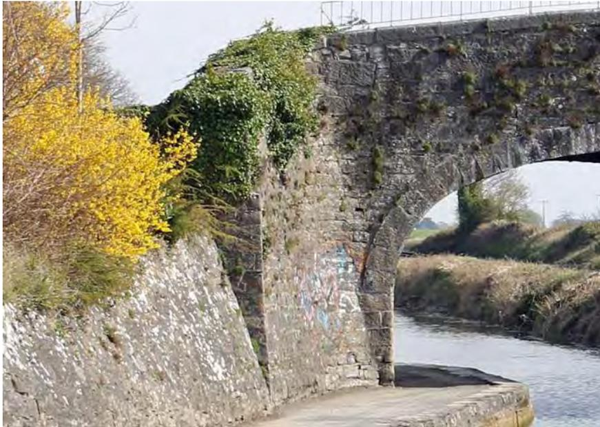
**Figure 367 Western wing wall of canal bridge**
