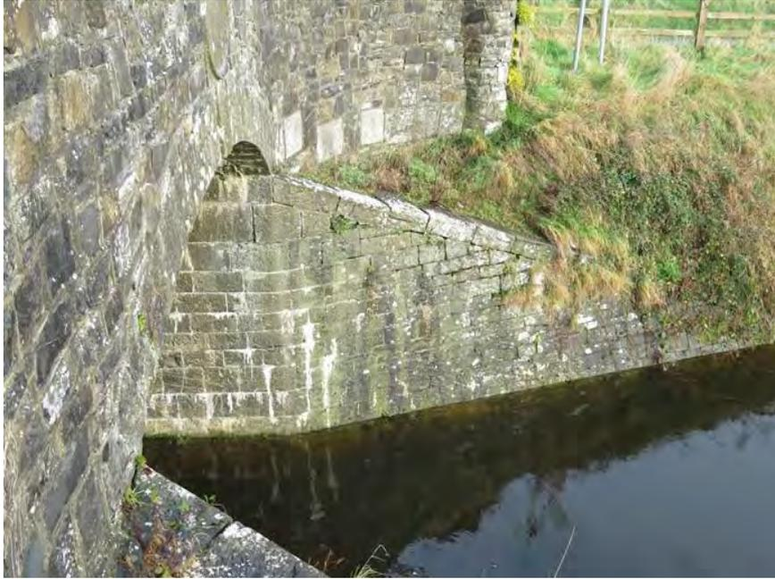
**Figure 435 Splay of abutment to east of bridge on northern side**
