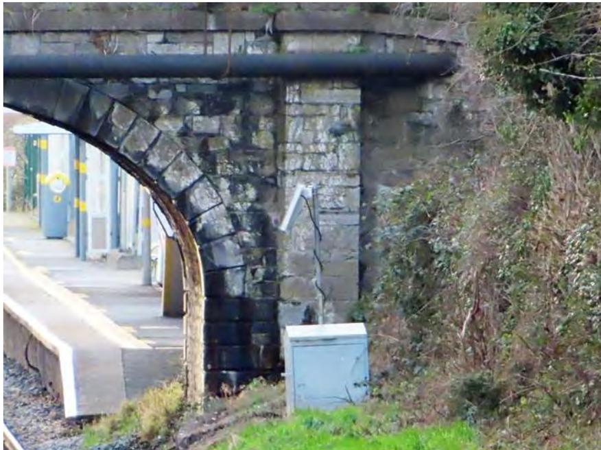
**Figure 200 Northern abutment and pier on eastern side of railway bridge**
