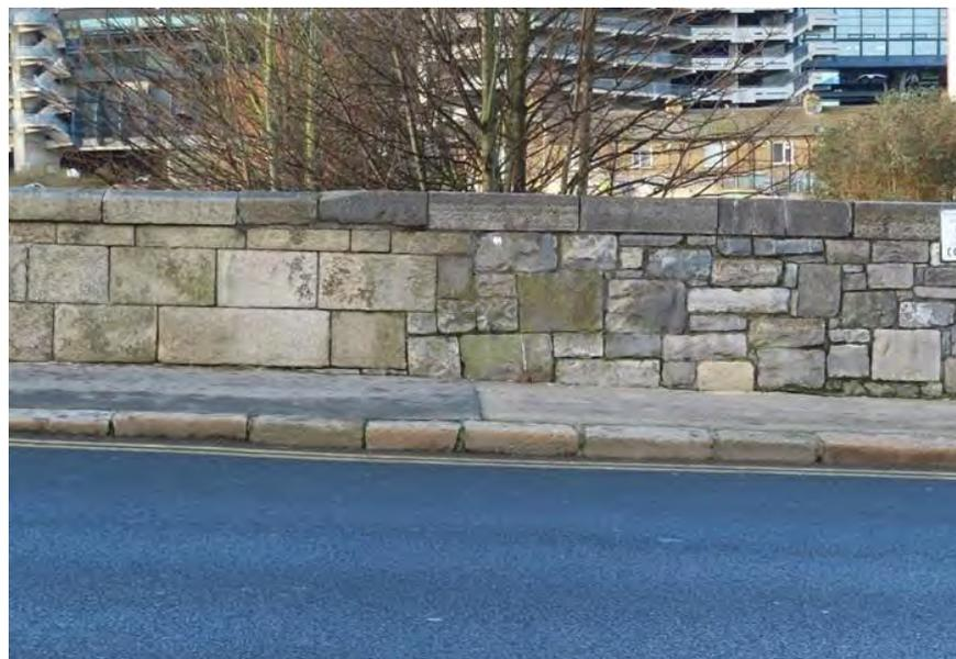
**Figure 60 Junction between parapets on western side of bridges**
