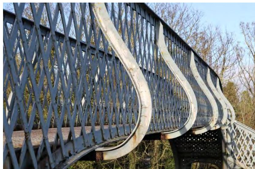
**Figure 239** Braces on outer face of parapet
