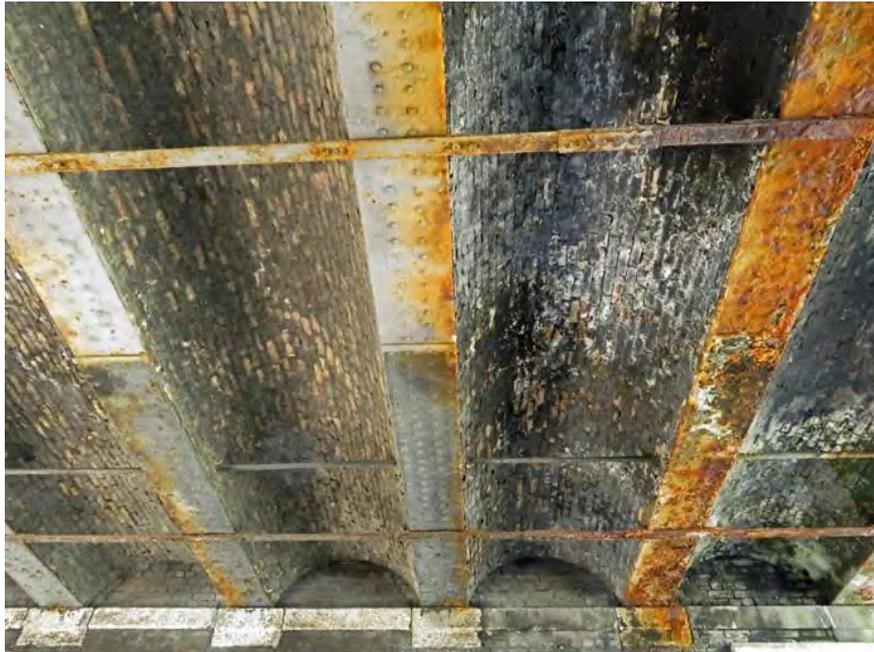
**Figure 467 Jack arches on soffit of bridge deck**
