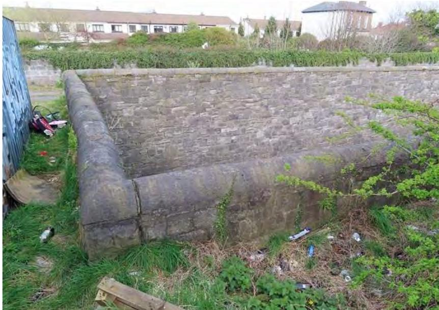
**Figure 111 Detail of parapets at accommodation bridge**
