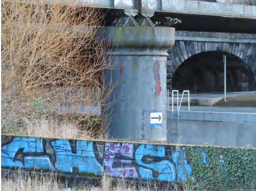
**Figure 23** Detail of cast-iron pier
