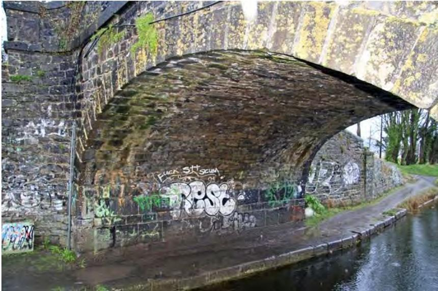
**Figure 313** Vault of canal bridge
