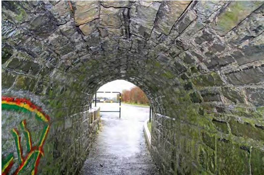
**Figure 413 Barrel of vault of towpath arch**
