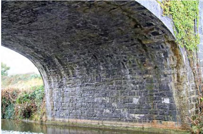
**Figure 369 Abutment and barrel of canal bridge**
