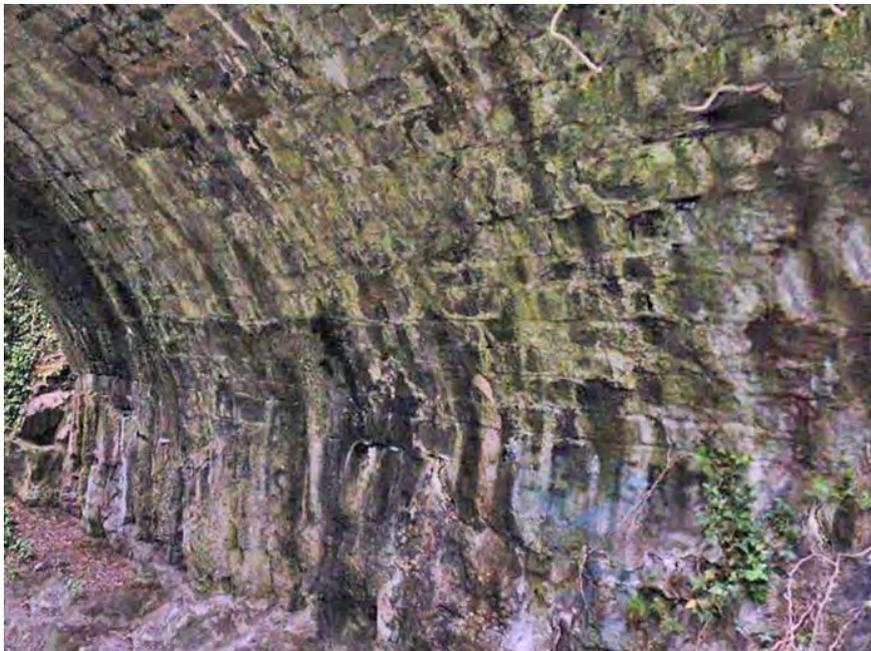
**Figure 212 Detail of abutment and vault beneath bridge**
