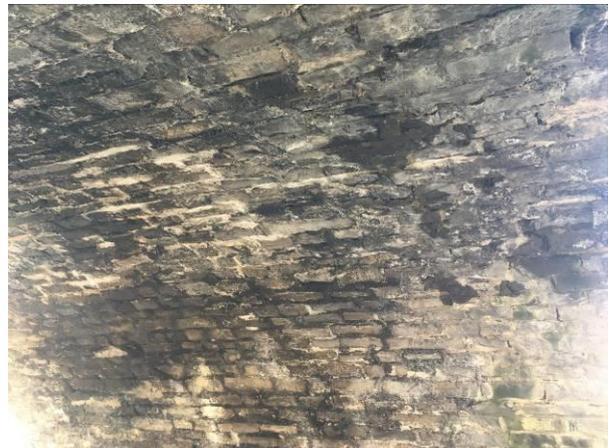
**Figure 19** – Condition of canal arch stonework.
