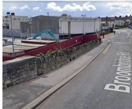
**Figure 9** – South east parapet end and historic random rubble limestone wall.
