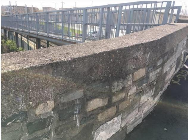
Figure 23 – Poor condition of pointing & concrete copings.
