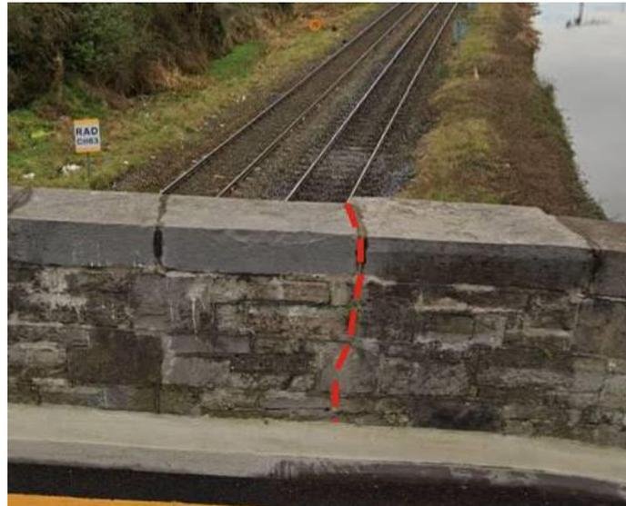
**Figure 28** – Image of parapet internally with line highlighting where the junction with the new concrete parapet will be.
