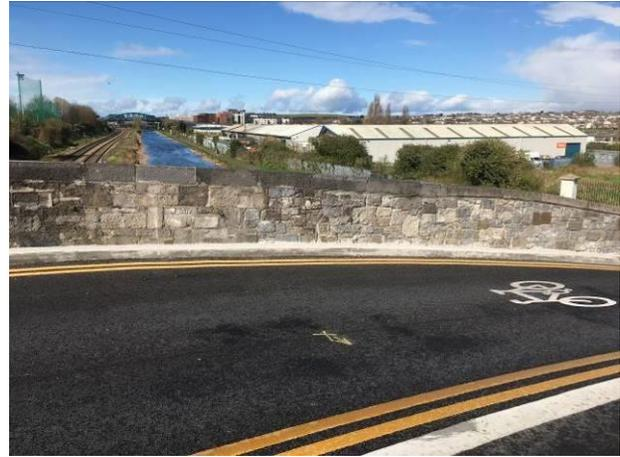
**Figure 14** – West parapet showing section of parapet rebuilt.
