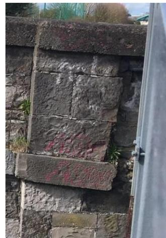
Figure 24 – Pier stone damaged.
