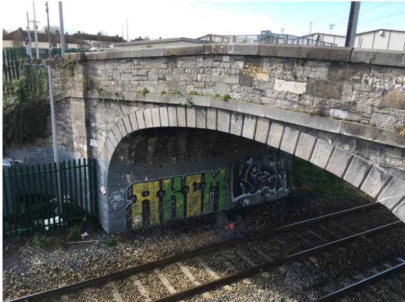
**Figure 4** – Railway arch showing voussoirs of arch ring, string course, engaged pier and a wing wall curving away to the east (left hand side).
