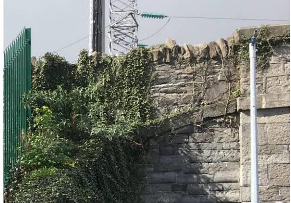
Figure 22 – Original copings visible to south east wing wall.
