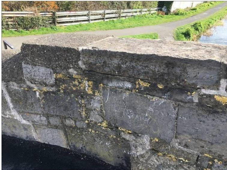
**Figure 30** – Existing parapet requires repair and conservation works.
