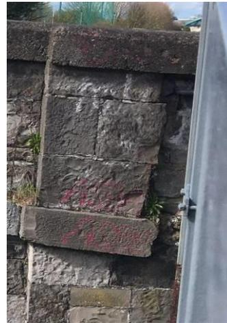
Figure 24 – Pier stone damaged.
