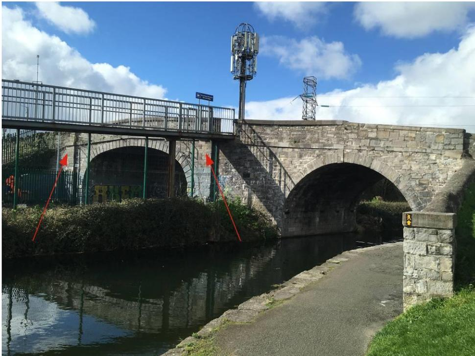
**Figure 27** – Existing bridge with engaged piers highlighted.
