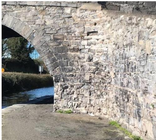
**Figure 18** – Weathered facing stone visible, especially below the spring of the arch.
