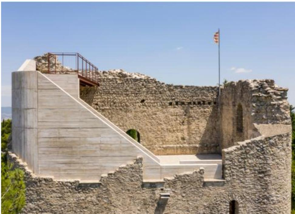
**Figure 26** – Example of a new board marked concrete insertion in an existing stone structure.
