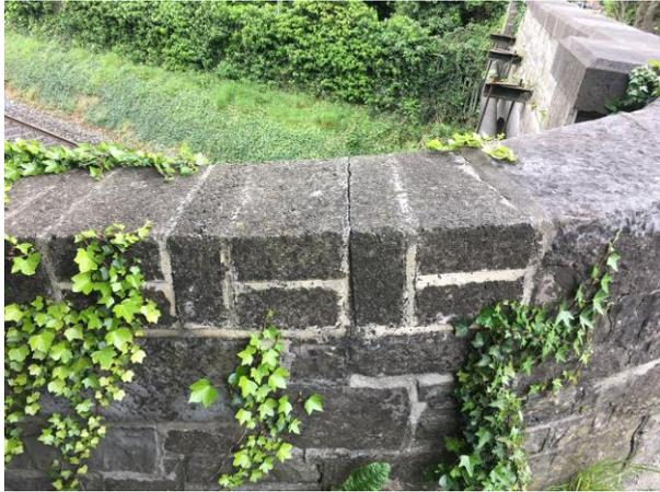
**Figure 18** – North east parapet repaired in blockwork with cracks visible.
