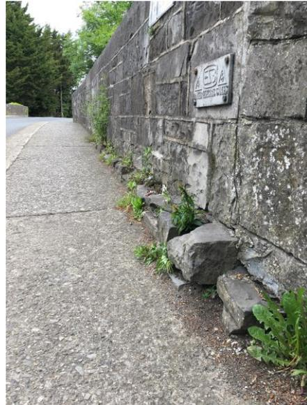
**Figure 23** – Stonework at base of wall requiring pointing.
