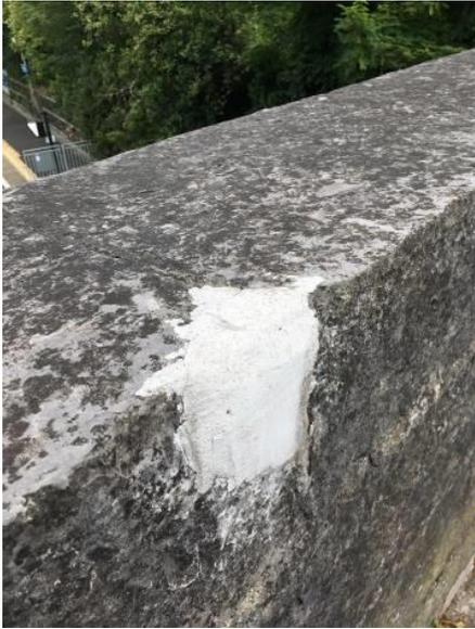
**Figure 22** – Poor mortar repairs to copings.
