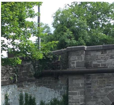
Figure 16 – Poorly rebuilt stonework around service pipe on north west side.
