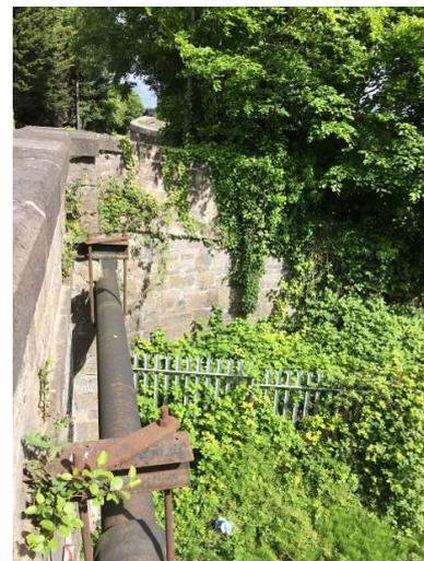
**Figure 6** – North east wing wall with substantial block repairs.
