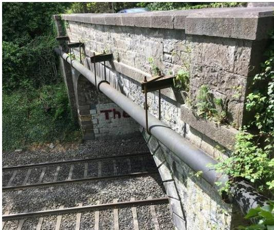
**Figure 9** – Canal spandrel with squared limestone.
