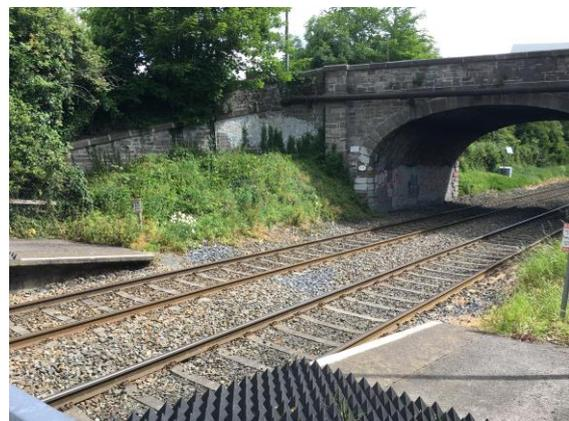
Figure 17 – Vegetation and paint on north west wing wall and paint under bridge.
