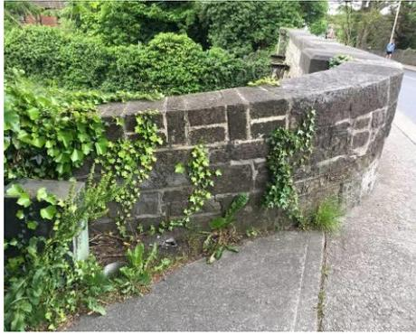
**Figure 7** – North east parapet with modern blockwork.
