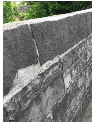
**Figure 21** – Joint below coping stones broken.
