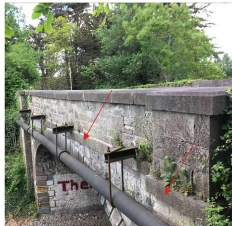
Figure 25 – East Elevation with string course highlighted.
