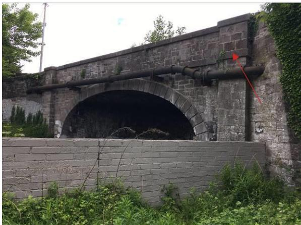
**Figure 24** – West elevation with string course highlighted.
