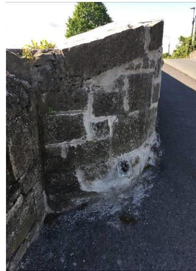
**Figure 26** – Recent repairs to north east corner.
