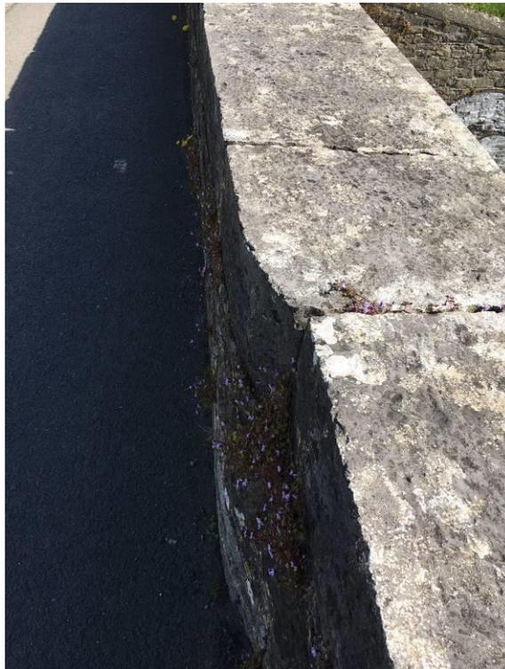
**Figure 14** – View taken looking down on coping stones on Cope Bridge's north east parapet, showing the depth of the wall top extending into the bridge.
