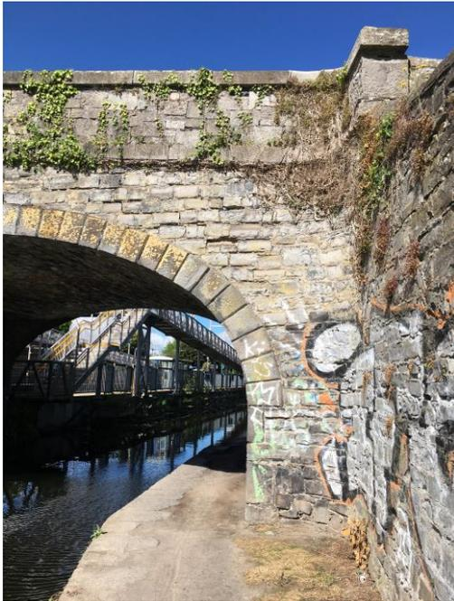
Figure 2 – East elevation showing arch ring.
