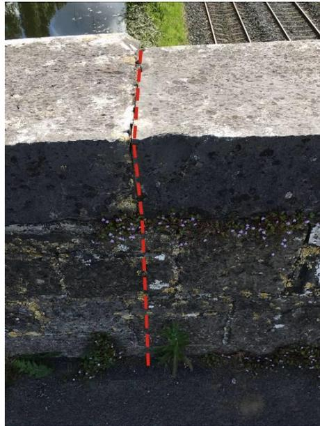
**Figure 31** - Image of parapet internally with line highlighting where the junction with the new concrete parapet will be.
