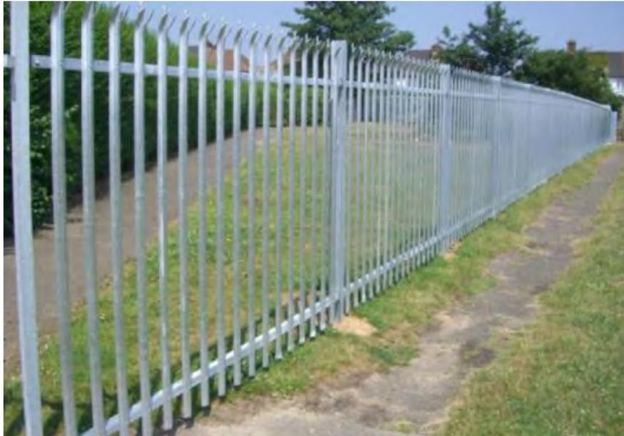
**Figure 4-27 Palisade fence example**
