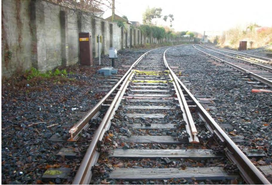
**Figure 4-211 Current siding trap point. Source IAMS**
