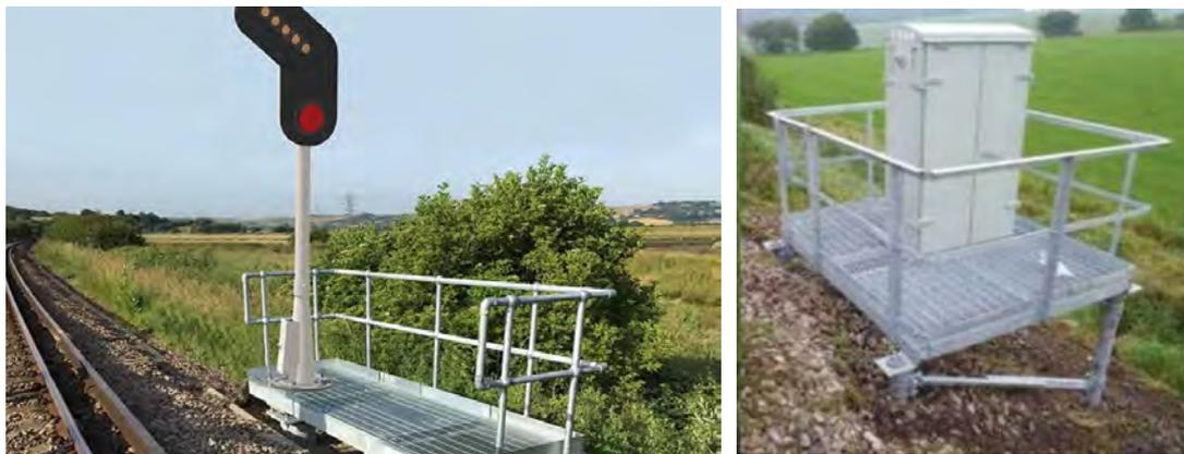
**Figure 4-13 Signal and LOC installed on a platform**
