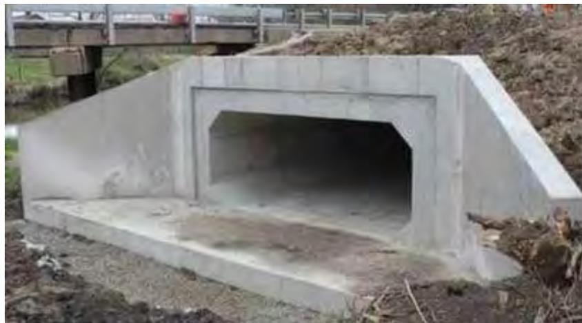
**Figure 4-259 Indicative flood relief culvert**
