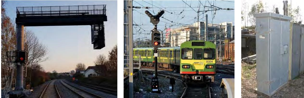
**Figure 4-10 Sample DART+ West signalling infrastructure (cantilever, signal, LOC, from left to right)**
