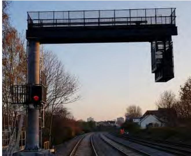
**Figure 4-12 Sample cantilever signal gantry**
