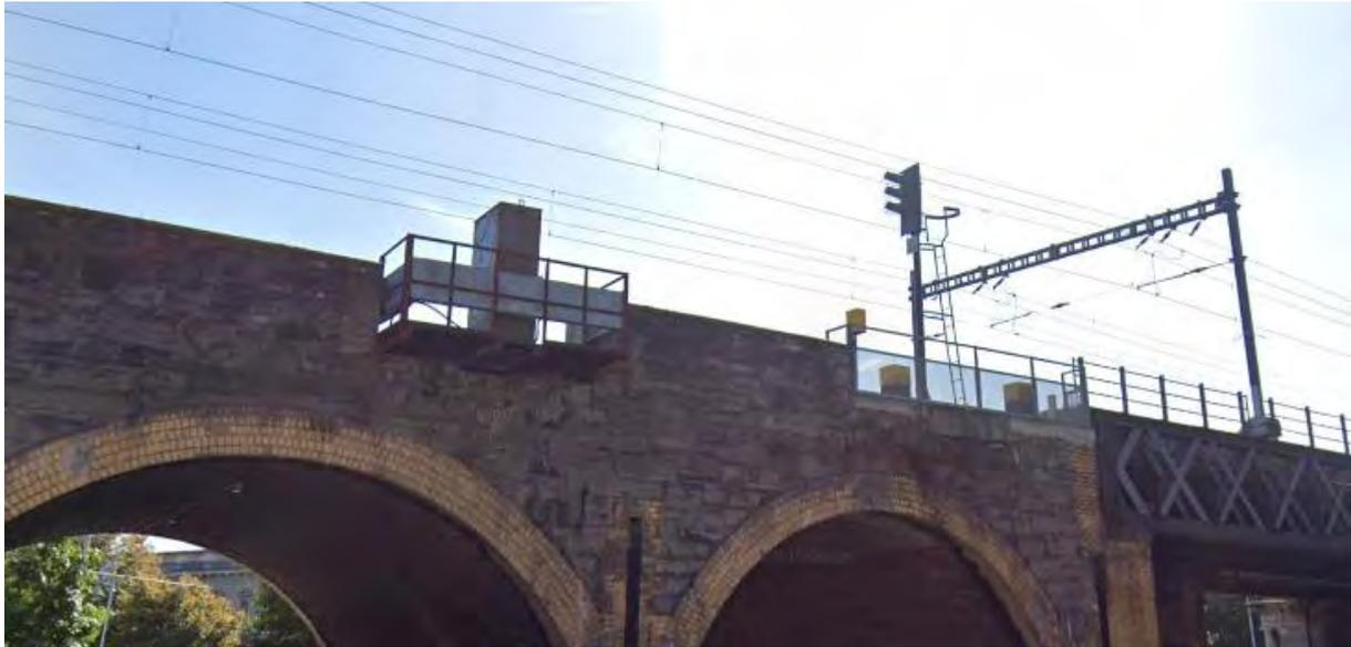
**Figure 4-14 Signalling equipment installed on a bridge platform.**
