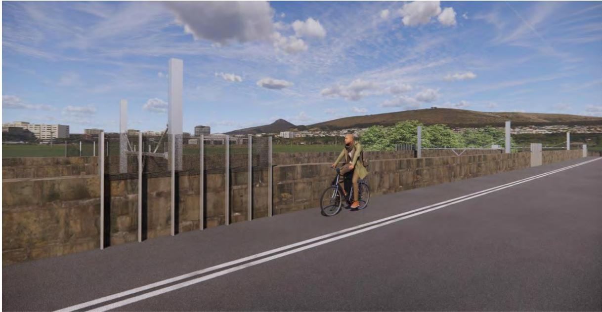
**Figure 4-54 Wall heightening adjacent to catenary posts**
