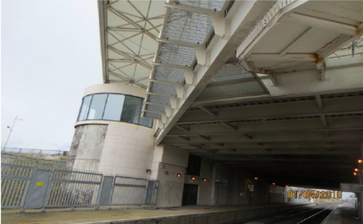
Figure 4-35 Park West & Cherry Orchard Station - View of the Maintenance Platform
