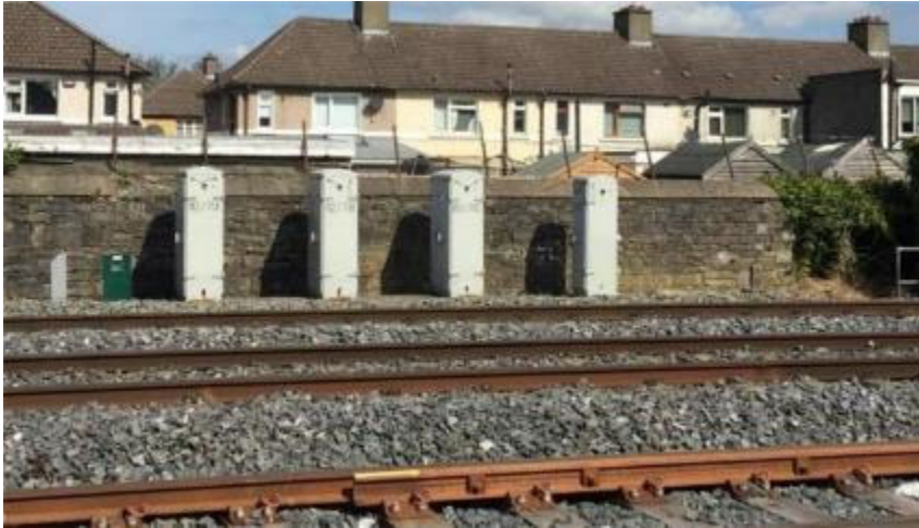
Figure 4-21 Typical Location Case
