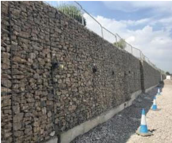
Figure 4-4 Example of Gabion Basket Wall
