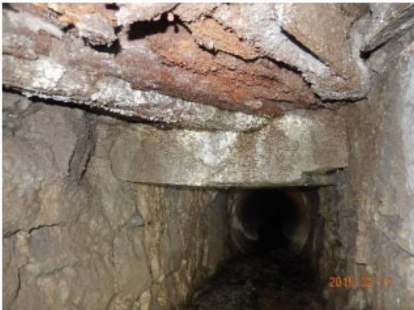
Figure 4-133 Existing Pond Overflow Pipe and Inspection Chamber
