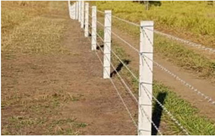
Figure 4-8 Post and Wire Fence
