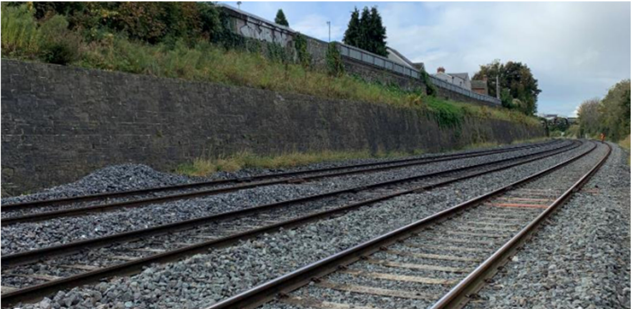
Figure 4-78 Masonry Retaining Wall on the South Side of the Rail Corridor
