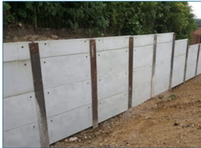
Figure 4-5 Example of King Post Retaining Wall
