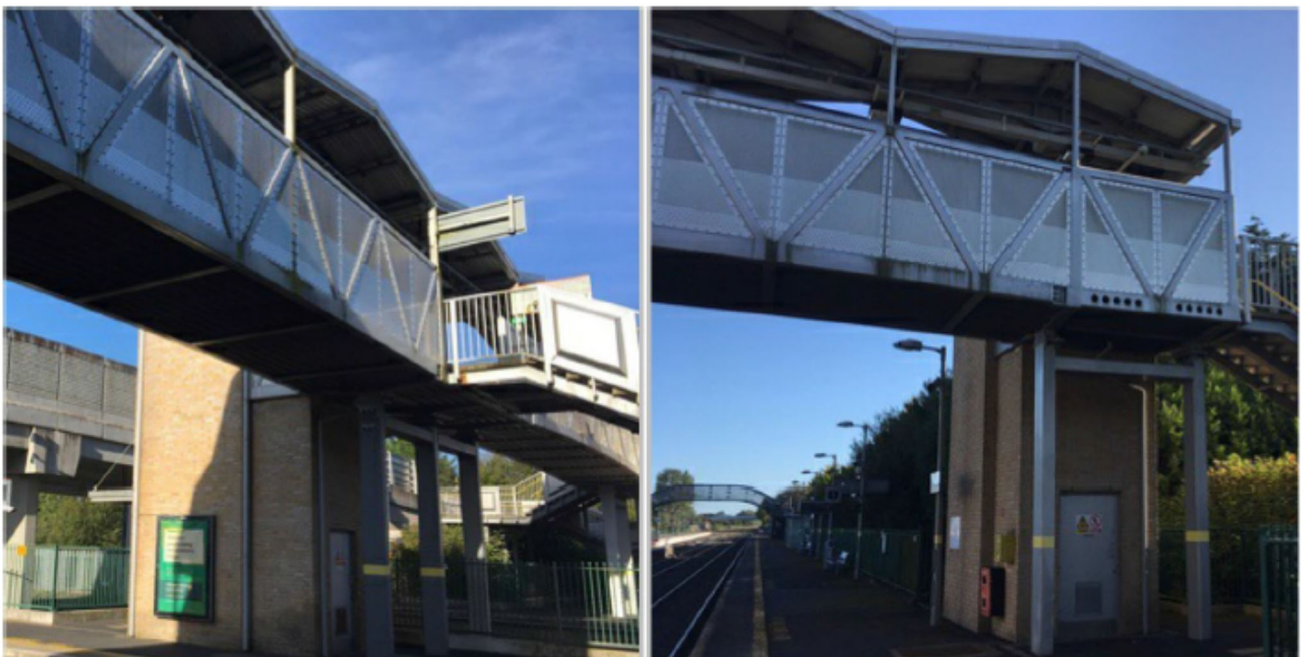
Figure 4-34 Hazelhatch Footbridge (OBC24A) External Views
