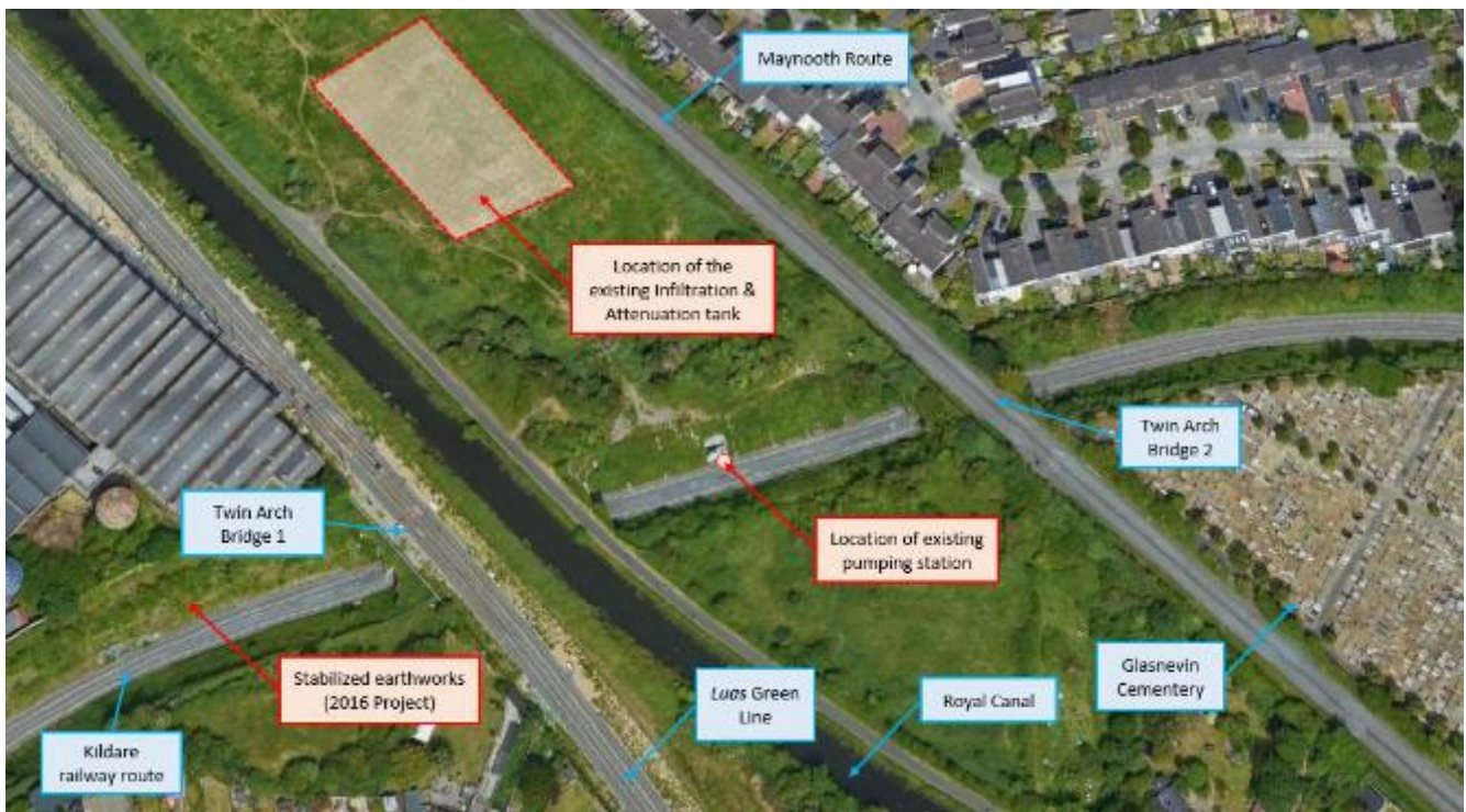
Figure 4-138 Location of the Twin Arch Bridges (OBO8 & OBO9) and the Stabilization Works
