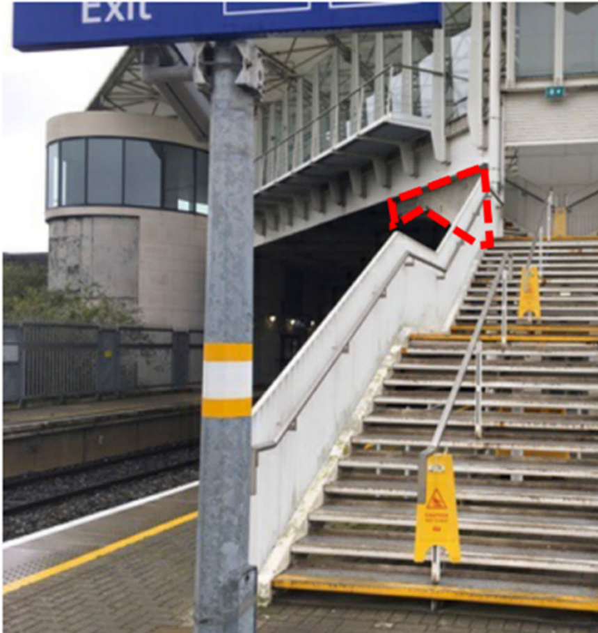
Figure 4-39 External View of the Central Stair, Park West & Cherry Orchard Station (Areas to Protect are Marked in Red)
