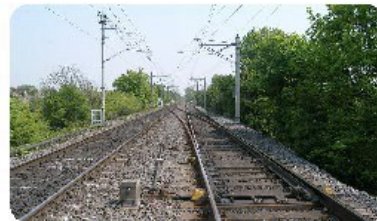
View of typical section of twin track electrified rail line
