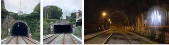
Portals to the Phoenix Park Tunnel and View of Inside Tunnel
