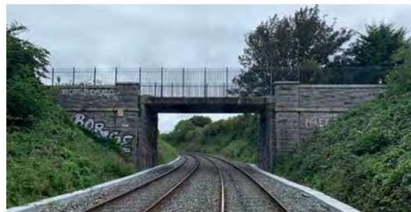
View from the east, of Glasnevin Cemetery Road Bridge
