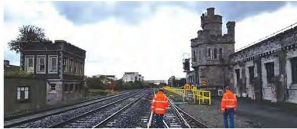
View of Locomotive Shed and Turret (right) and Signal Box (left)
