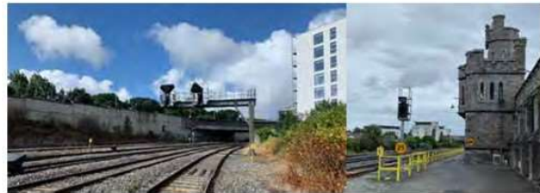
Typical Signalling Infrastructure
