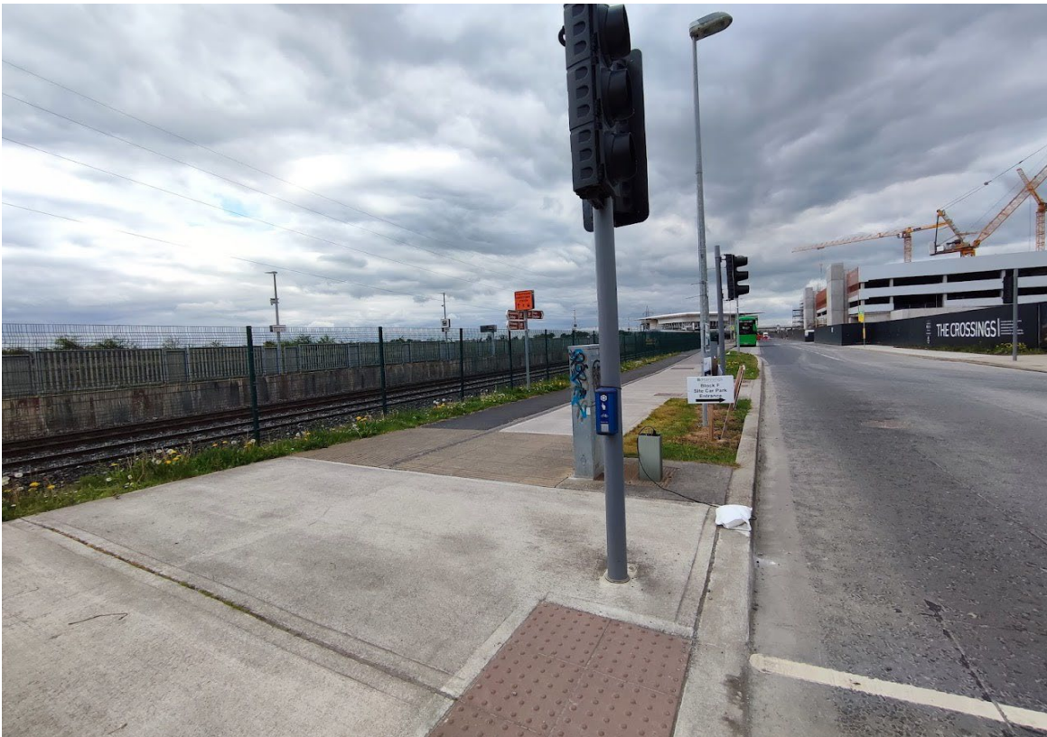
Figure A14-3 Adamstown 10m Installation
