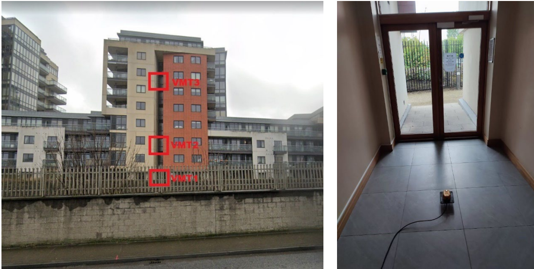
Figure A14-4 Kilmainham Square Installation
