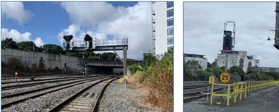
Figure 2-2 Typical Existing Signalling Infrastructure
