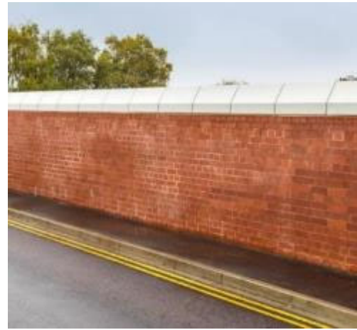
Figure 4-33 GRP Parapet Extension
