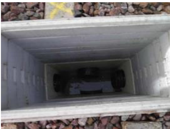
Figure 4-140 Proposed Catch-Pit with Modular Inspection Chamber
