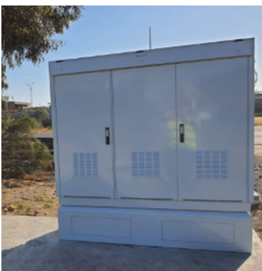
Figure 4-20 Typical Object Controller Cabinet (OBJ)
