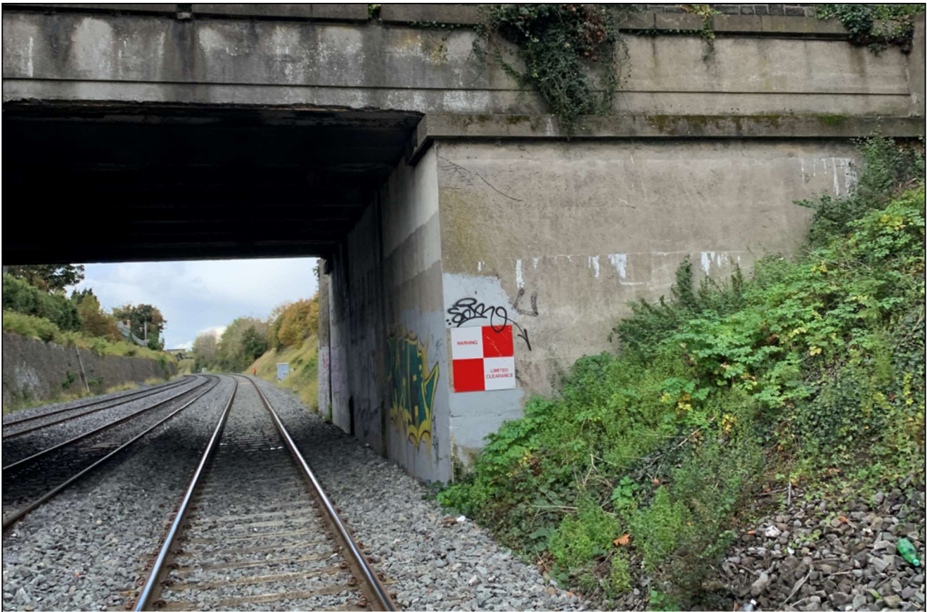
Figure 2-7 Nearest rail from northern bridge abutment wall is 1.3m - Facing West
