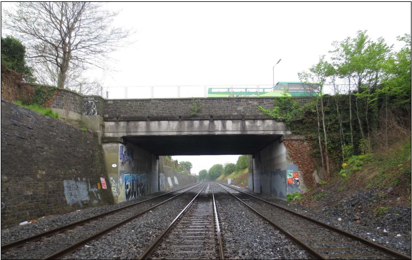
Figure 2-2 Memorial Road Bridge (OBC3) - East Elevation
