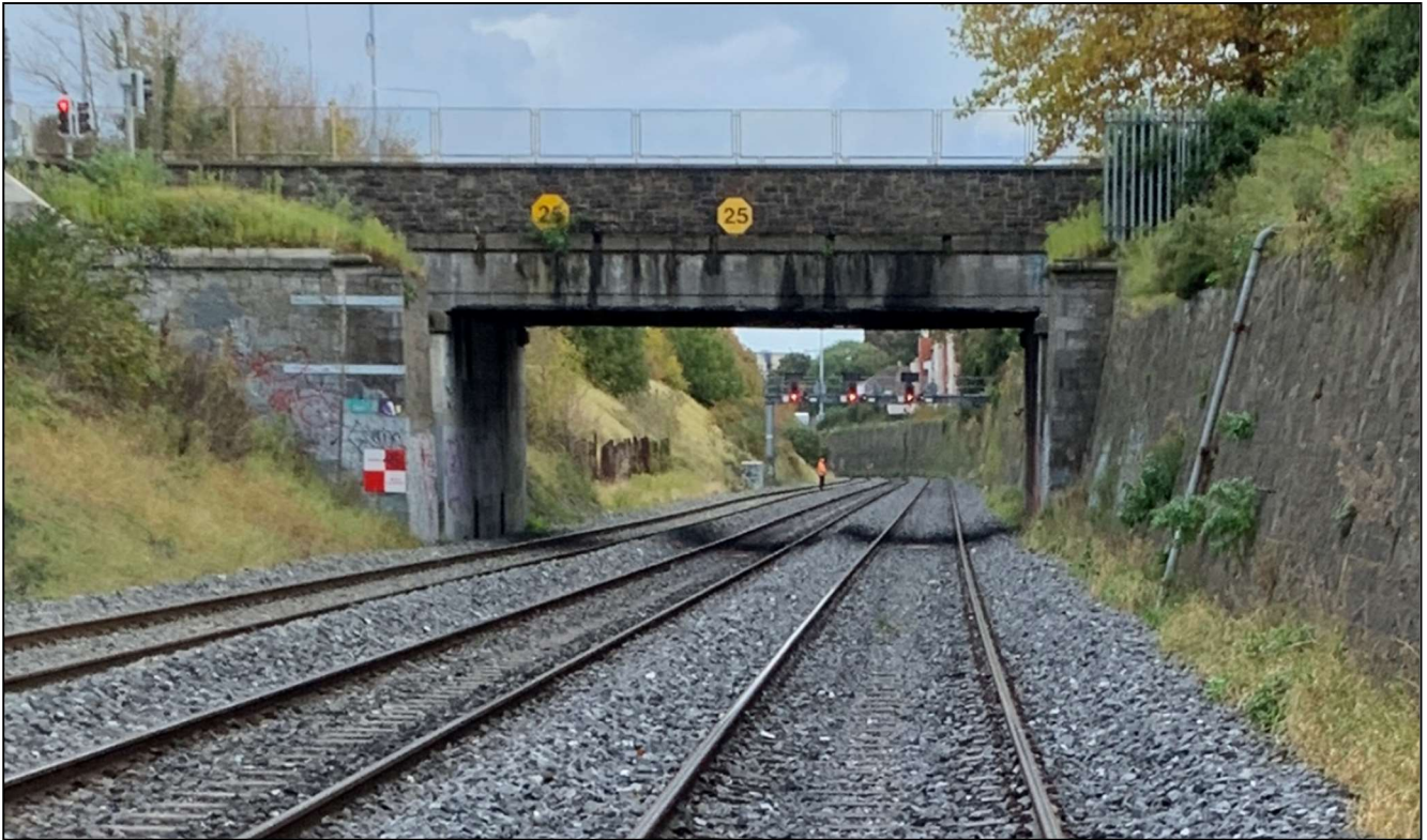
Figure 2-6 Nearest rail from southern bridge abutment wall is 1.7m - Facing East
