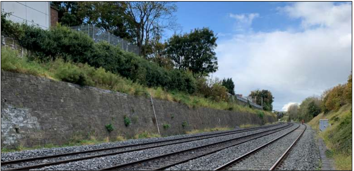
Figure 2-3 Masonry Retaining Wall south-west side of Memorial Road Bridge (OBC3)
