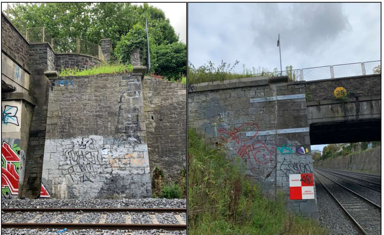
Figure 2-4 Disused masonry abutments to the west of Memorial Road Bridge (OBC3)
