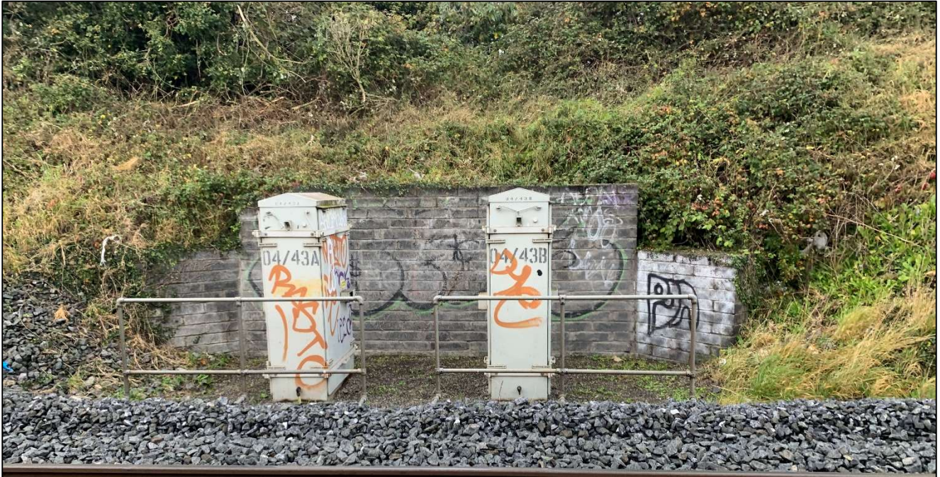
Figure 2-3 Masonry retaining wall
