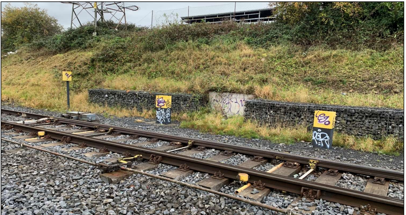
Figure 2-9 Gabion retaining wall along southern edge of cess.
