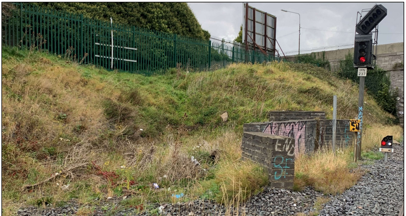
Figure 2-7 Blockwork headwall east of Le Fanu Road Bridge (OBC7)
