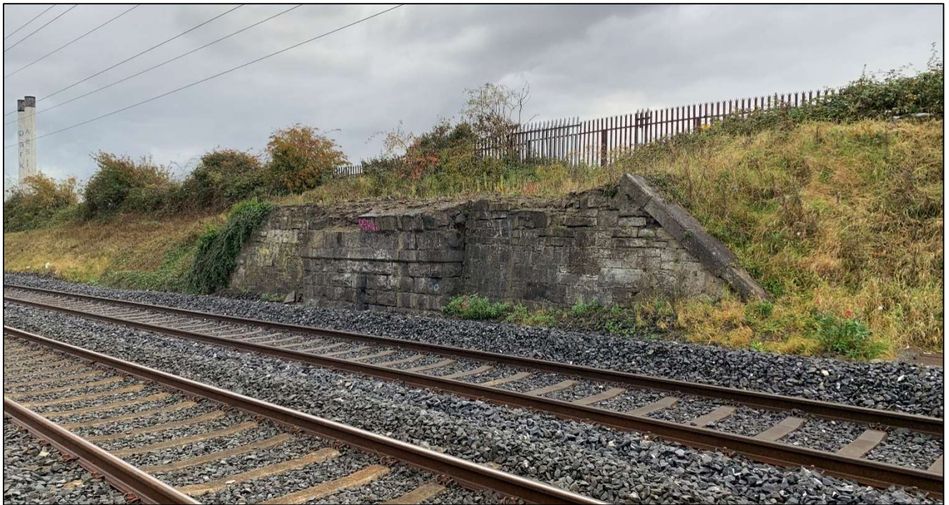
Figure 2-11 Masonry retaining wall (possibly a partially defunct bridge abutment)
