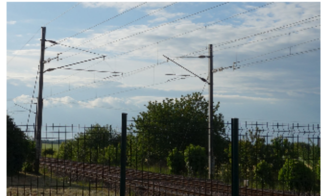
Figure 7. Example of 1x25kV OHLE (Niort-La Rochelle, France)
