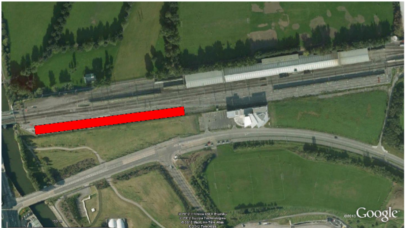
Figure 17. Fairview Depot Extension
