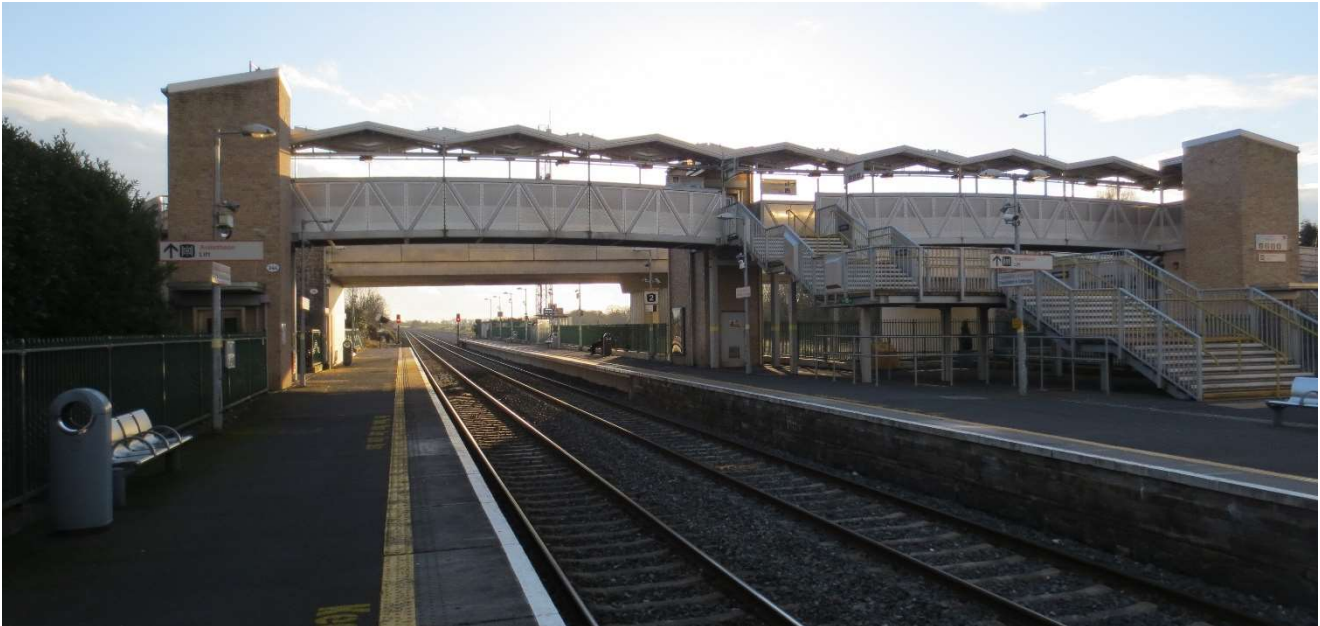
Figure 2-21 Hazelhatch Footbridge (OBC24A) East Elevation
