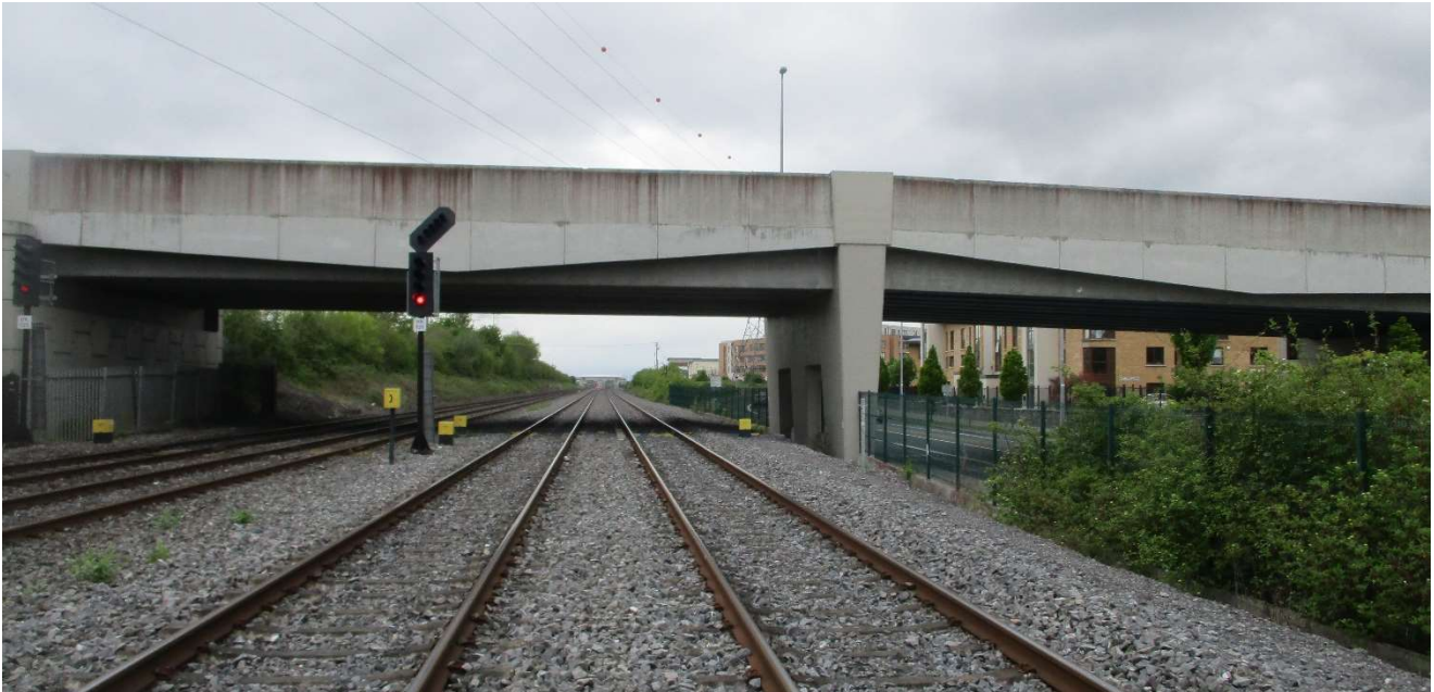
Figure 2-15 Finnstown R120 Road Bridge (OBC19) East Elevation
