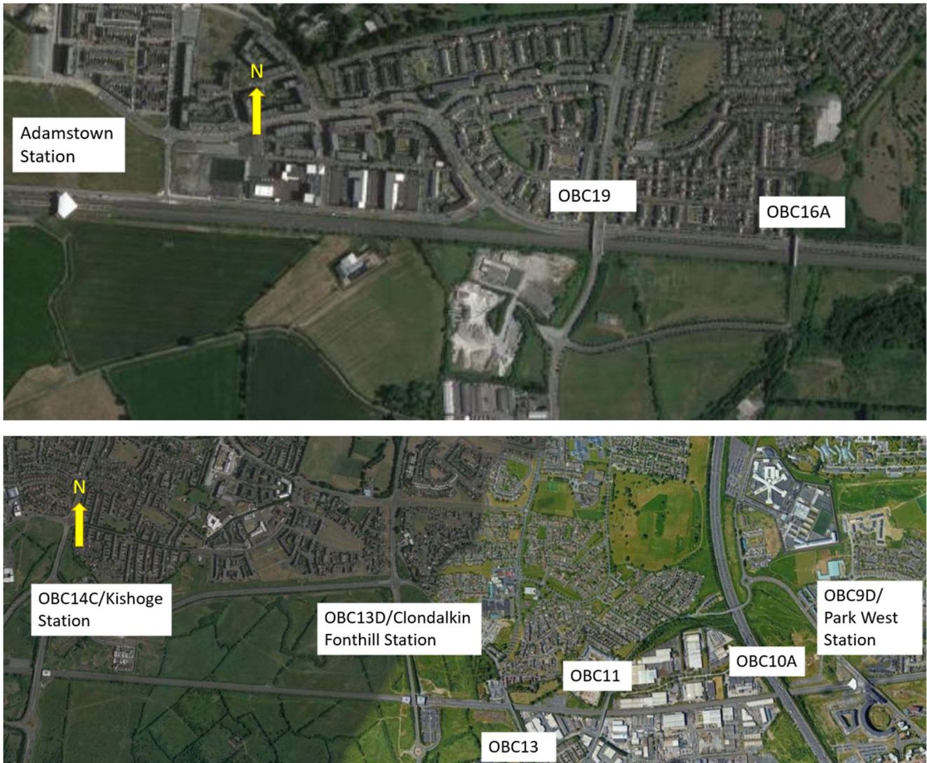
Figure 2-2 Aerial view of study area Hazelhatch – Park West
