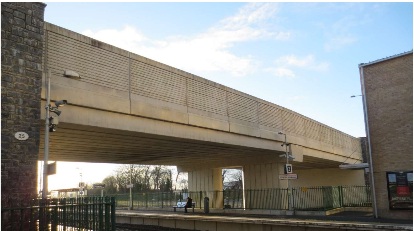
Figure 2-22 Hazelhatch R405 Road Bridge (OBC25) East Elevation
