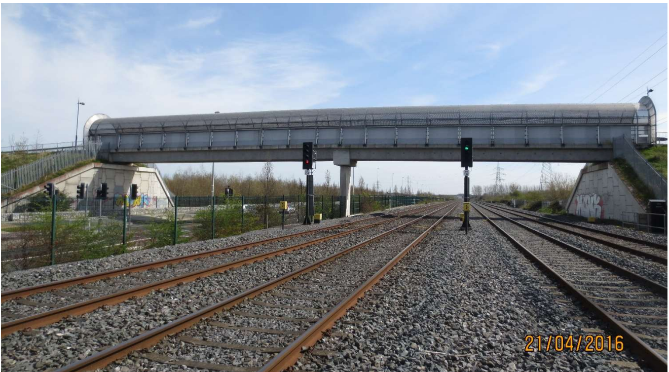
Figure 2-14 Adamstown Footbridge (OBC16A) West Elevation
