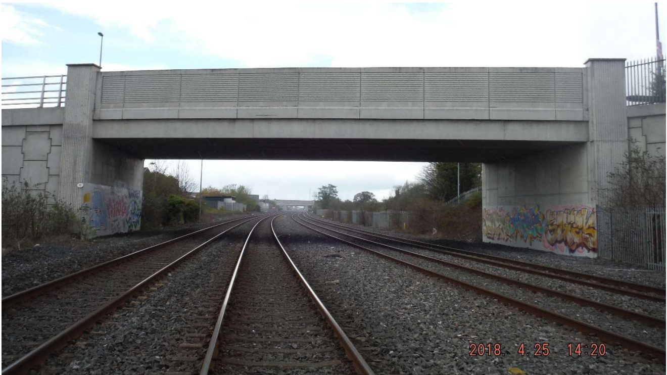
Figure 2-7 Cloverhill Road Bridge (OBC11) East Elevation
