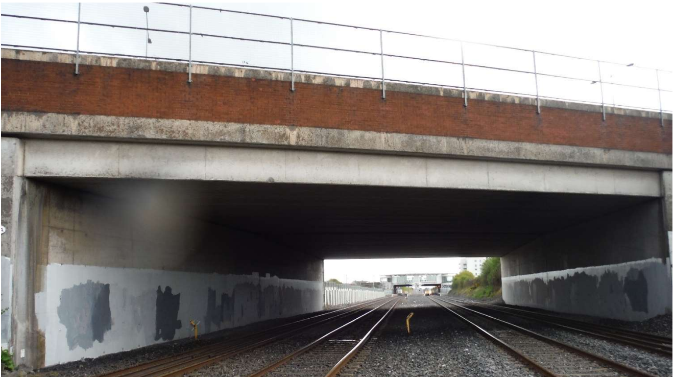
Figure 2-6 M50 Motorway Bridge (OBC10A) East Elevation
