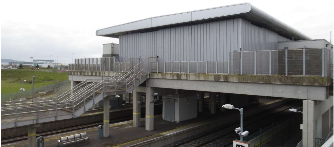
Figure 2-12 Kishoge Station Bridge (OBC14D) East Elevation
