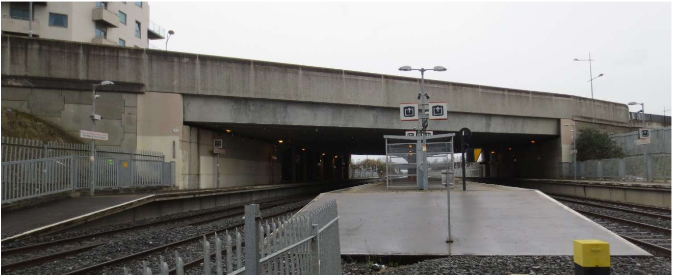
Figure 2-3 Park West Avenue Road Bridge (OBC9B) East Elevation
