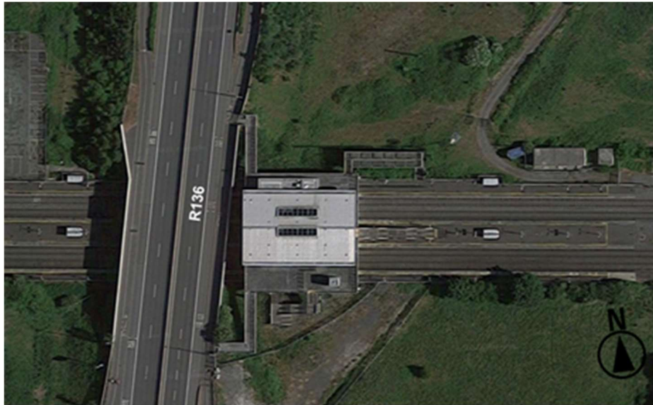
Figure 2-31 Kishoge station. Aerial view.
