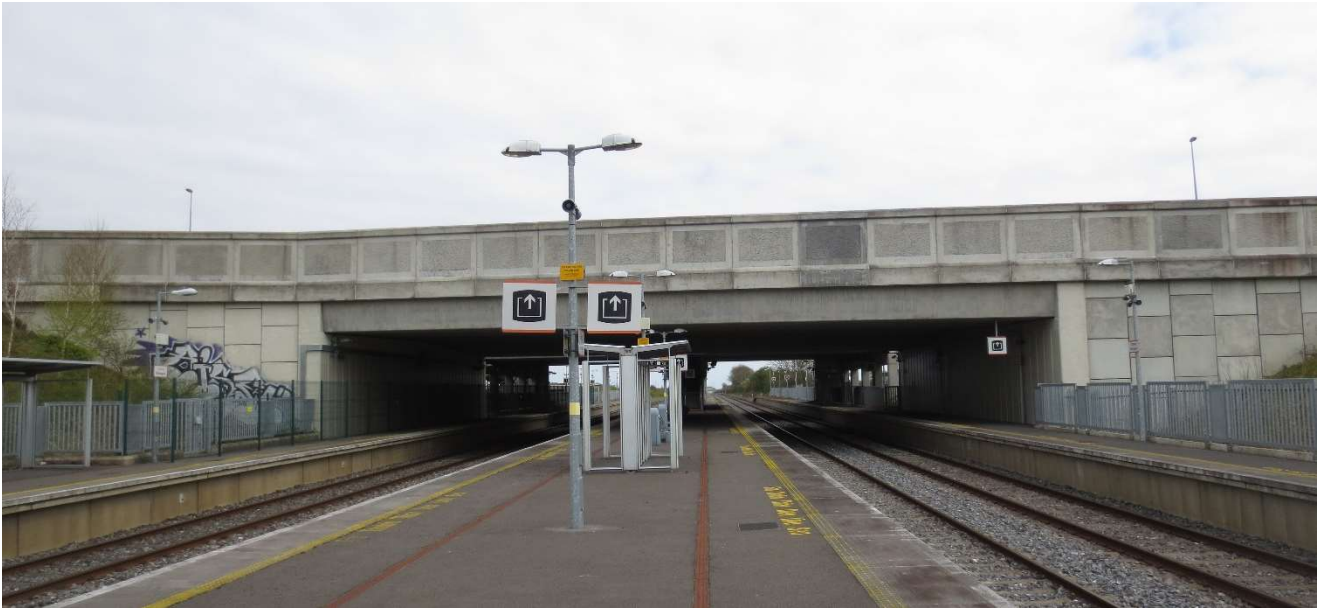
Figure 2-13 Kishoge Road Bridge (OBC14C) West Elevation
