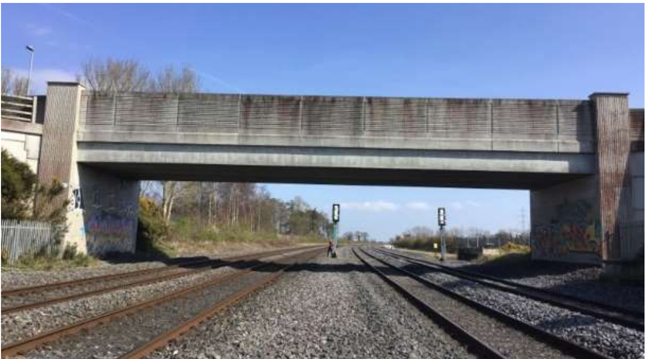
Figure 2-18 Stacumny Bridge (OBC21) West Elevation
