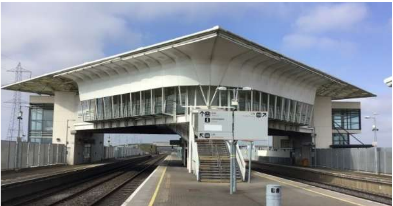
Figure 2-16 Adamstown Station Building (OBC20D) East Elevation
