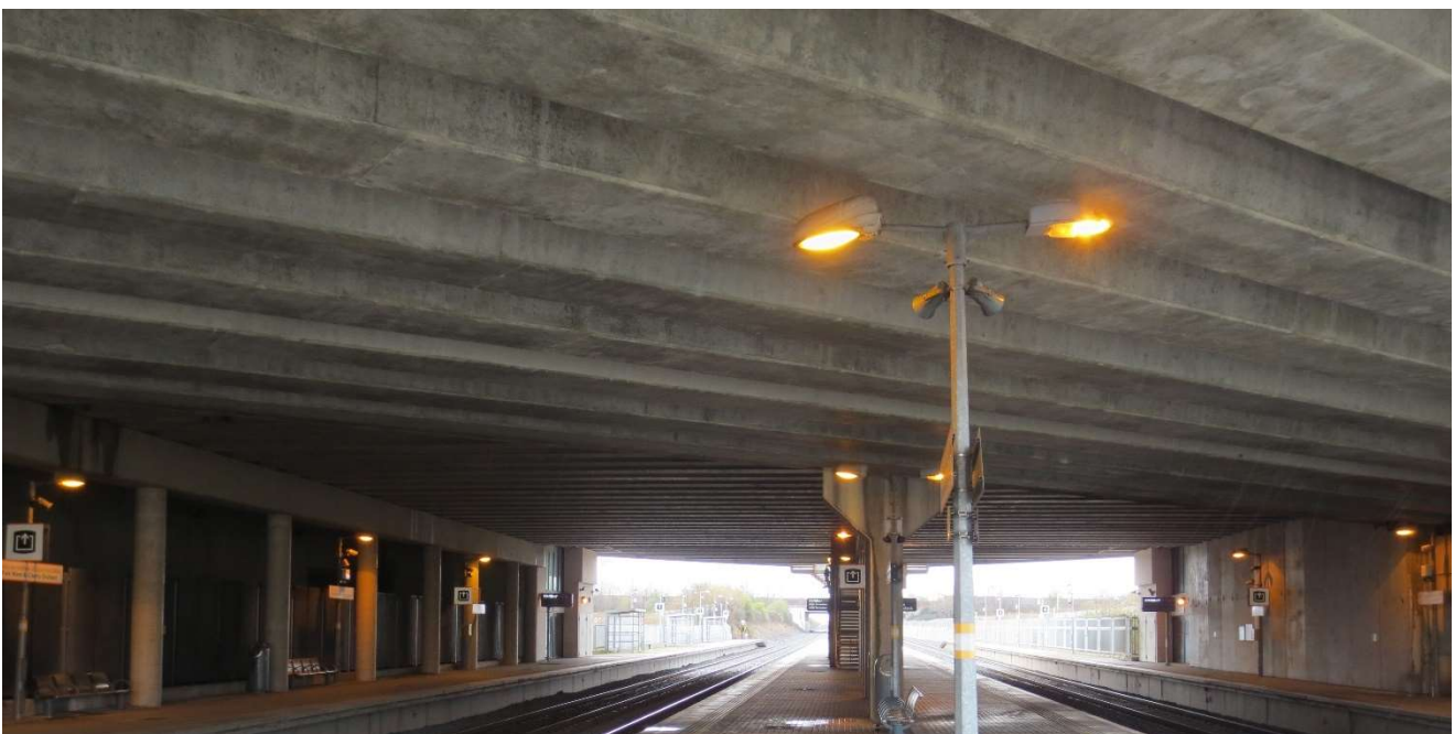
Figure 2-4 Park West Station Concourse Bridge (OBC9C) East Elevation
