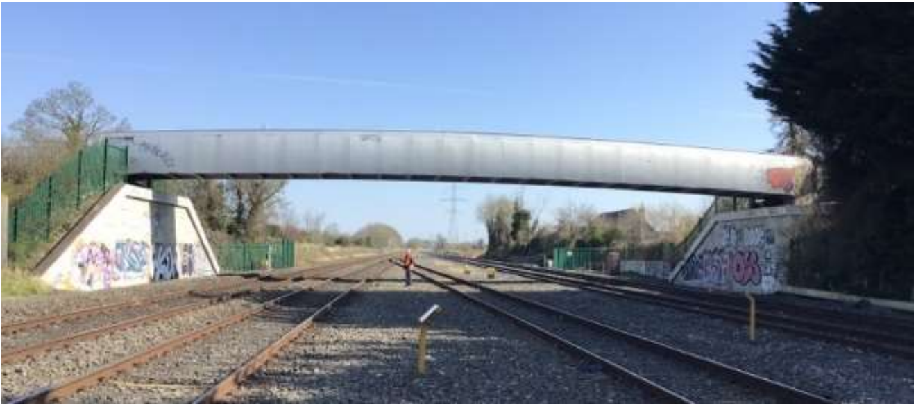
Figure 2-19 Straleek Footbridge (OBC23B) West Elevation
