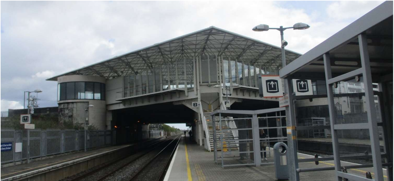
Figure 2-5 Park West Station Building Bridge (OBC9D) West Elevation
