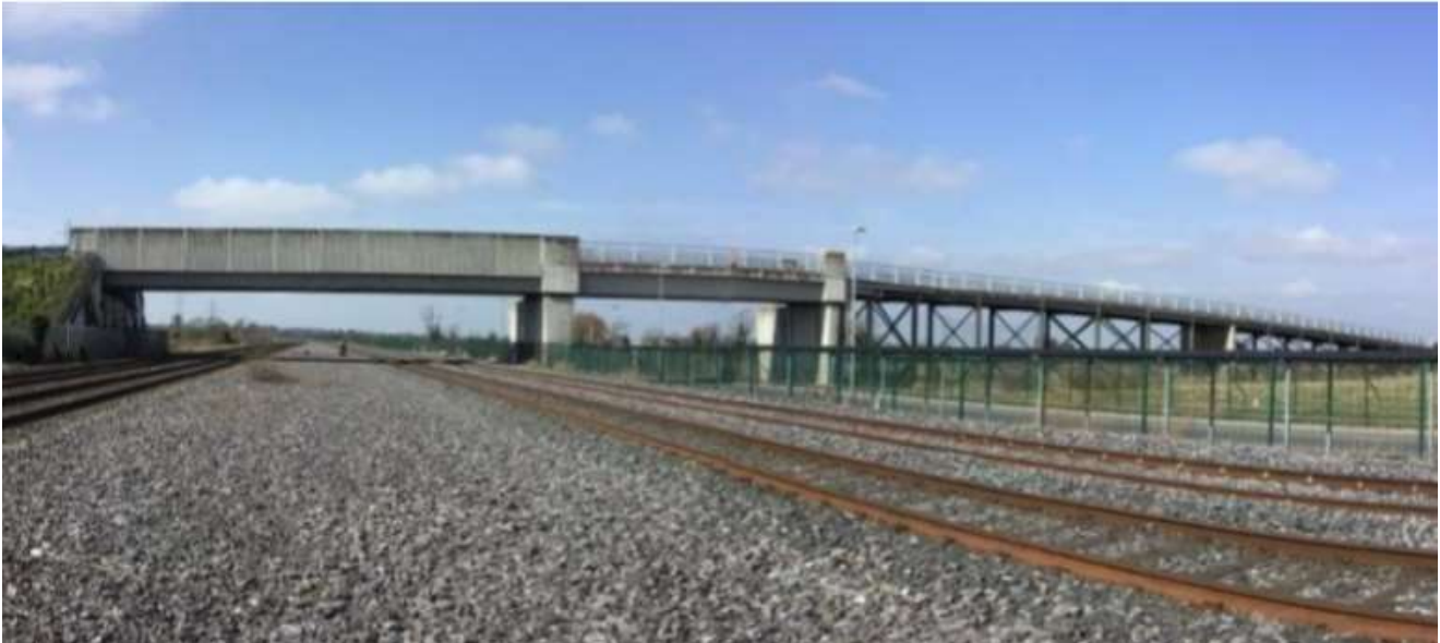
Figure 2-17 Crowley's Bridge (OBC20E) East Elevation
