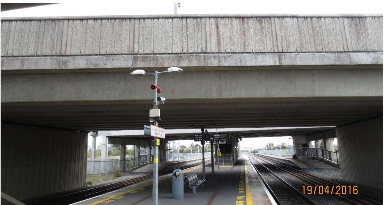
Figure 2-10 Nangor Road Bridge (OBC13A) West Elevation
