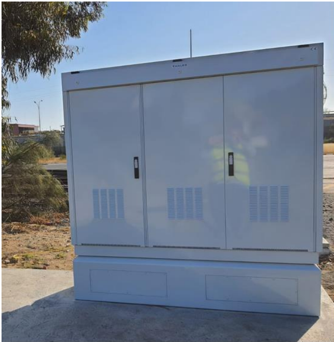
Figure 7-13 Typical Object Controller Cabinet (OBJ)
