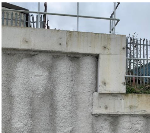
Figure 7-6 Example of a Secant Wall
