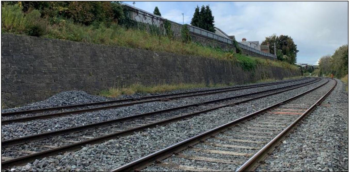
Figure 2-12 Masonry Retaining Wall on the south side of the rail corridor
