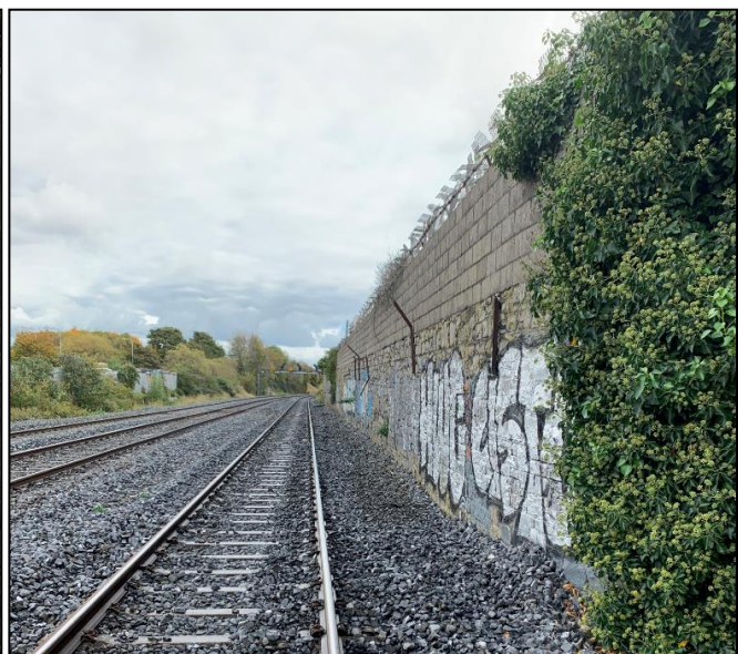
Figure 2-13 Masonry retaining wall buttress & logistics company retaining wall
