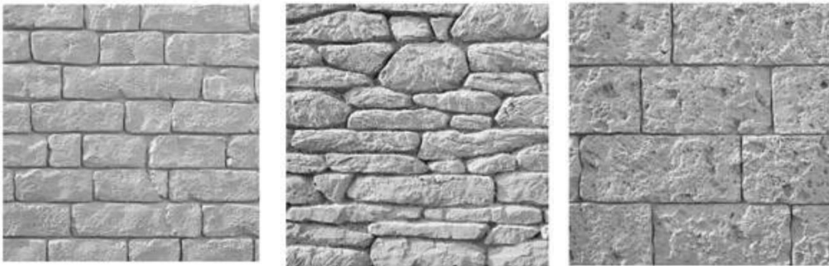
Figure 7-3 Abutment, Retaining Wall, Parapets and/or H4A containment wall finishes for precast concrete
