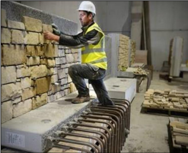
Figure 7-4 Precast panels fully clad with masonry
