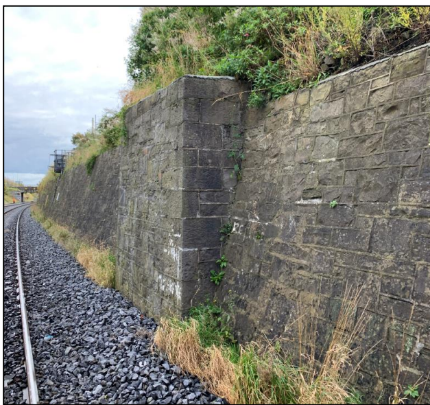
Figure 2-13 Masonry retaining wall buttress & logistics company retaining wall
