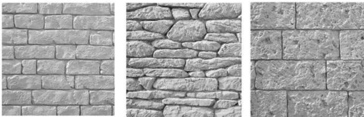
Figure 7-3 Parapets and/or H4A containment wall finishes for precast concrete
