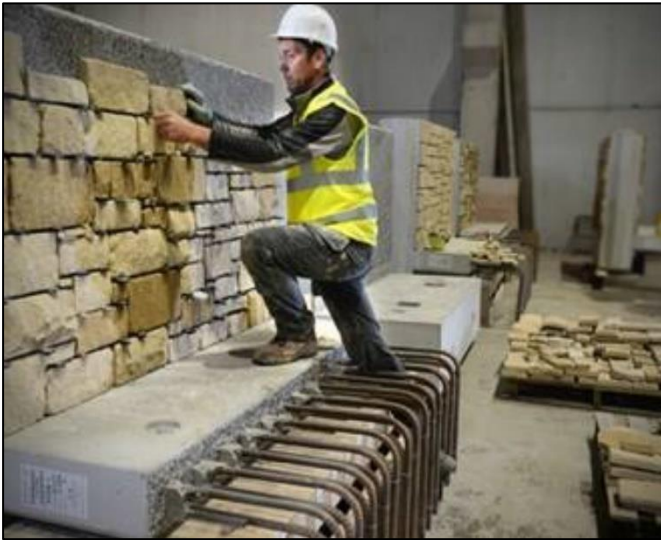
Figure 7-4 Precast panels fully cladded with masonry
