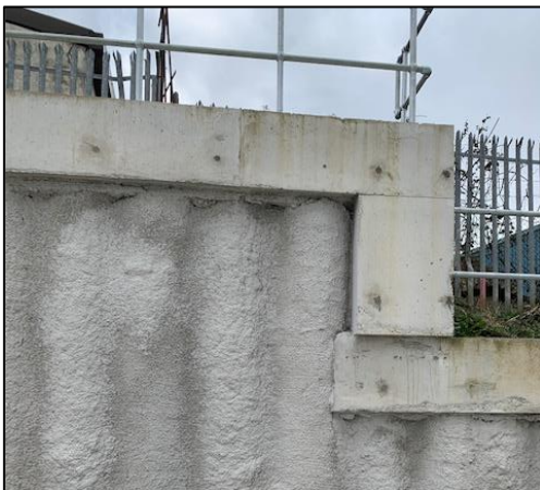
Figure 7-6 Example of a Secant Wall
