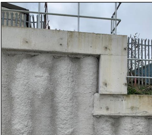
Figure 7-6 Example of a Secant Wall
