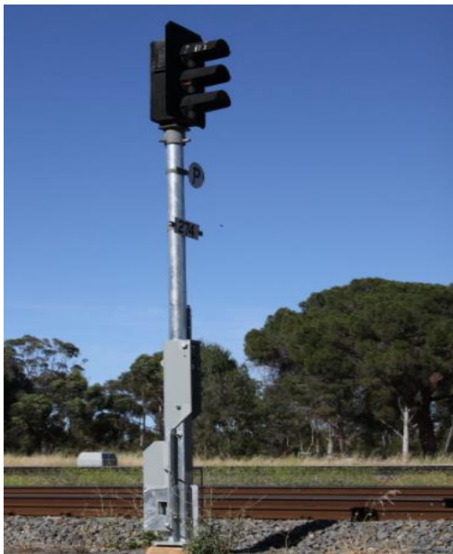
Figure 7-12 Typical Signalling Post
