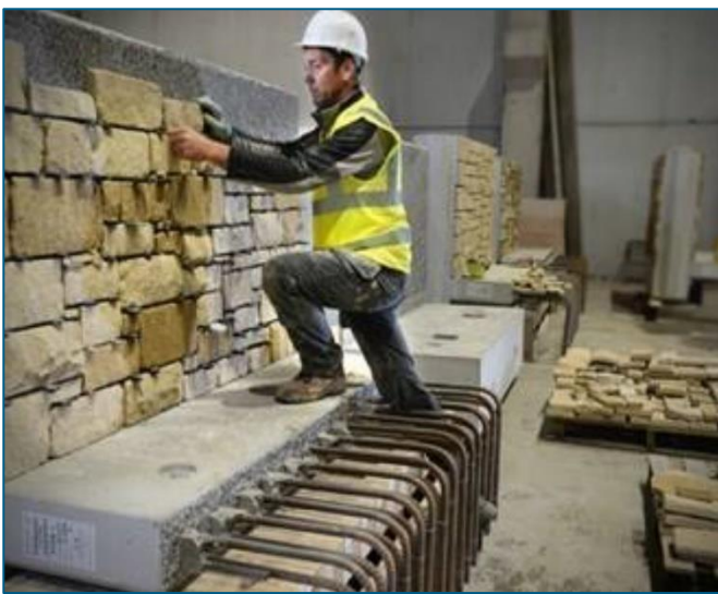
Figure 7-4 Precast panels fully clad with masonry
