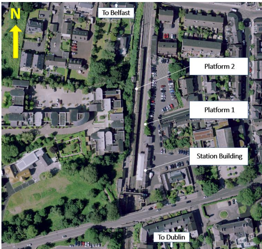
Figure 2-3: View of Malahide Station (Source: OSI aerial imagery)
