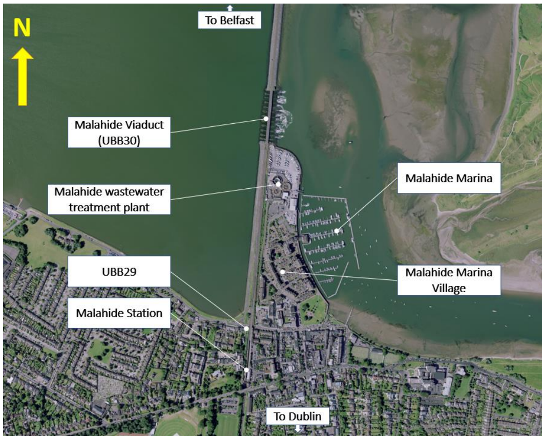
Figure 2-1: Aerial view of the Malahide area (Source: OSI aerial imagery)
