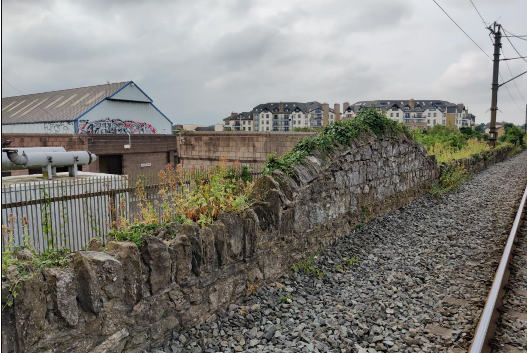
Figure 2-8: View south-east near the wastewater treatment plant (source: Arup)
