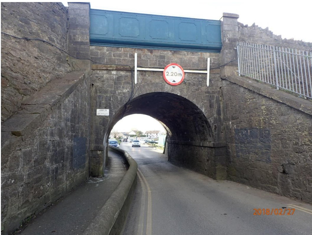
Figure 2-7: View looking west on to UBB29 (source: Irish Rail)
