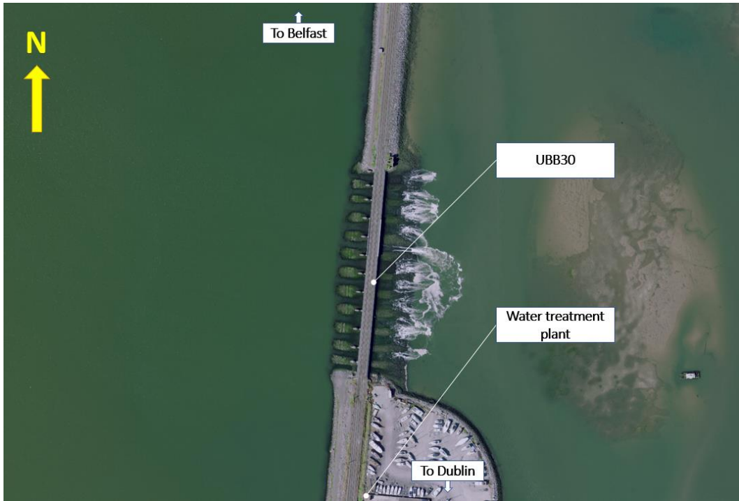
Figure 2-9: Aerial view on UBB30 carrying the Up and Down Belfast lines over the estuary (source: OSI aerial mapping)
