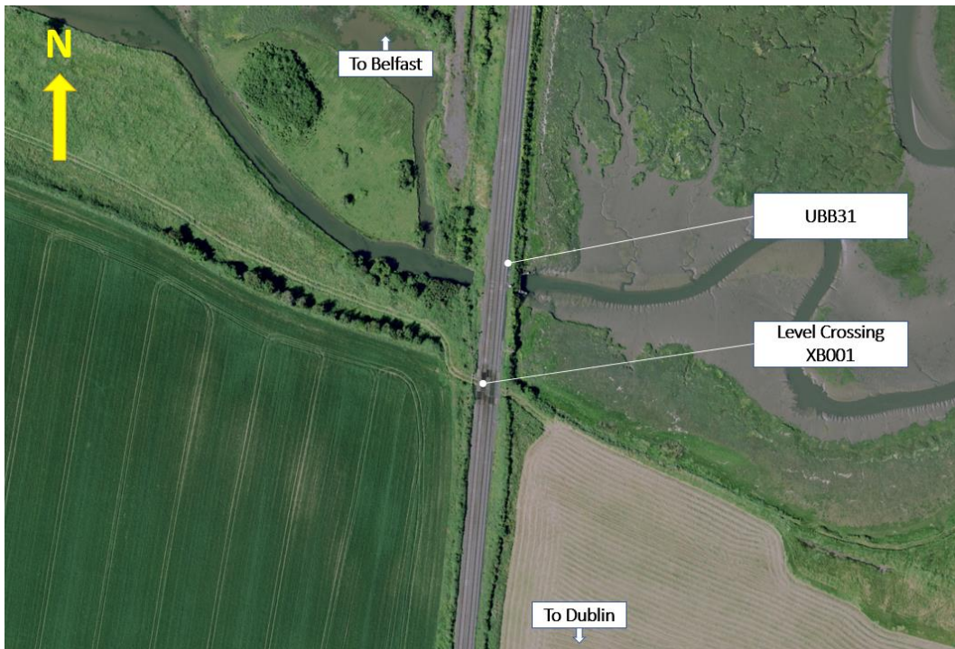
Figure 2-10: Aerial view on UBB31 (source: OSI aerial mapping)
