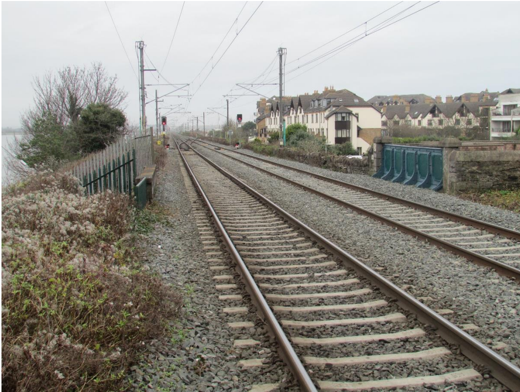
Figure 2-6: View of existing track over UBB29 (source: Arup)
