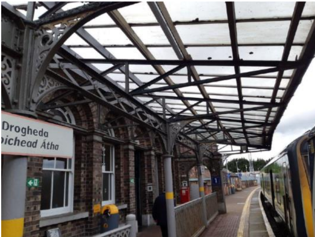
Figure 5-41 Drogheda Platform 1 Canopy (Source: Arup)
