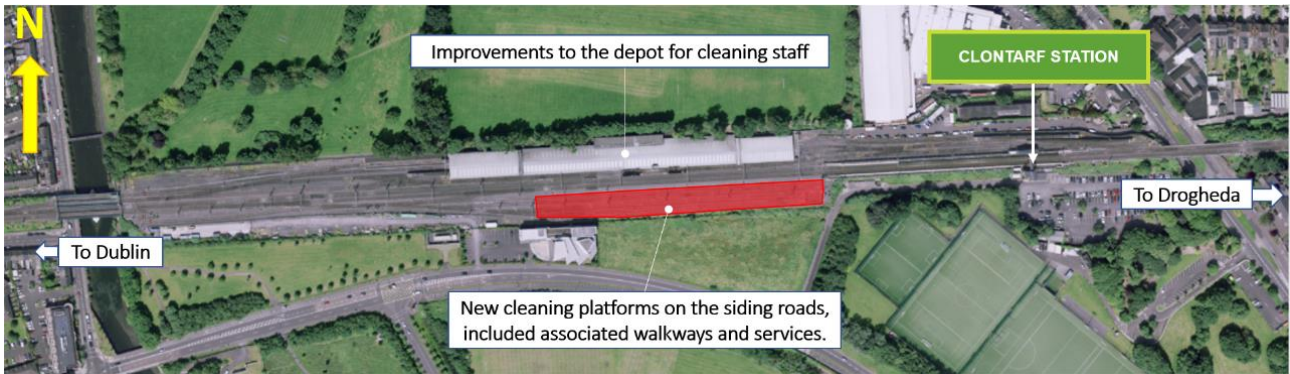
Figure 6-3 Fairview Depot works overview
