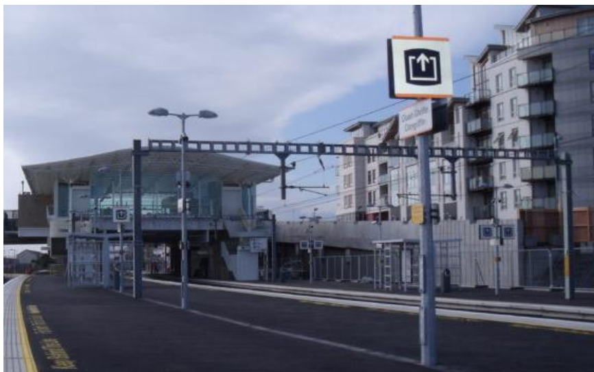
Figure 5-7: Existing portal at Clongriffin Station
