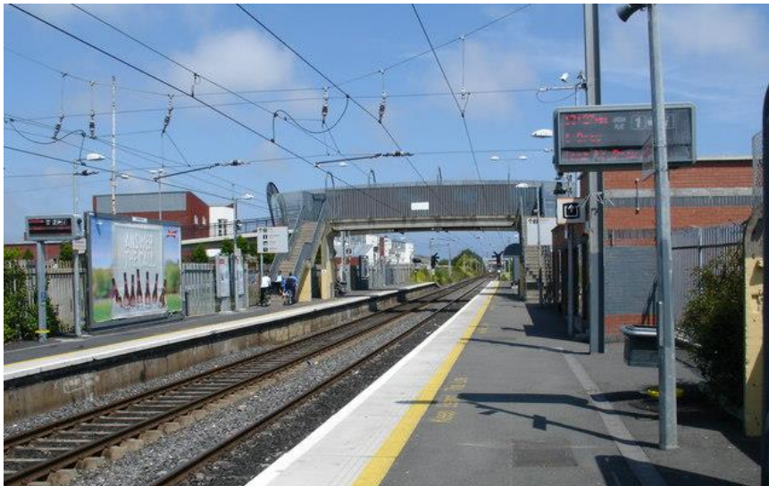
Figure 5-6: Existing head span at Howth Station
