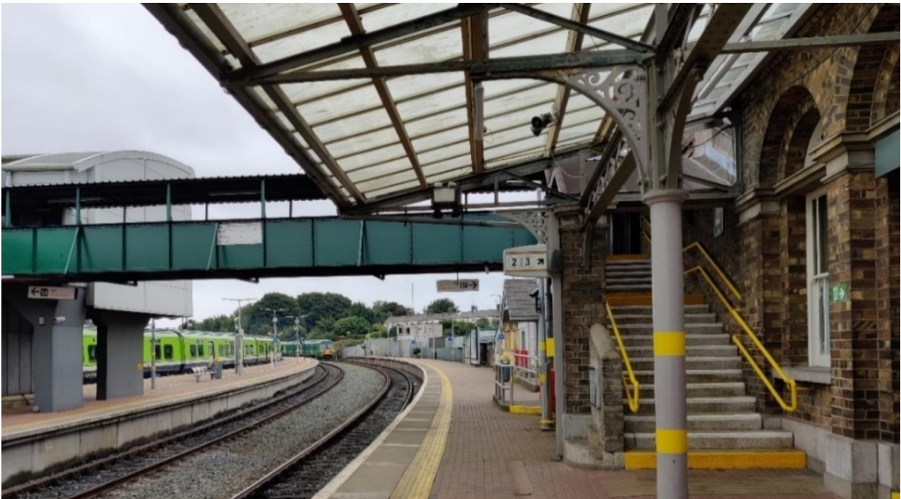
Figure 5-28 OBB81 bridge elevation and stairs access from Platform 1
