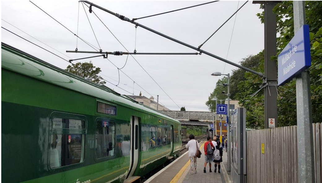
Figure 5-4: Existing single-track cantilevers at Malahide Station
