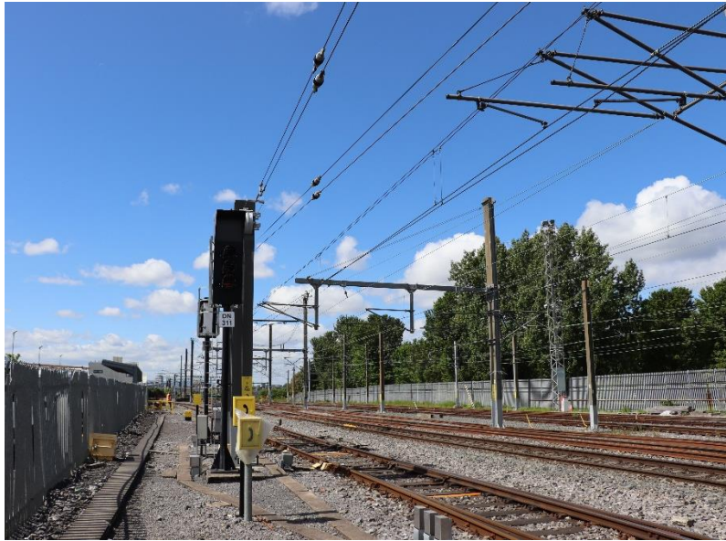
Figure 5-1: An example of OHLE on an existing line
