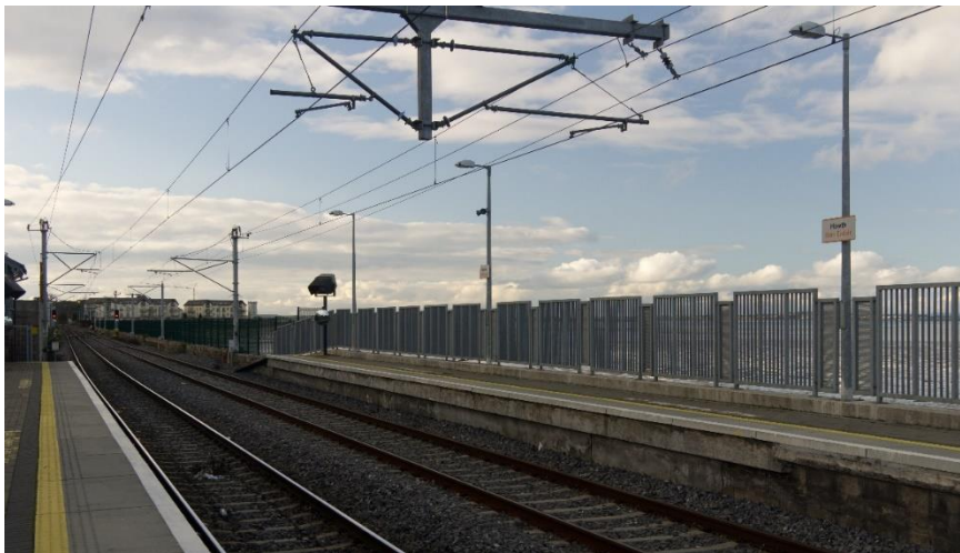
Figure 5-5: Current two track cantilever at Kilbarrack Station
