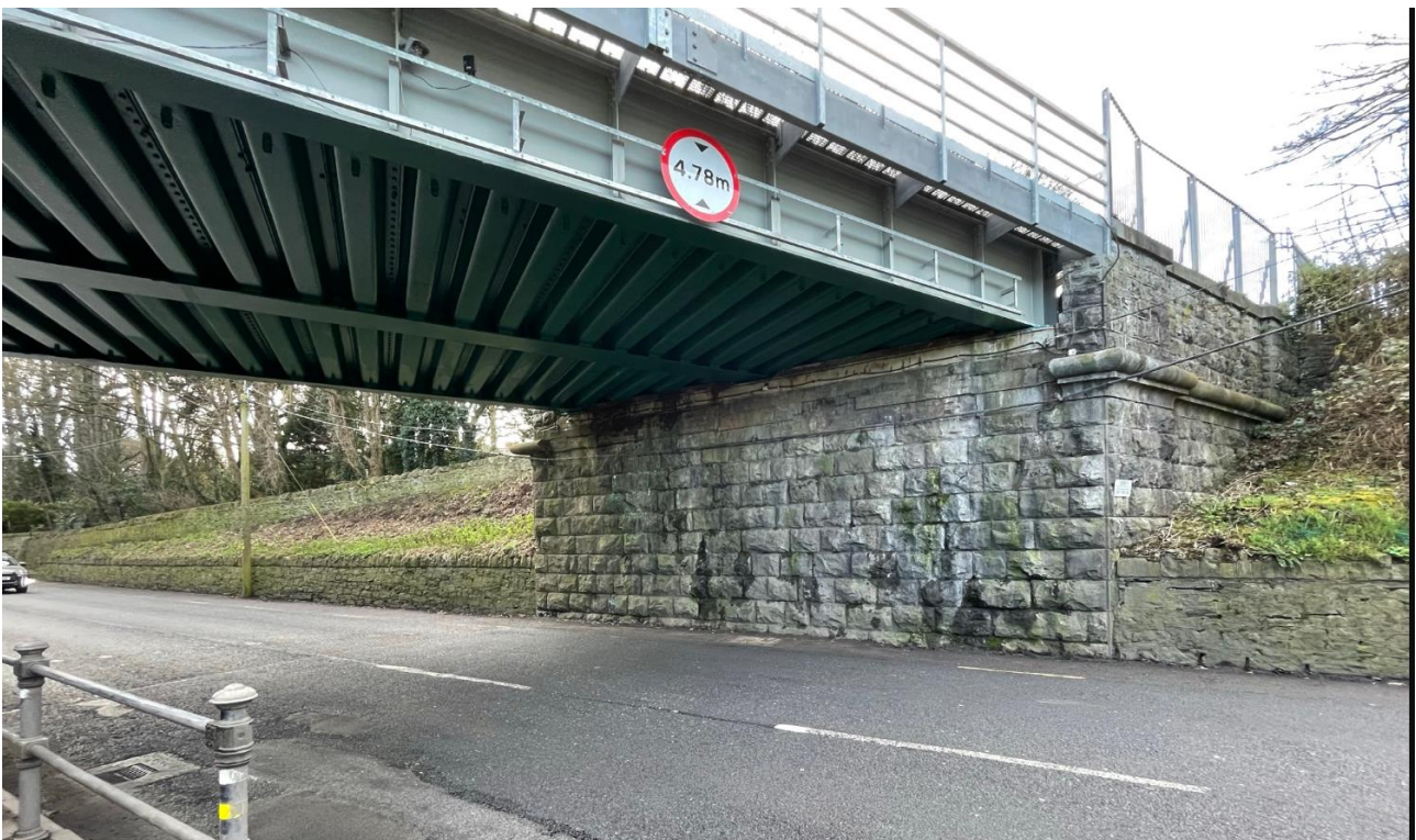
Figure 11-6 Dublin Road Bridge (UKB1)
