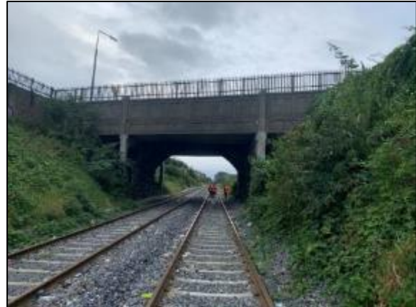
Faussagh Road Bridge (OBO7)
