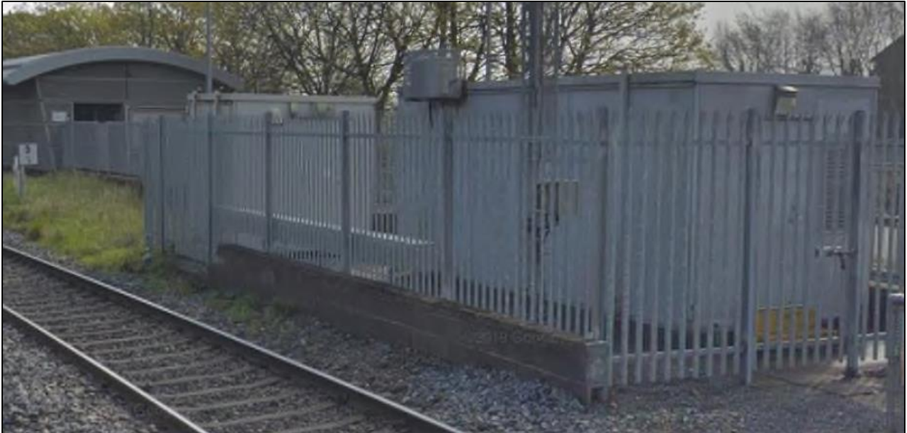
Figure 5-5 Typical Telecom Equipment Building
