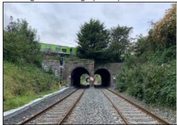
Maynooth Line Twin Arch (OBO9)
