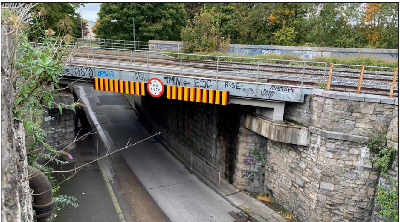
Figure 7-26 Sarsfield Road Bridge
