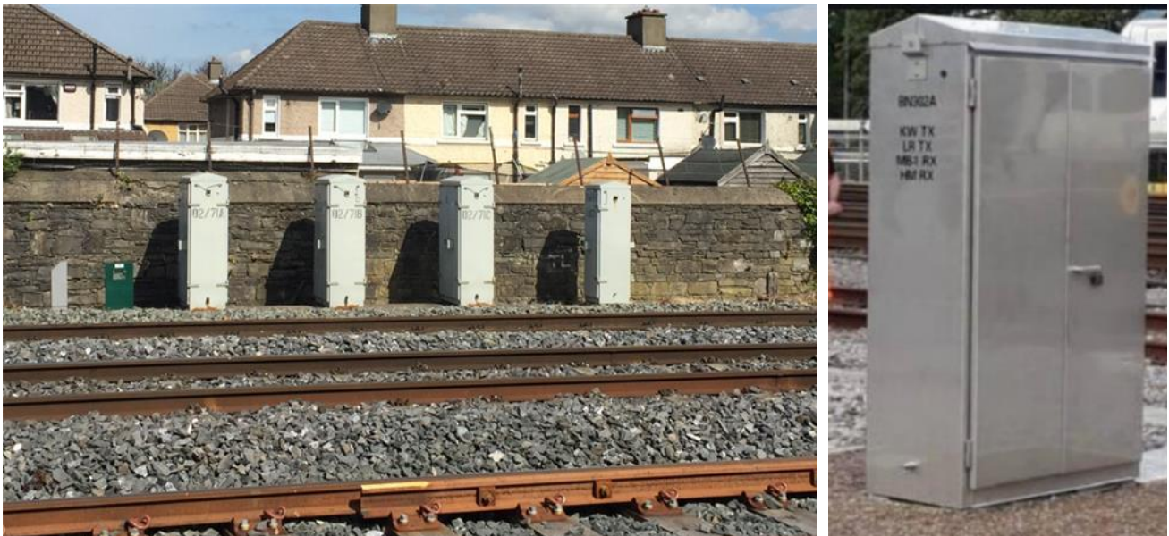
Figure 5-2 Examples of typical Object Controller Cabinet (OBJ) and Location Case
