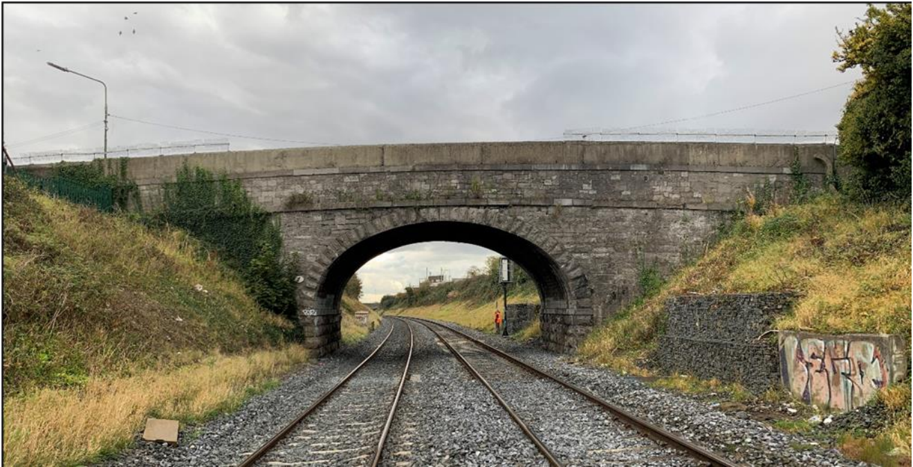
Figure 7-3 Le Fanu Road Bridge - West Elevation
