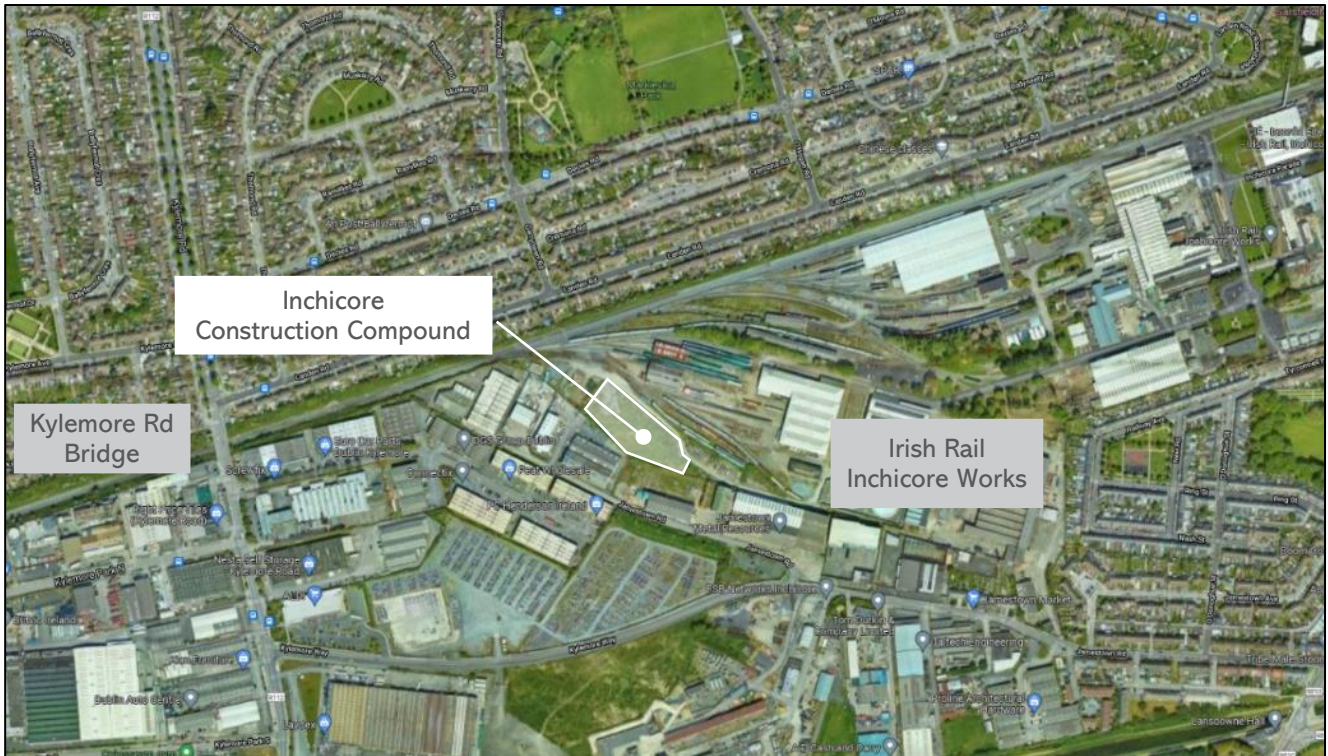
Figure 7-22 Inchicore Preferred Construction Compound Location
