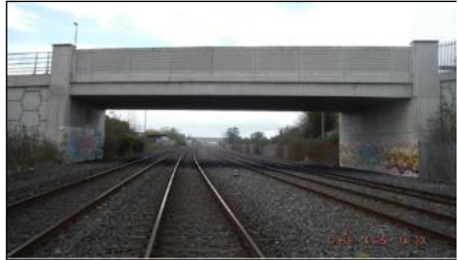
Station Road / Cloverhill Road Bridge (OBC11)
