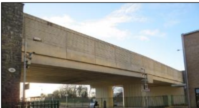
Hazelhatch R405 Road Bridge (OBC25)
