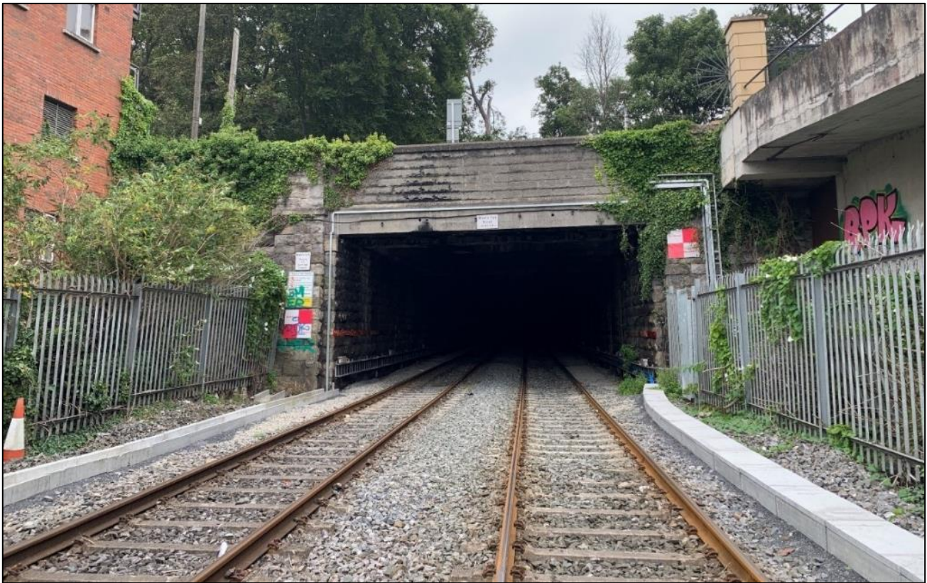
Figure 8-2 Phoenix Park Tunnel Entrance
