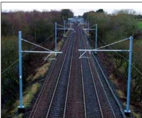
Figure 5-6 Typical OHLE Mast Arrangement
