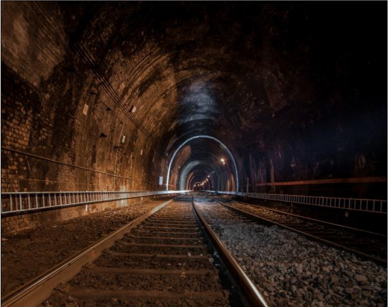
Figure 8-7 View Inside the Phoenix Park Tunnel
