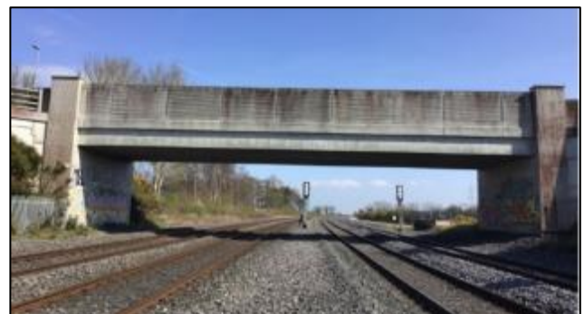
Stacumny Road Bridge (OBC21)
