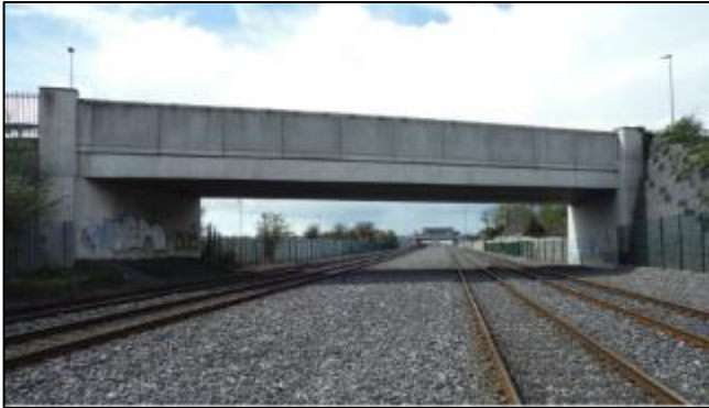
Ninth Lock Road Bridge (OBC13)
