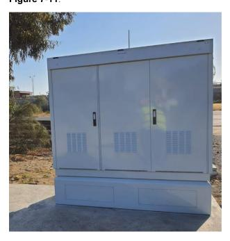
Figure 7-11 Typical Object Controller Cabinet
