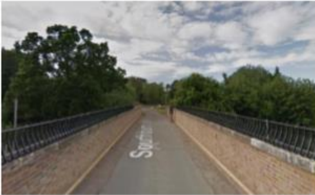
Option 1: Increased Parapet Heights to Achieve Safety Requirements for OHLE
