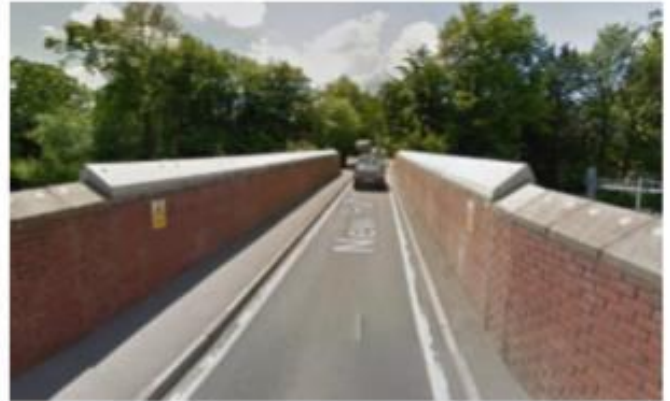
Option 1: Increased Parapet Heights to Achieve Safety Requirements for OHLE
