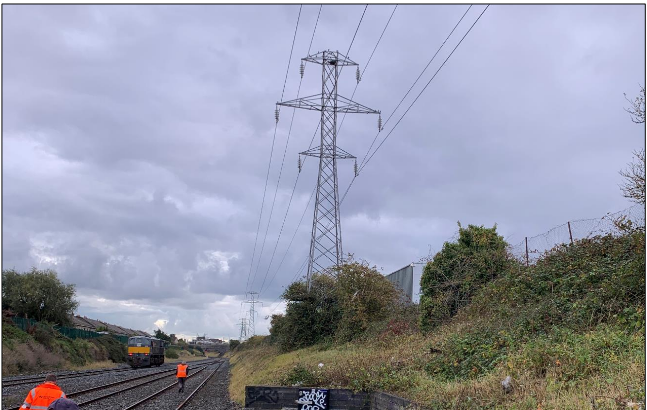
Figure 4-3 High voltage transmission lines along south of rail corridor (Facing East)
