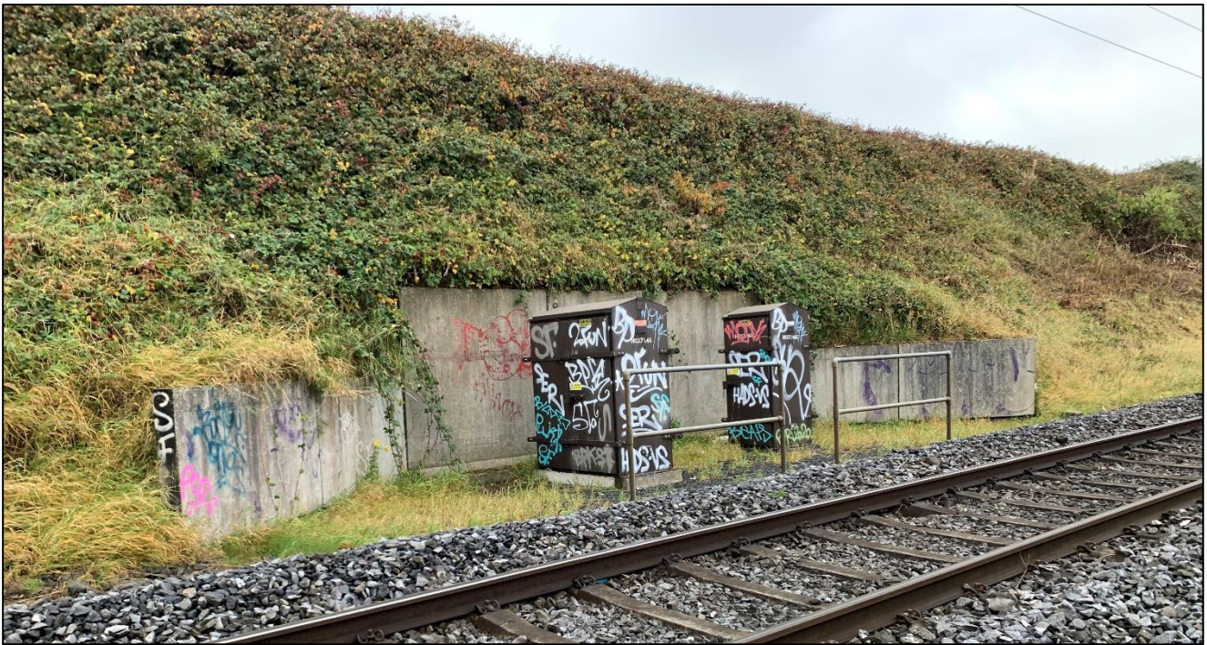
Figure 2-12 RC retaining wall east of Le Fanu Road Bridge (OBC7)
