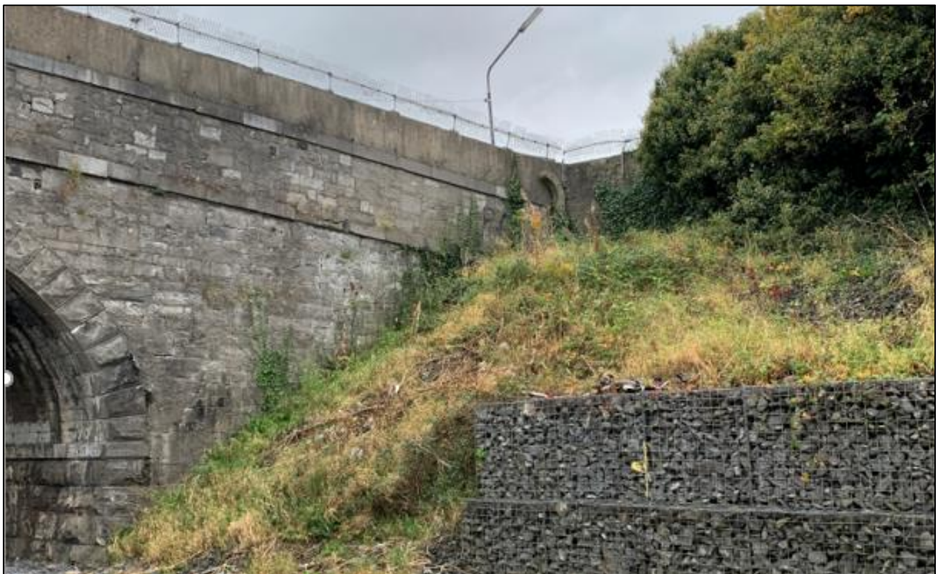
Figure 5-1 Le Fanu Road Bridge (OBC7) wingwall, south-west
