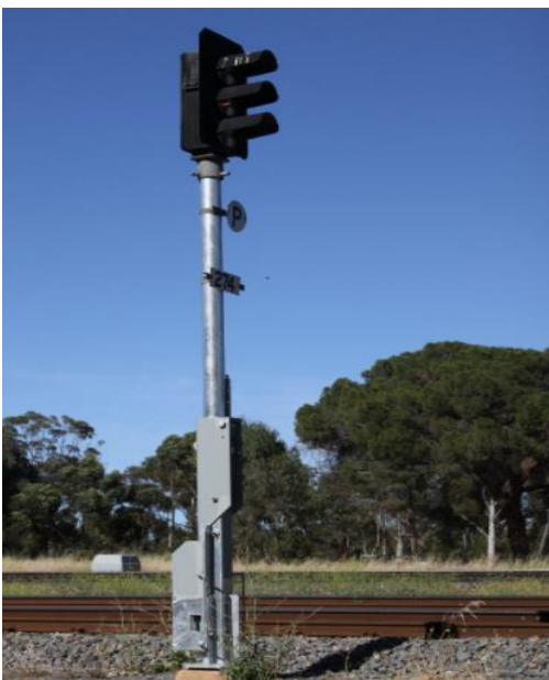
Figure 7-13 Typical Signalling Post
