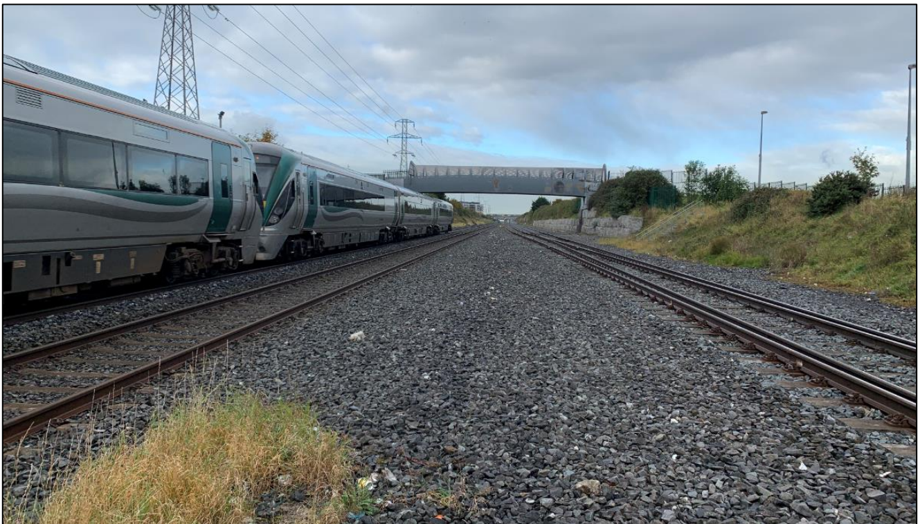
Figure 2-14 Cherry Orchard Footbridge (OBC8B) and Points 802 on right (Facing West)
