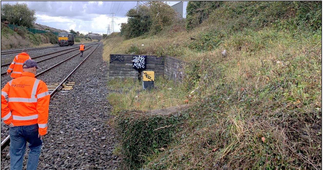
Figure 2-9 Blockwork Headwall - Facing East
