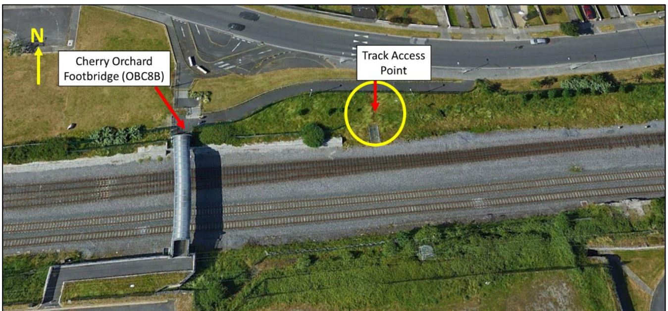
Figure 2-16 Track access point on the east side of Cheery Orchard Footbridge (OBC8B)
