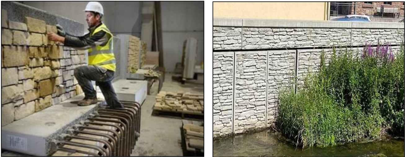
Figure 7-4 Precast panels fully clad with masonry
