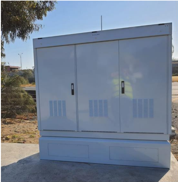
Figure 7-14 Typical Object Controller Cabinet (OBJ)
