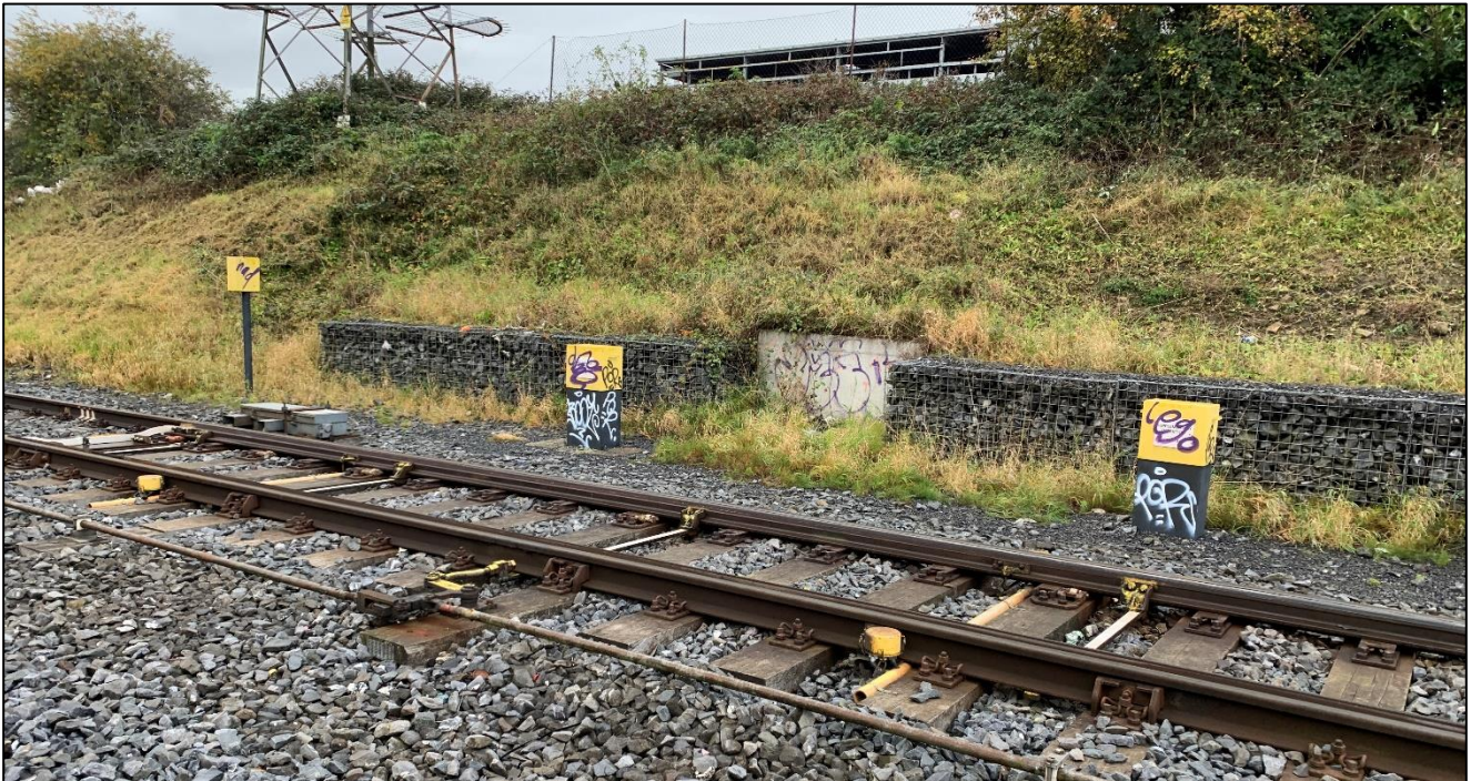
Figure 2-11 Gabion retaining wall along southern edge of cess.
