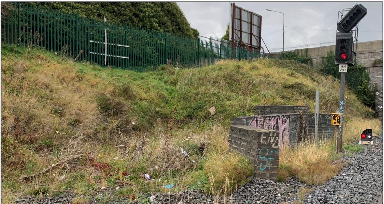
Figure 2-13 Blockwork headwall east of Le Fanu Road Bridge (OBC7)
