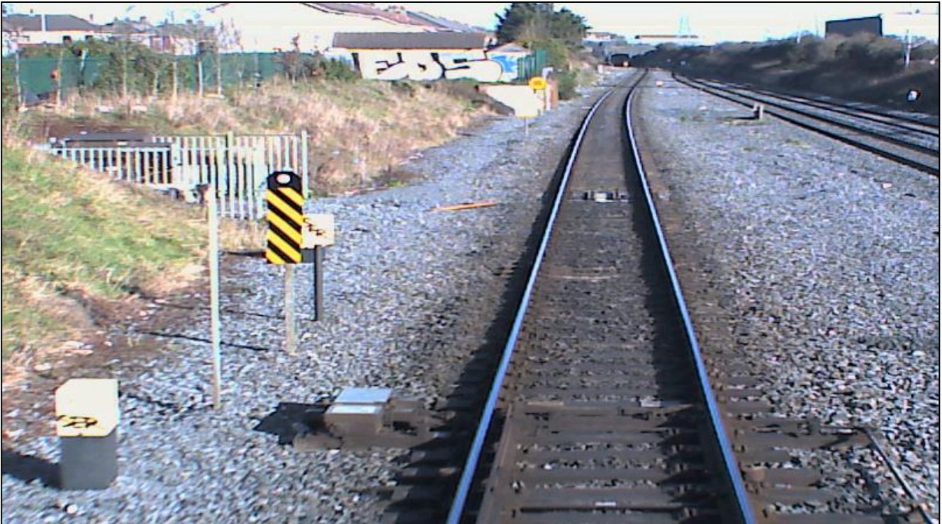
Figure 2-8 Blockwork Headwall and Fencing - Facing East
