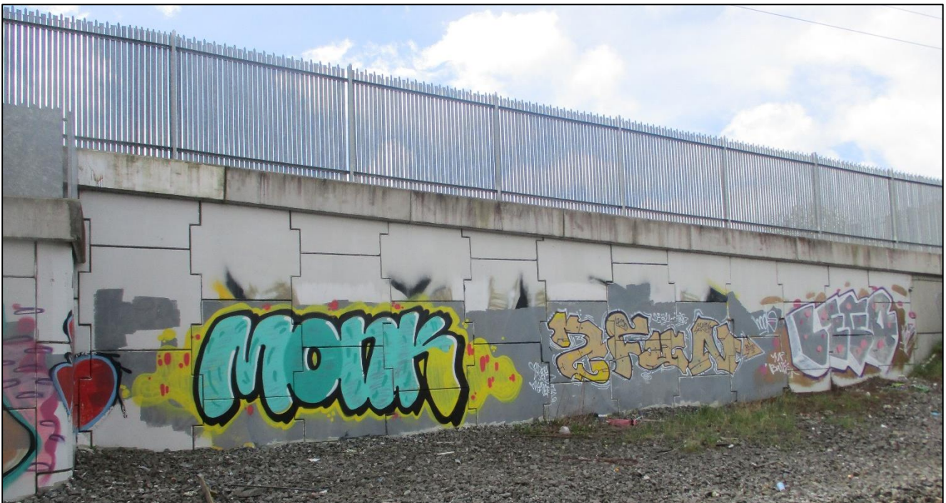
Figure 2-5 MSE Retaining Wall, south-west side of Cherry Orchard Footbridge (OBC8B)
