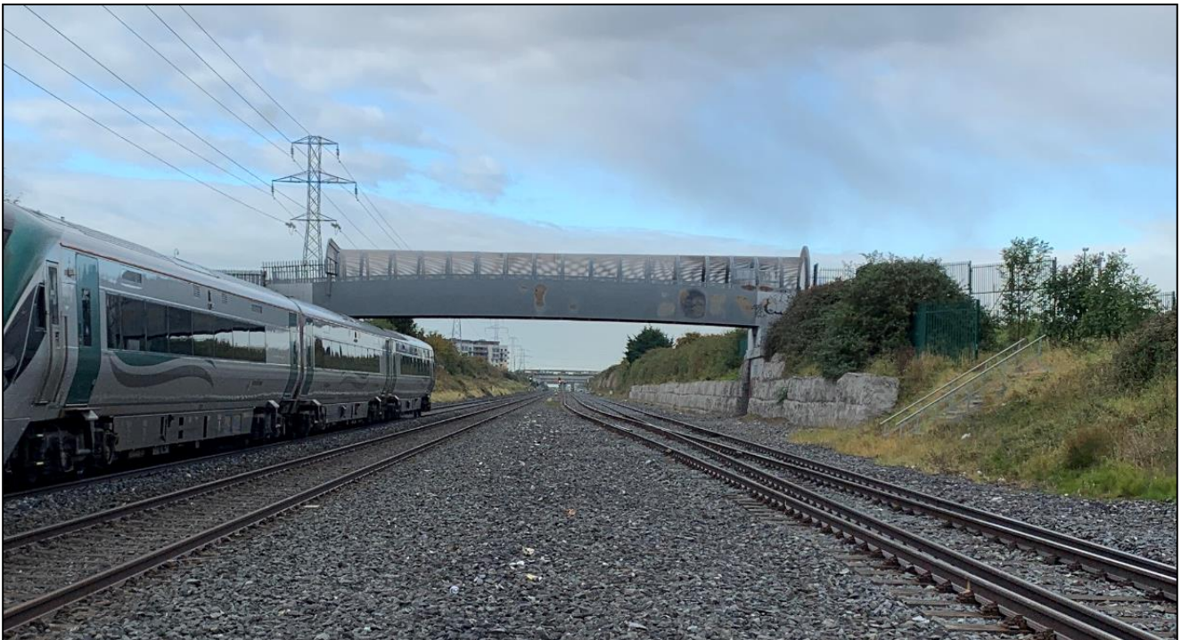
Figure 2-2 Cherry Orchard Footbridge (OBC8B) - east elevation
