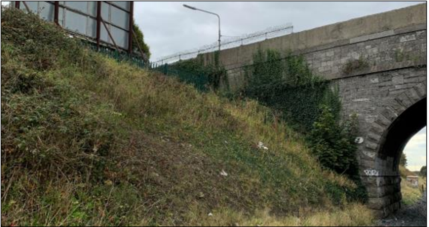
Figure 5-2 Le Fanu Road Bridge (OBC7) wingwall, north-west
