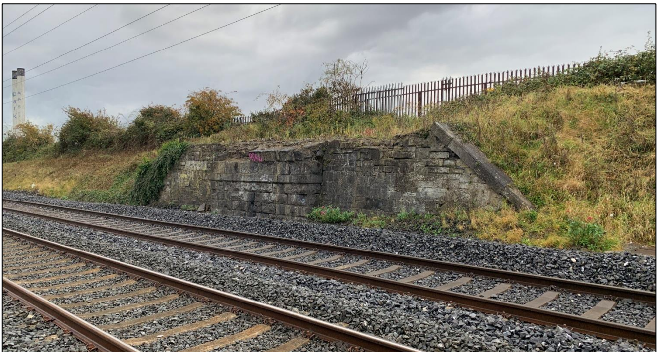
Figure 2-7 Masonry retaining wall (possibly a partially defunct bridge abutment)
