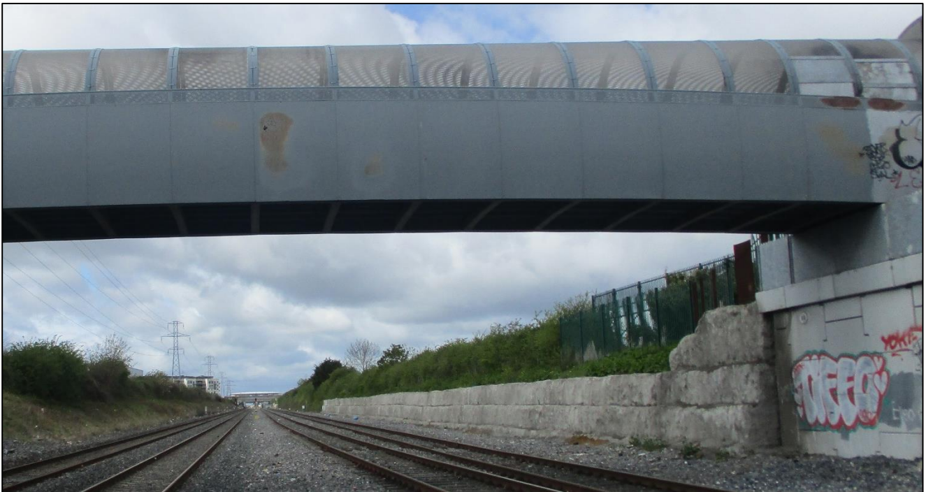
Figure 2-4 Masonry Retaining Wall, north-west side of Cherry Orchard Footbridge (OBC8B)
