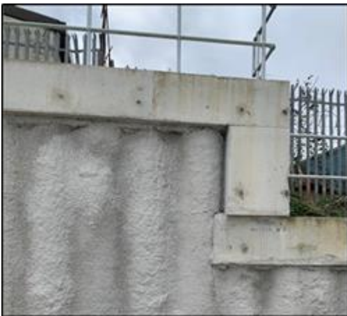
Figure 7-6 Example of a Secant Wall
