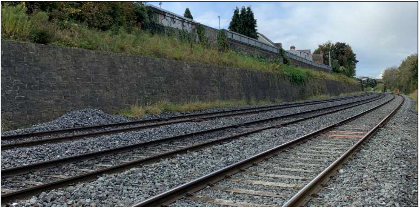
Figure 2-8 Masonry Retaining Wall on the south side of the rail corridor
