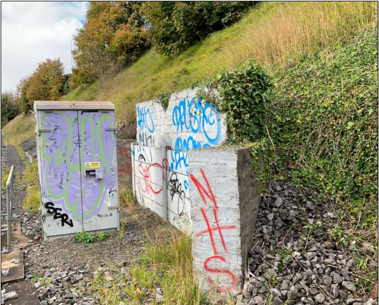
Figure 2-12 Blockwork headwall at on the north side of tracks (east end of the area)
