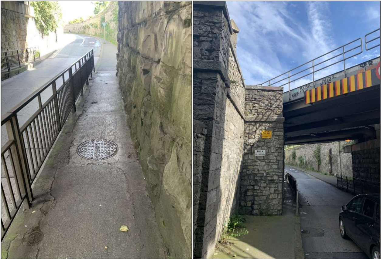
Figure 2-4 Sarsfield Road Bridge (UBC4) - East footway & West abutment
