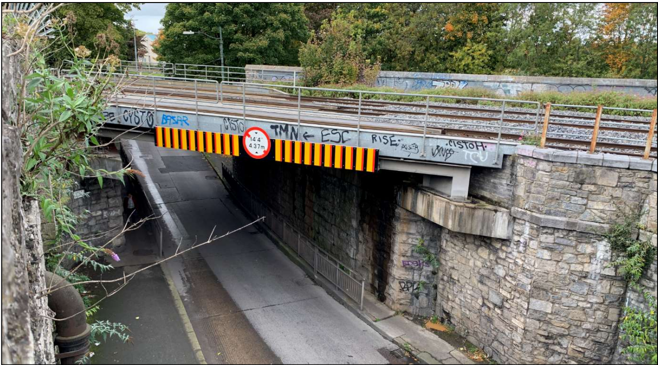
Figure 2-2 Sarsfield Road Bridge (UBC4) - South Elevation
