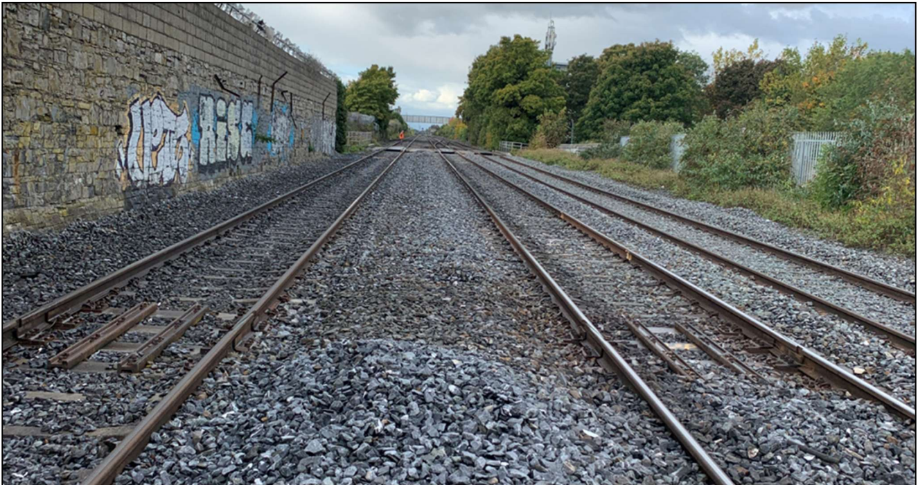
Figure 2-16 Adjustment switches on Relief Line (LHS) and Down Main (Centre).
