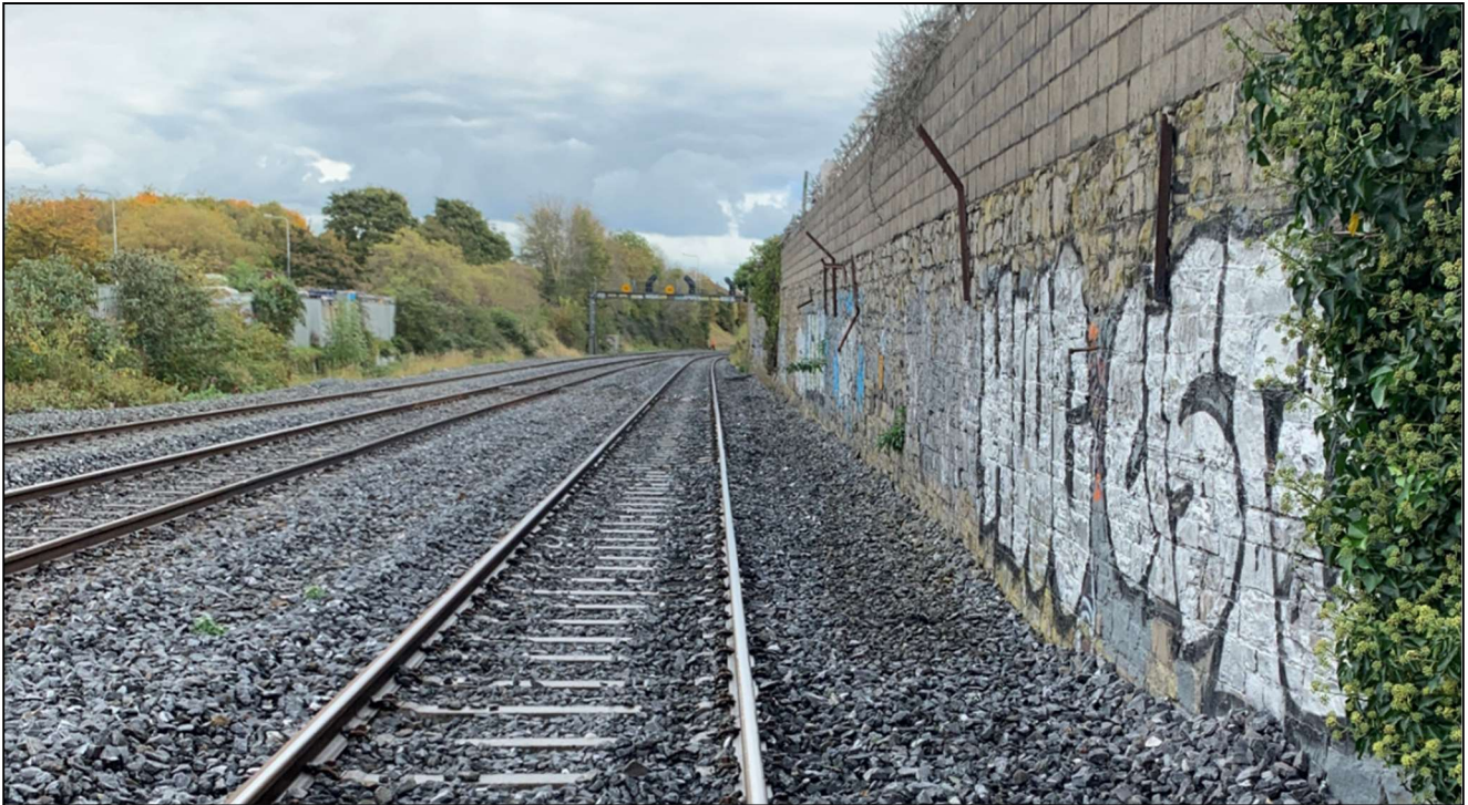
Figure 2-14 Clearance from boundary wall to outer rail is 1.7m - Facing East
