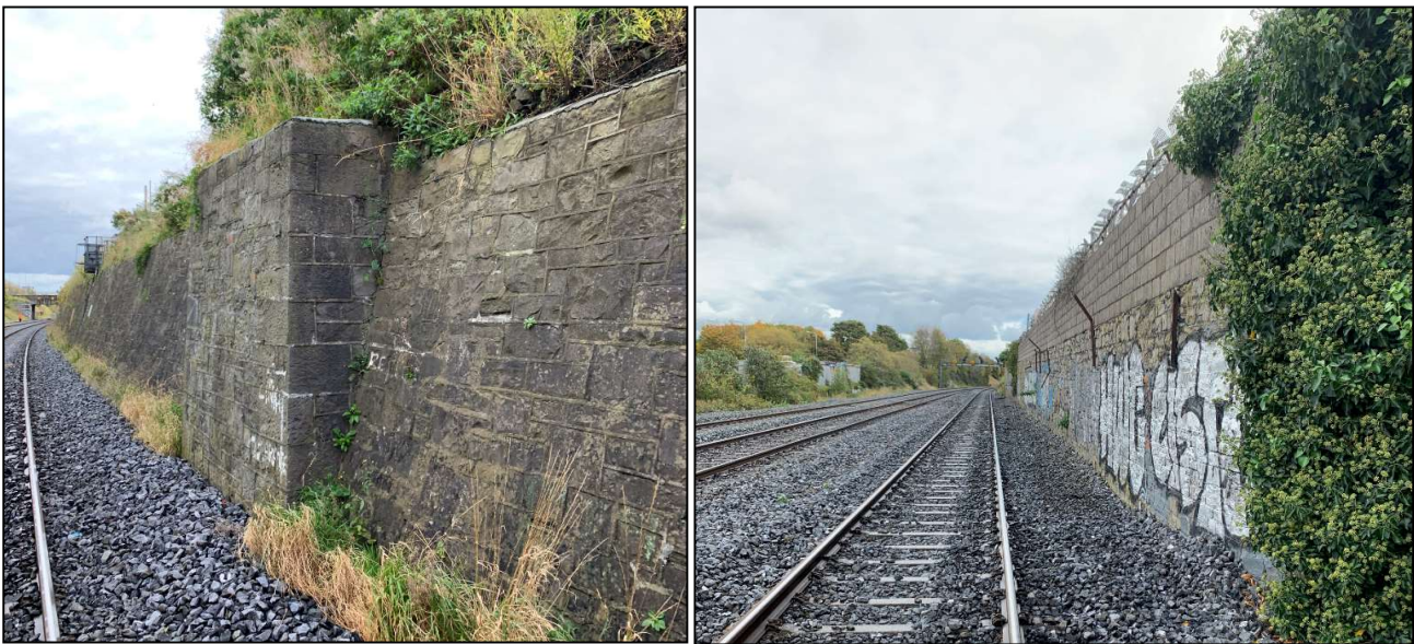
Figure 2-9 Masonry retaining wall buttress & logistics company retaining wall
