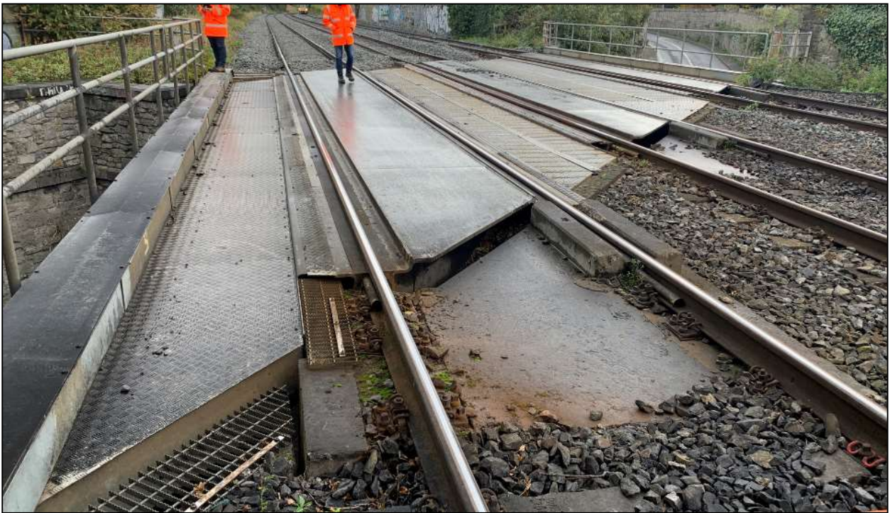
Figure 2-5 Sarsfield Road Bridge (UBC4) Deck level - Facing East
