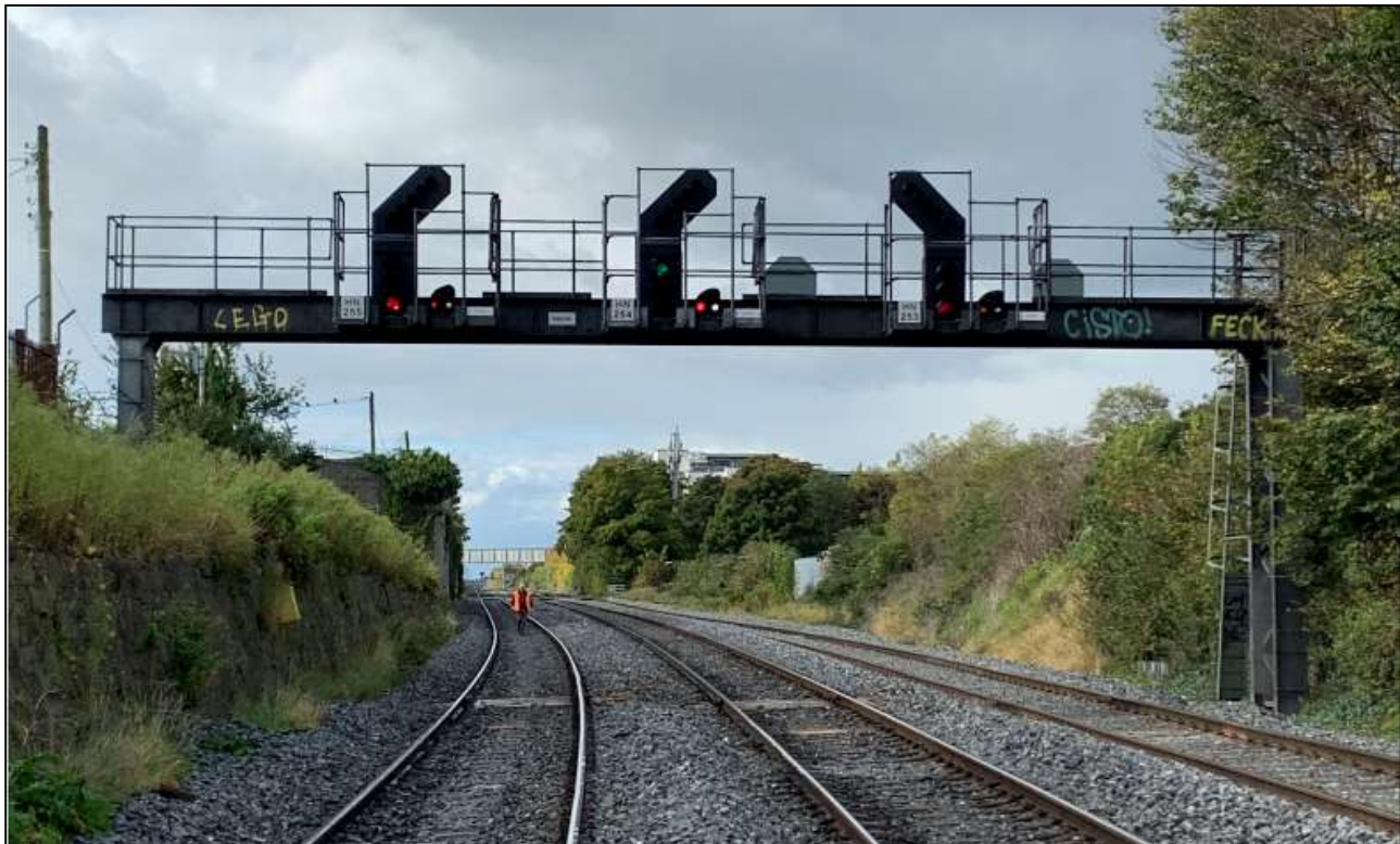
Figure 2-7 Portal signal gantry (OBC3A) - west of Sarsfield Road Bridge (UBC4)
