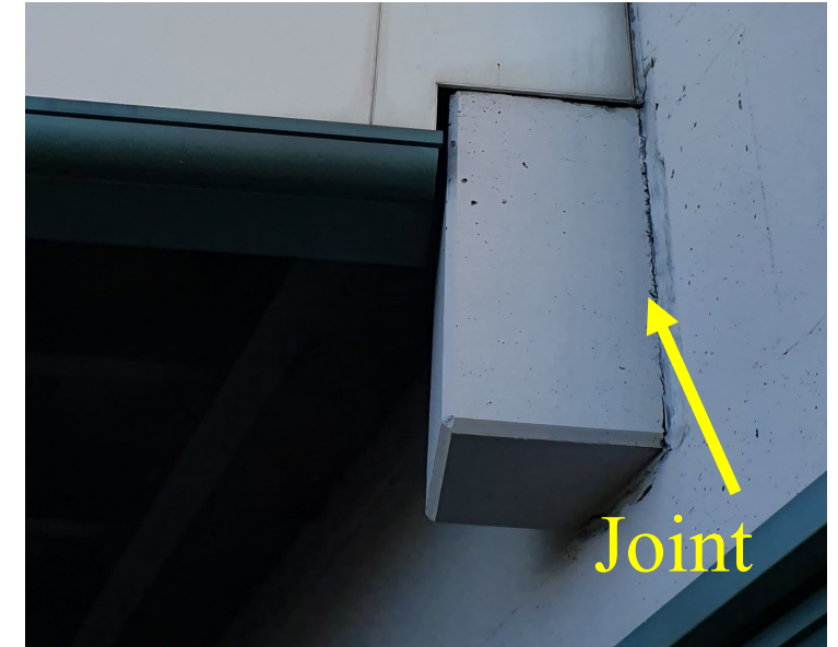
Donaghmede Entrance - Joint around corbel supporting footbridge
