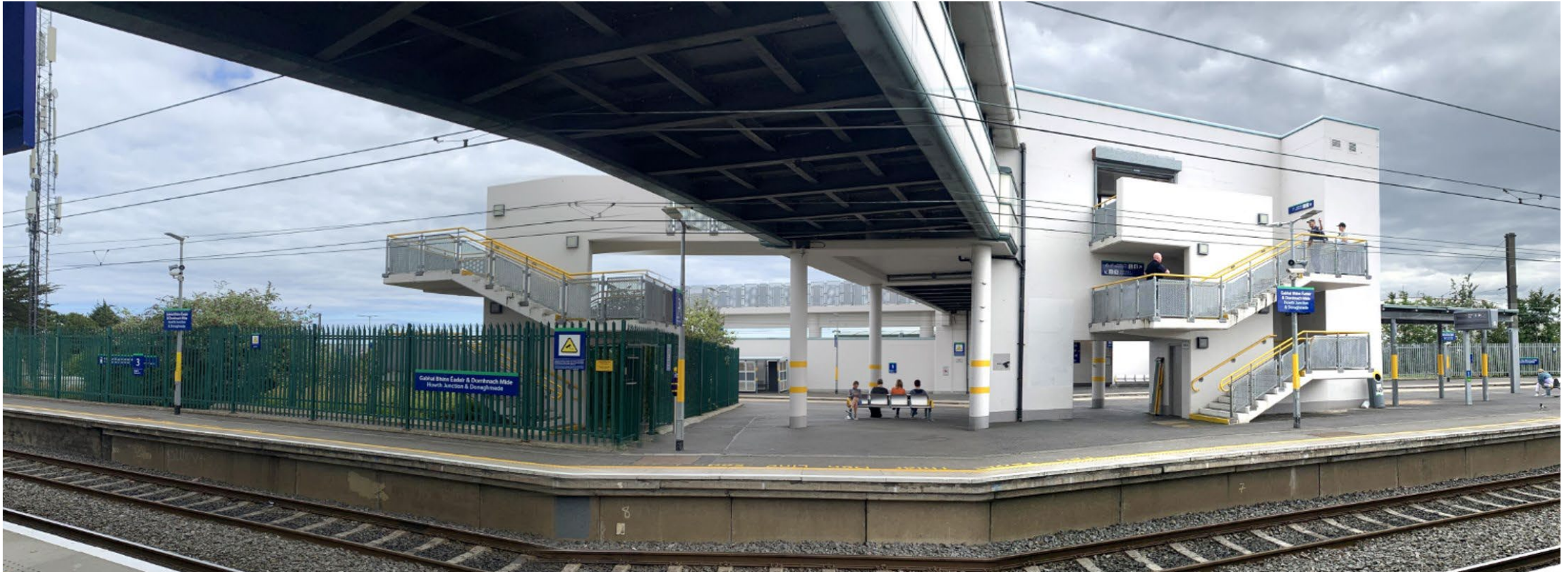
Photo of the existing Central Connection from Platform 4 demonstrating the poor visibility to Platforms 1 and 2
