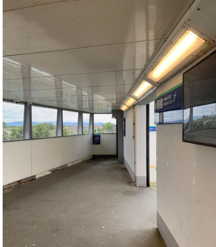
Photo of existing lift entrance at footbridge level
