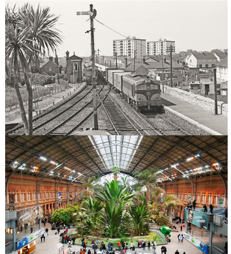
Station as a garden? Howth Junction 1977 | Madrid Atocha Station
