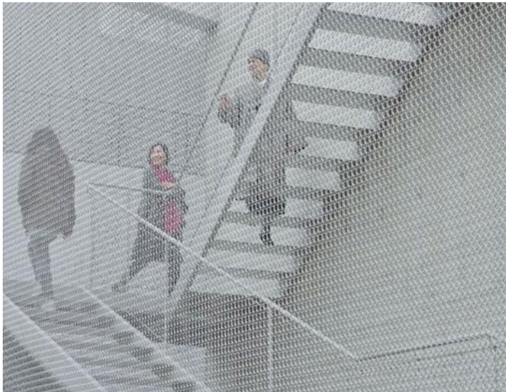
Architectural mesh applied to external stairs
