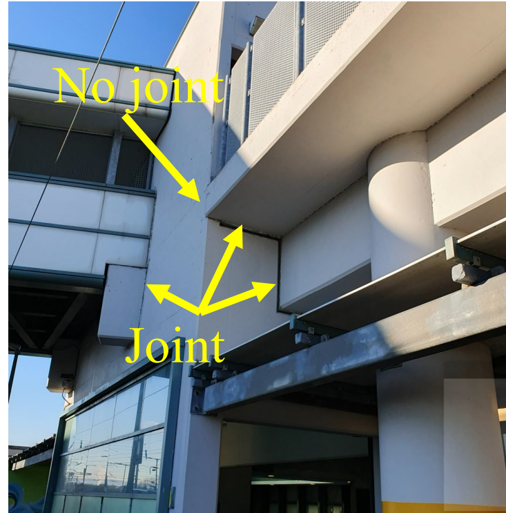
Donaghmede Entrance - Joints of footbridge support
