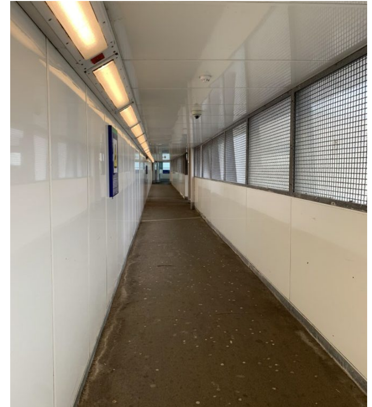
Photo of existing footbridge (station side)
