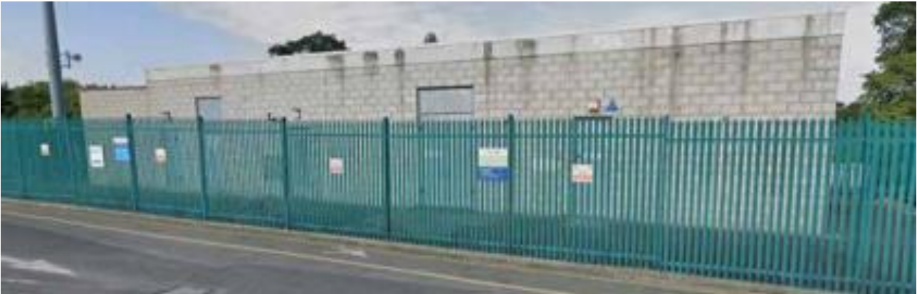
Figure 3-7: An example of a typical substation
