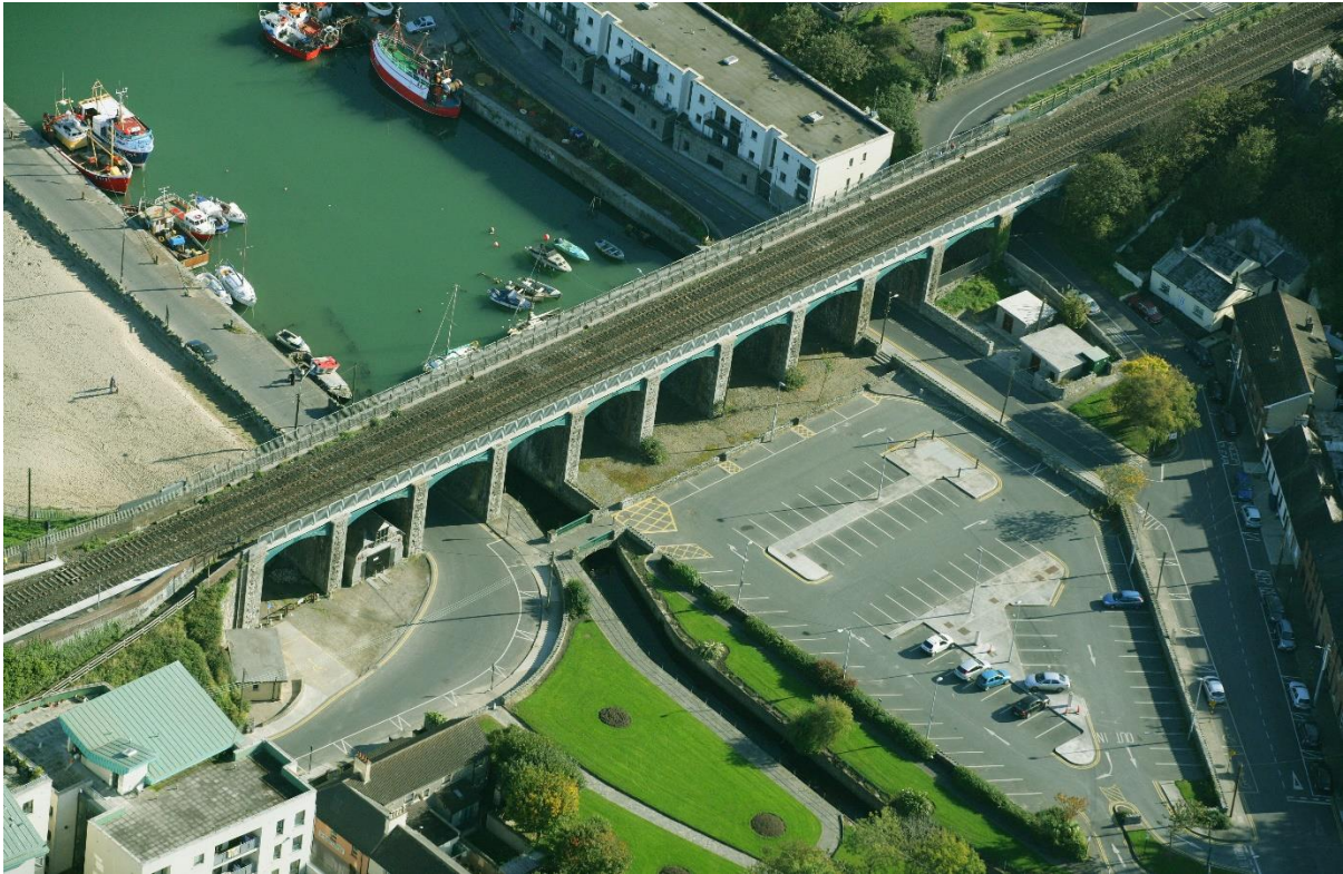
Figure 3-3: Balbriggan Viaduct UBB56 (© Peter Barrow Photography)
