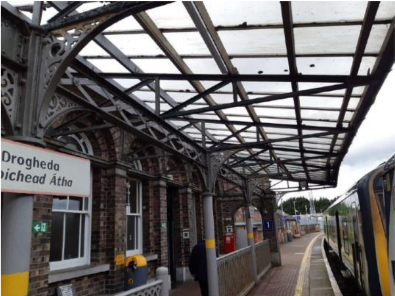
Figure 3-8: Drogheda Platform 1 Canopy
