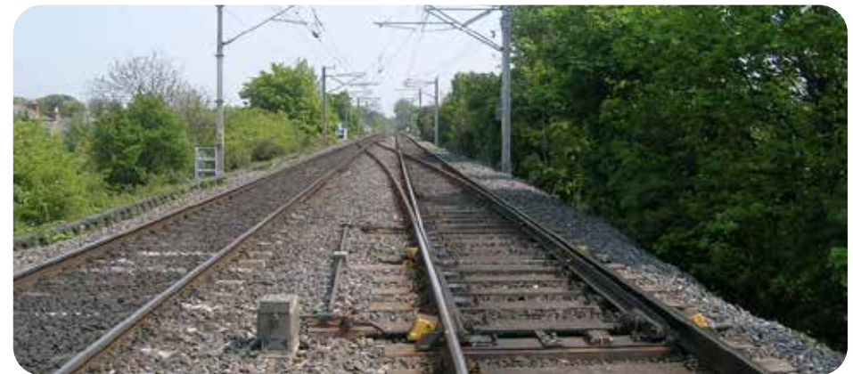
View of typical section of twin track electrified rail line
