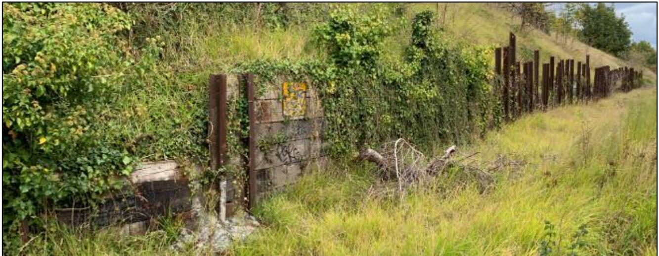
**Figure 2-7 King post retaining wall on the north side of the corridor between South Circular Road Bridge (OBC1) and Memorial Road Bridge (OBC3)**
