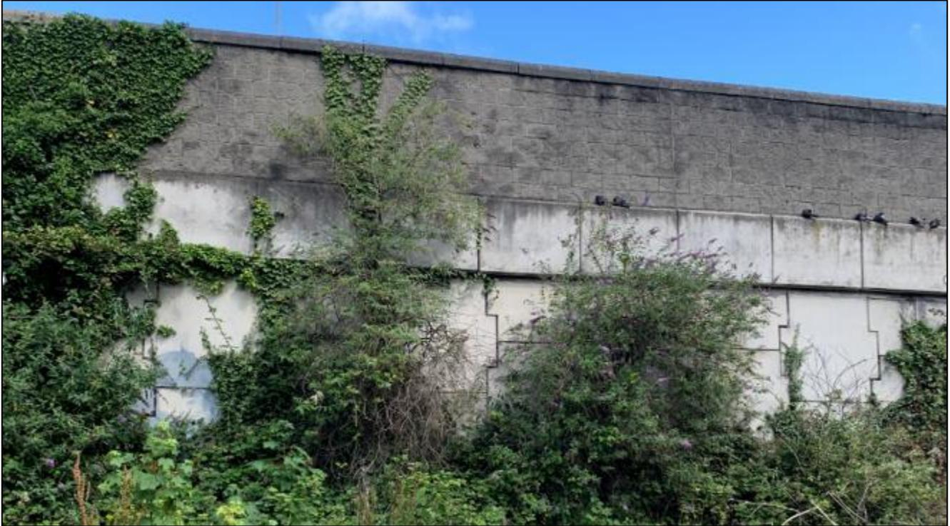
**Figure 2-5 MSE retaining wall on the north side of the corridor between South Circular Road Bridge (OBC1) and St. John’s Road Bridge (OBC0A)**
