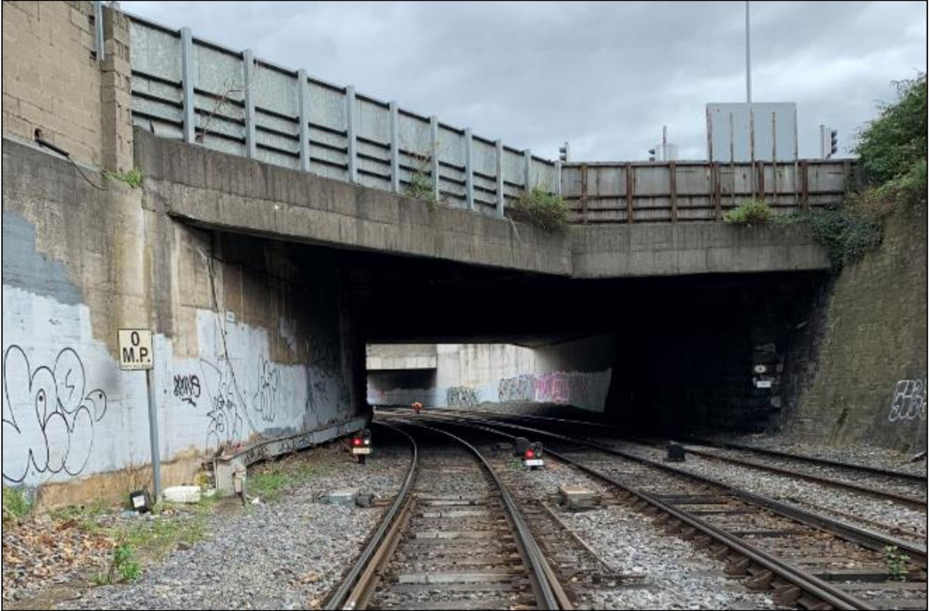
**Figure 2-10 Tight horizontal radius and reduced sight distance at South Circular Road Bridge (OBC1) - Facing East**
