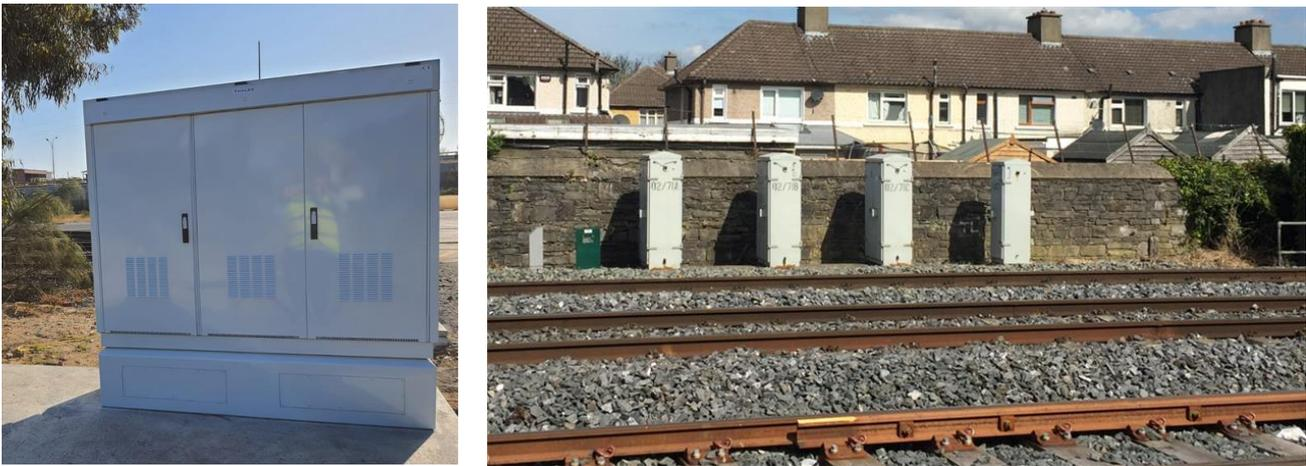
**Figure 7-14 Typical Object Controller Cabinet (OBJ) and Location Case**
