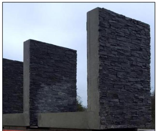
**Figure 7-5 Precast panels fully clad with masonry**
