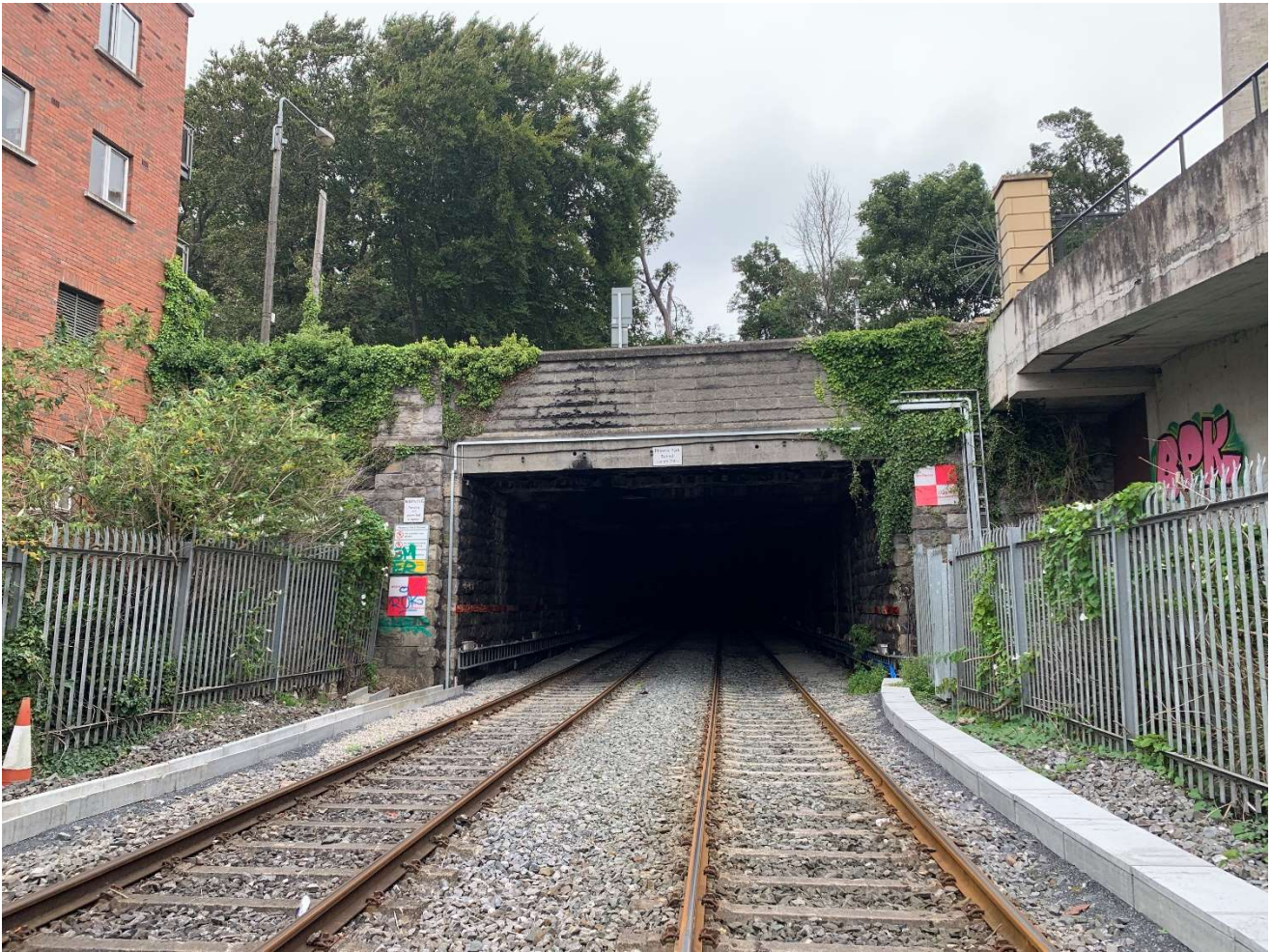
Figure 2-4 Conyngham Road Bridge (OBO2) – Southern Elevation
