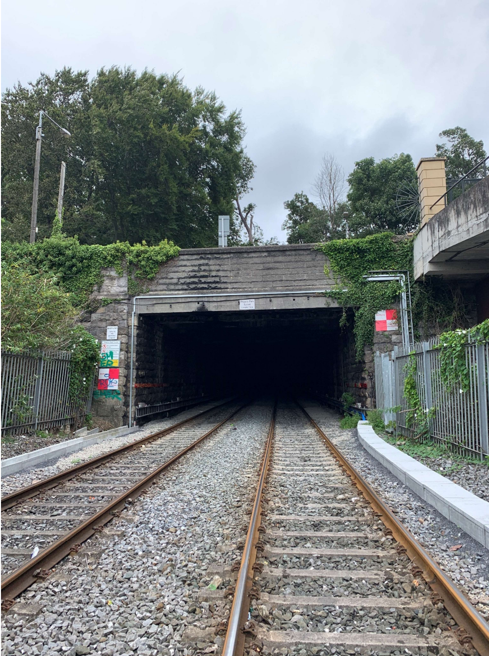
Figure 2-9 Conyngham Road Bridge (OBO2) / Phoenix Park Tunnel South Portal
