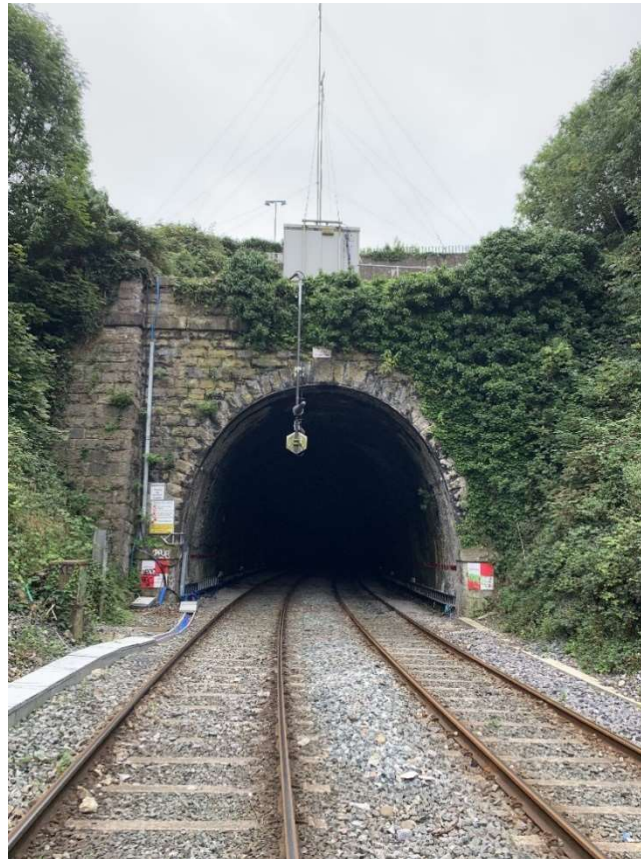
Figure 2-5 Phoenix Park Tunnel, North Portal
