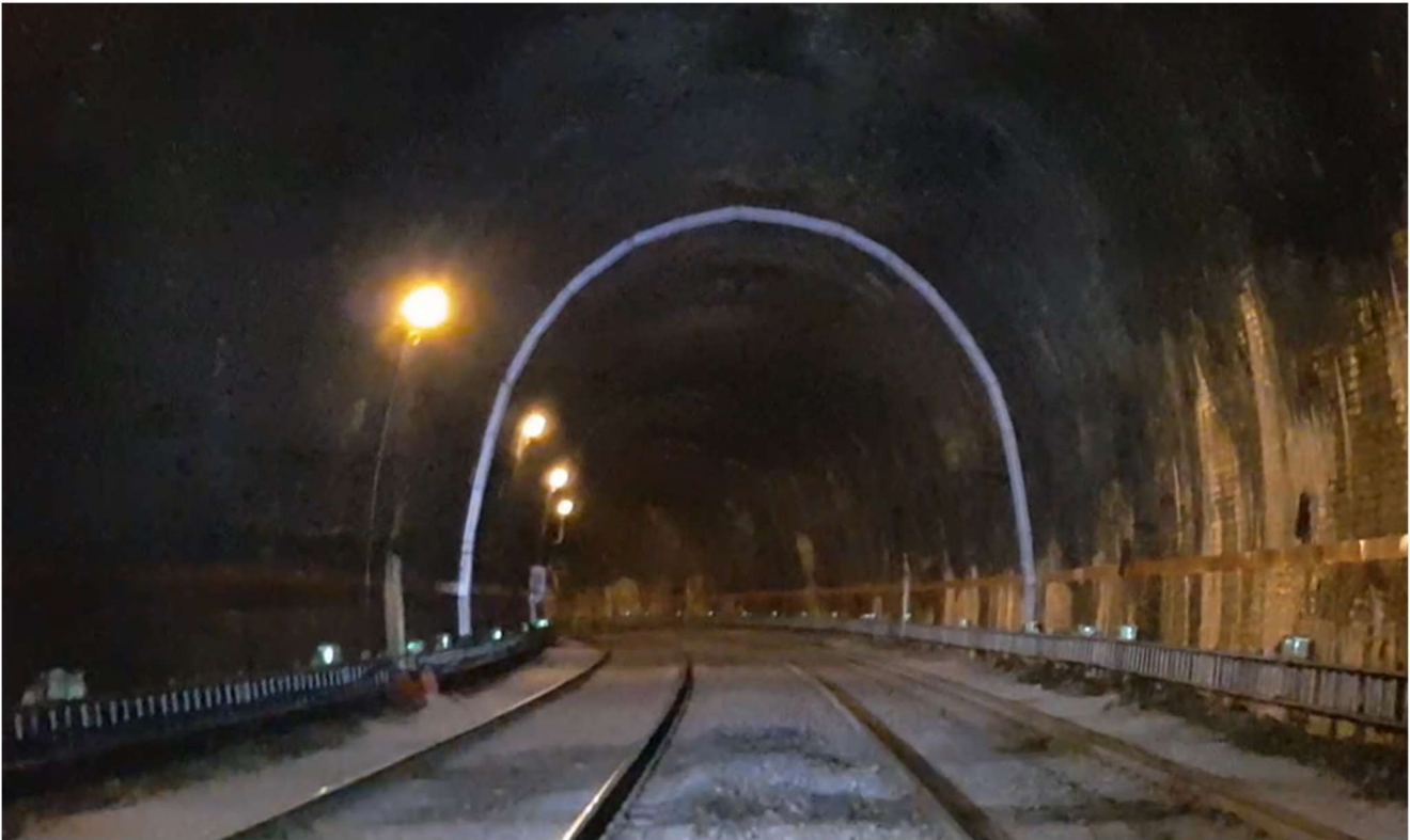
Figure 2-10 View of Phoenix Park Tunnel.
