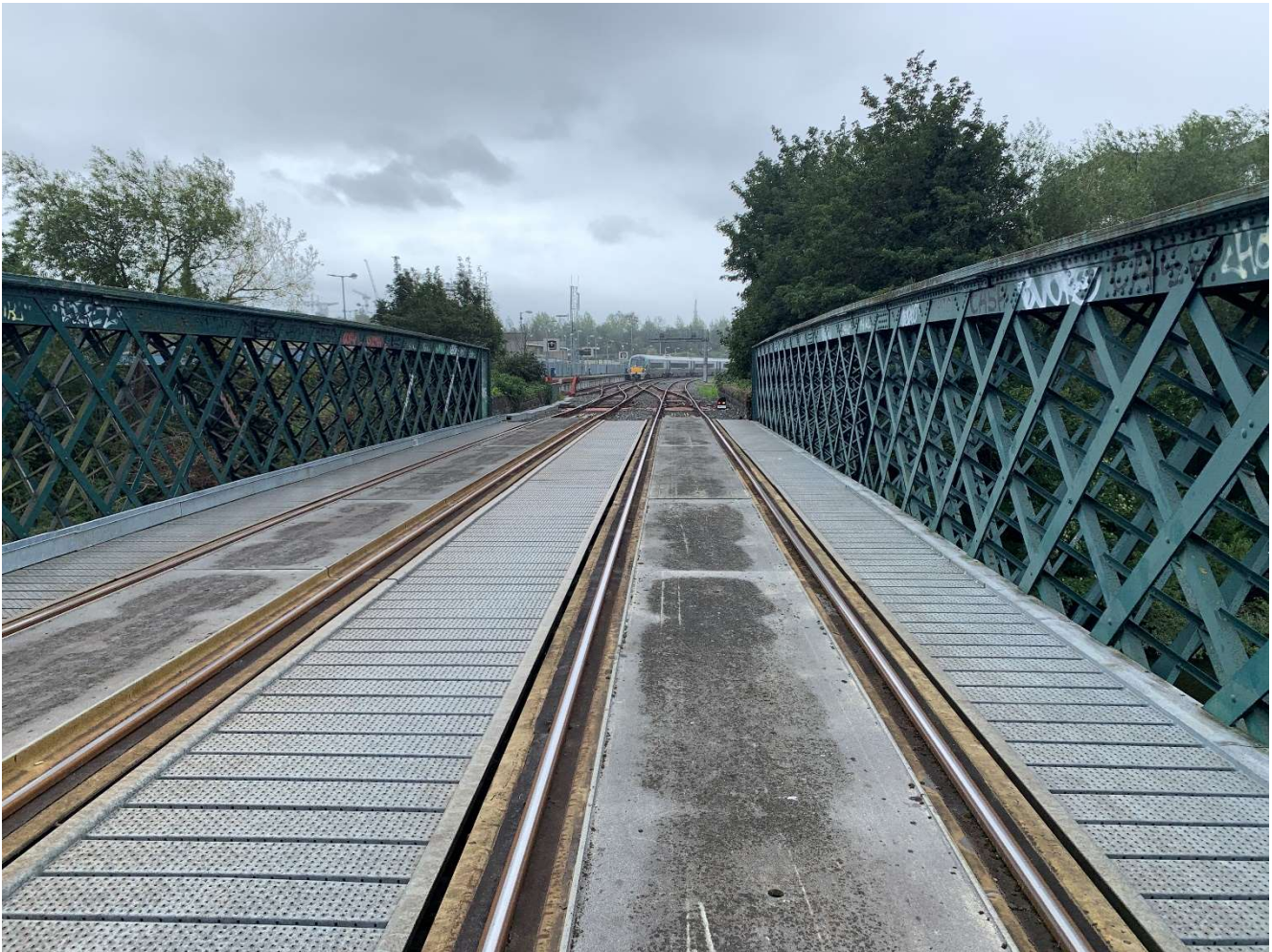
Figure 2-3 Liffey Bridge (UBO1) (Deck Level – Facing South)
