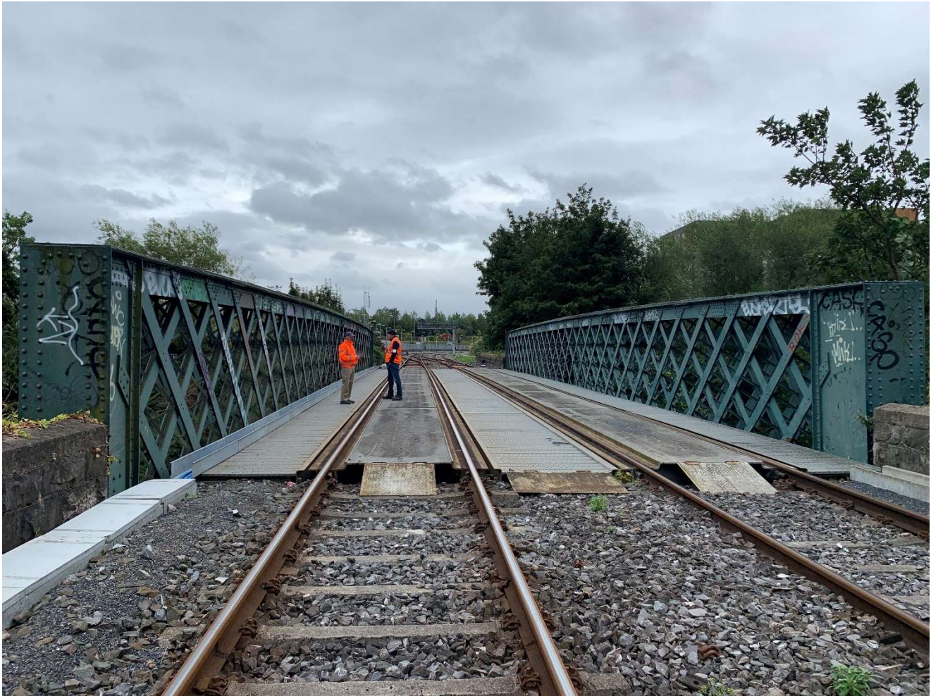
Figure 2-8 Liffey Bridge (UBO1) fixed rail restraint
