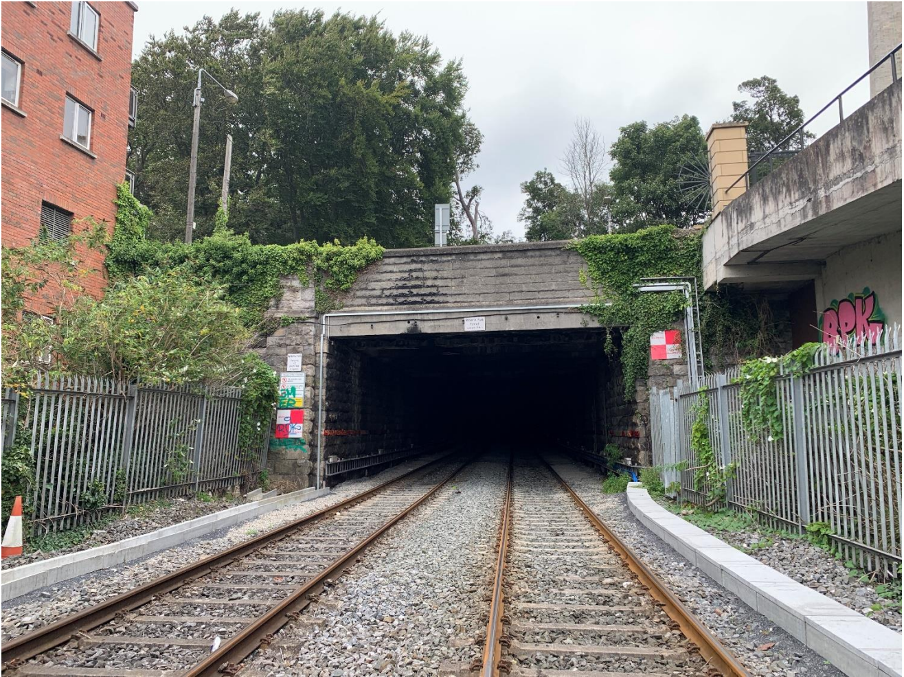
Figure 2-3 Conyngham Road Bridge (OBO2) – Southern Elevation
