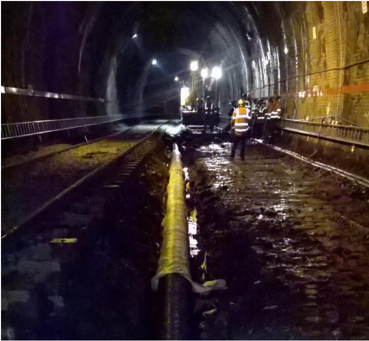
Figure 2-14 Existing 300mm perforate pipe at Phoenix Park Tunnel
