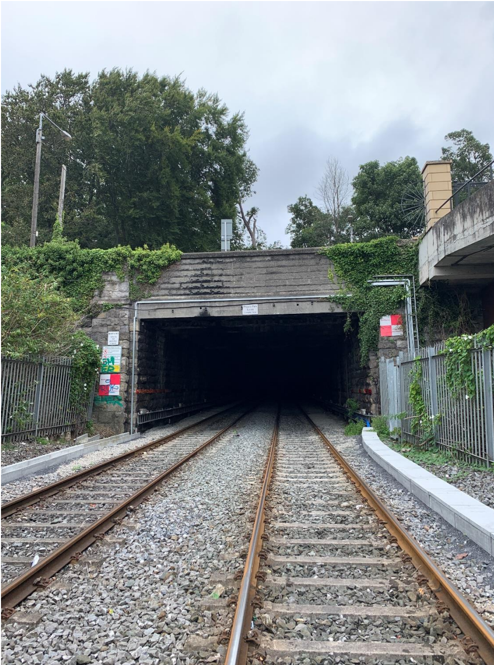
Figure 2-8 Conyngham Road Bridge (OBO2) / Phoenix Park Tunnel South Portal
