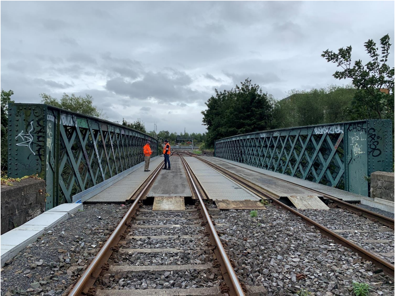
Figure 2-7 Liffey Bridge (UBO1) fixed rail restraint - Facing South
