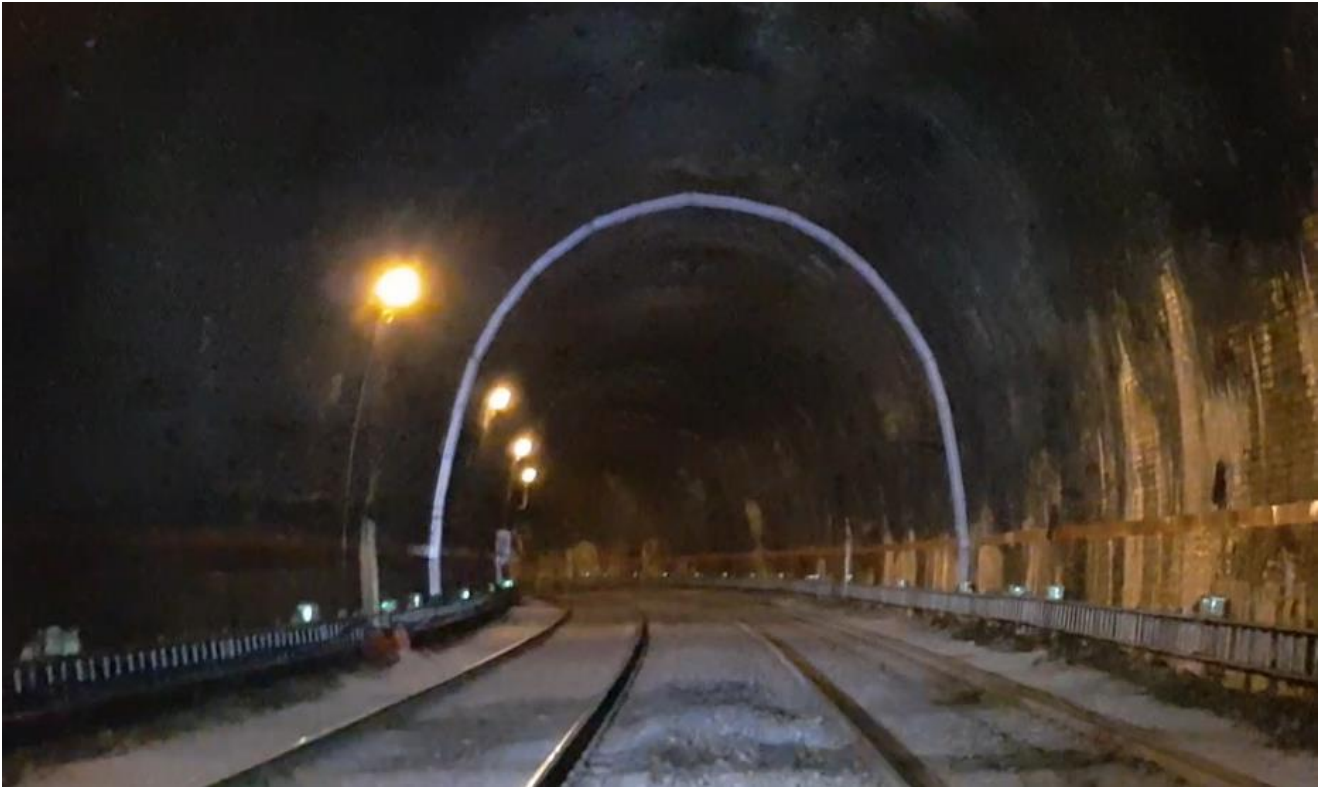
Figure 2-9 View of Phoenix Park Tunnel.
