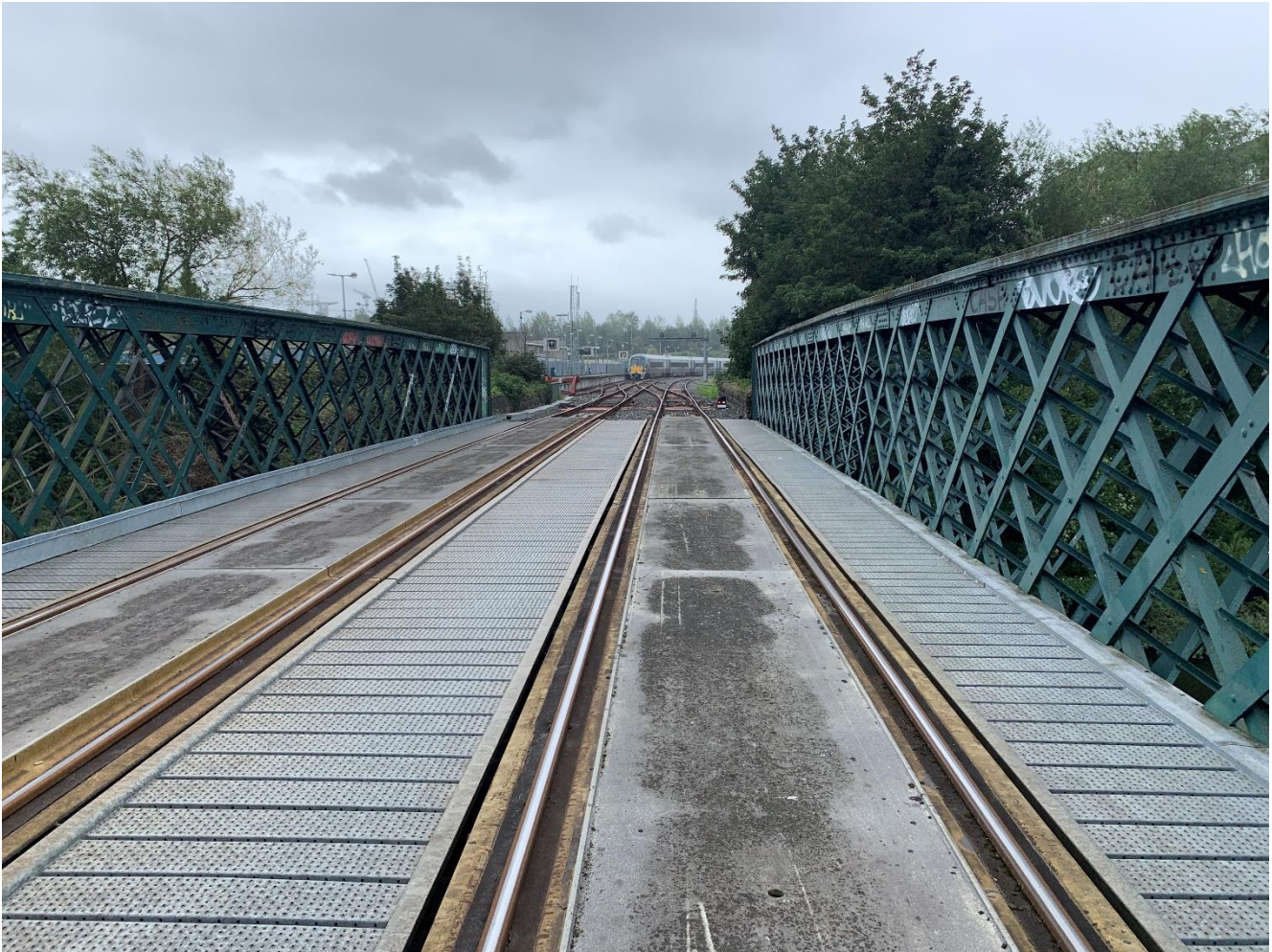
Figure 2-2 Liffey Bridge (UBO1) (Deck Level – Facing South)
