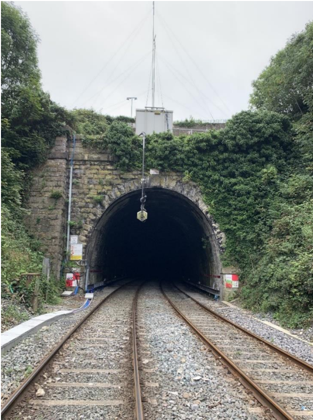
Figure 2-4 Phoenix Park Tunnel, North Portal
