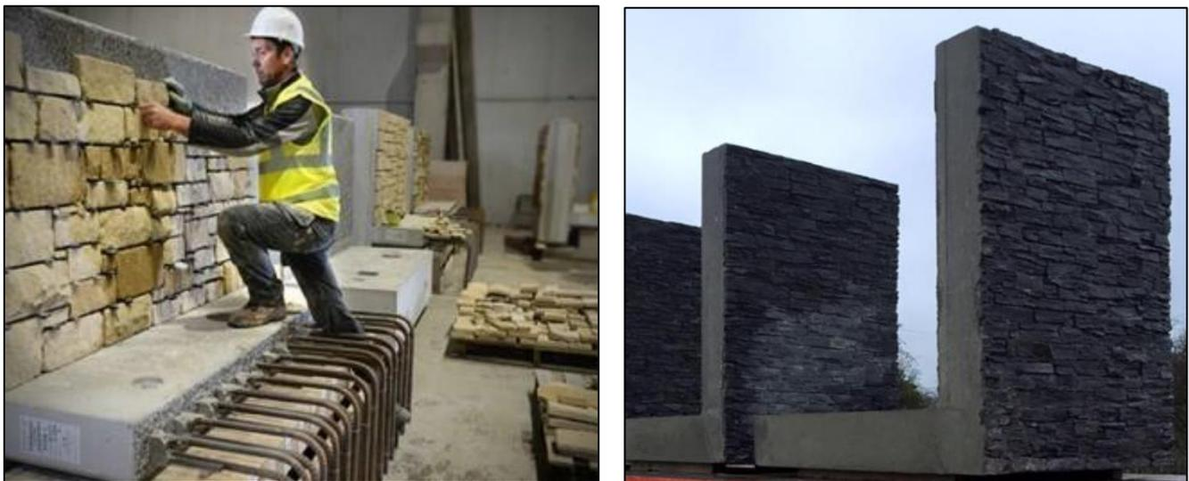
**Figure 7-5 Precast panels fully clad with masonry**
