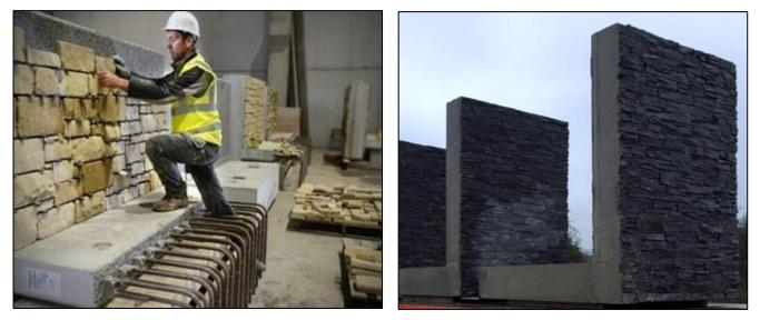
Figure 7-5 Precast panels fully cladded with masonry
