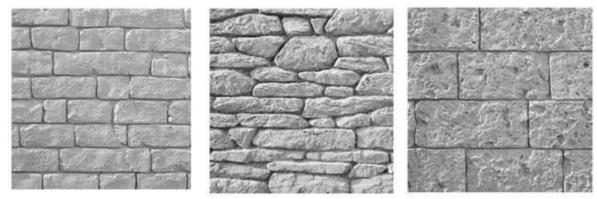
Figure 7-4 Parapets and/or H4a containment wall finishes for precast concrete
