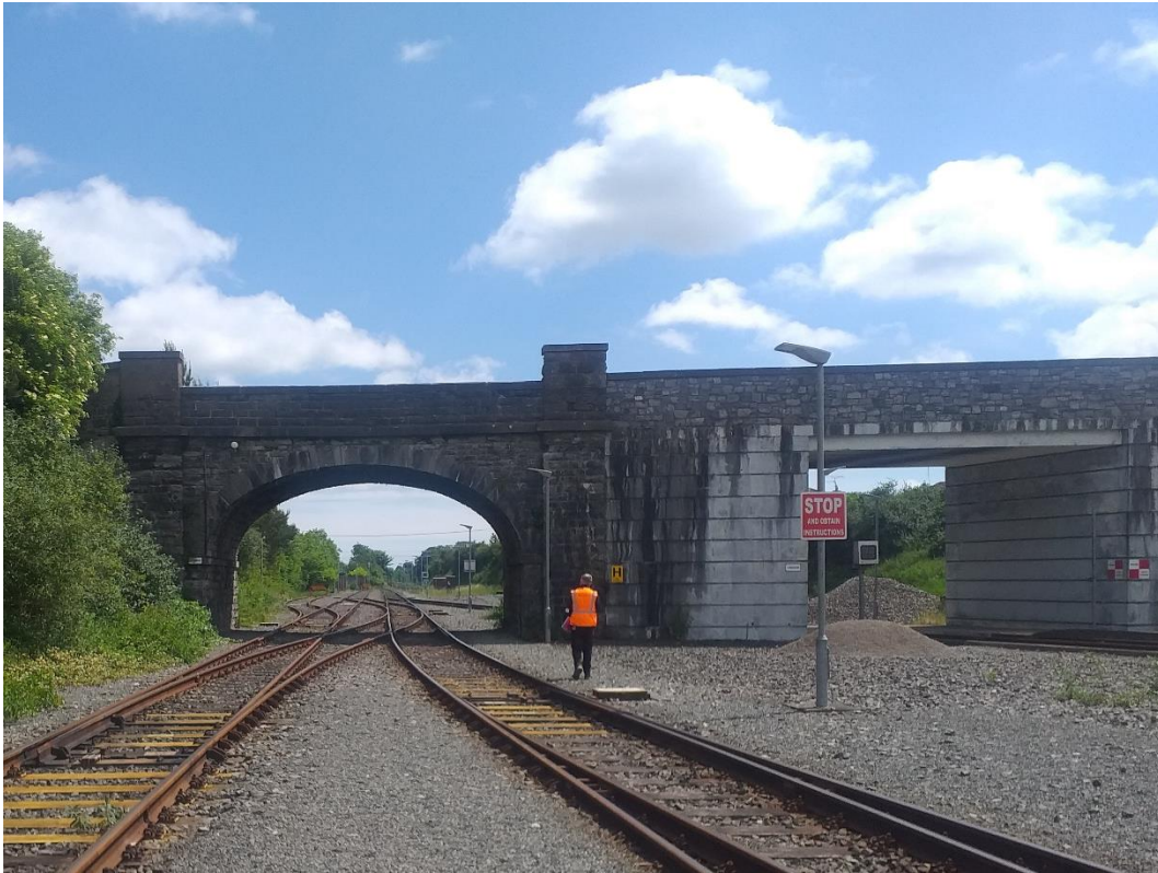
Figure 2-4: OBB80A (left) and OBB80B (right) from track level
