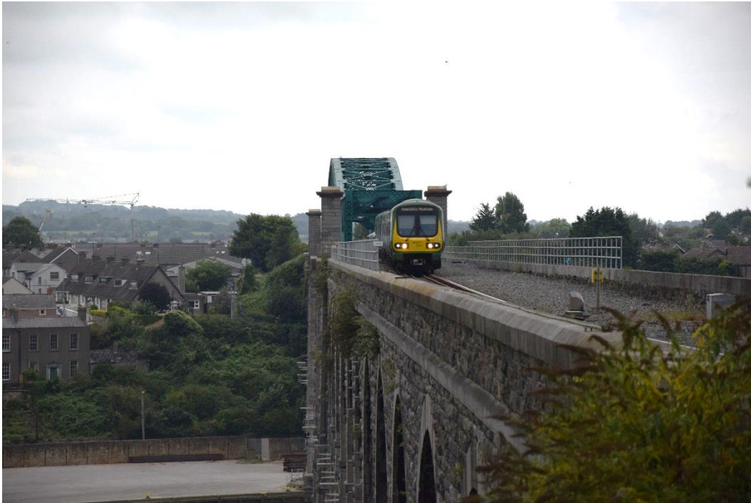
Figure 2-10: UBB82 Boyne Viaduct (Protected Structure LCC RPS DB-176)
