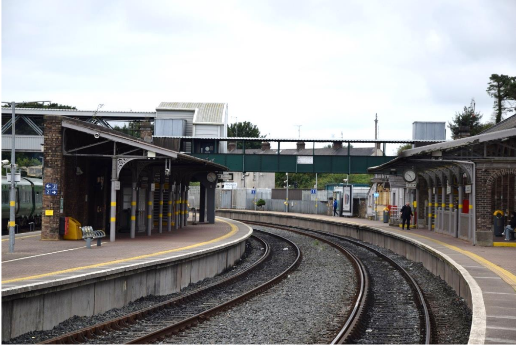
Figure 2-6: OBB81 Drogheda MacBride Station footbridge
