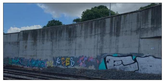
Figure 2-6 RC retaining wall on the south side of the corridor between South Circular Road (OBC1) and St. John's Road Bridge (OBC0A)
