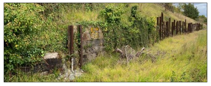
Figure 2-7 King post retaining wall on the north side of the corridor between South Circular Road Bridge (OBC1) and Memorial Road Bridge (OBC3)
