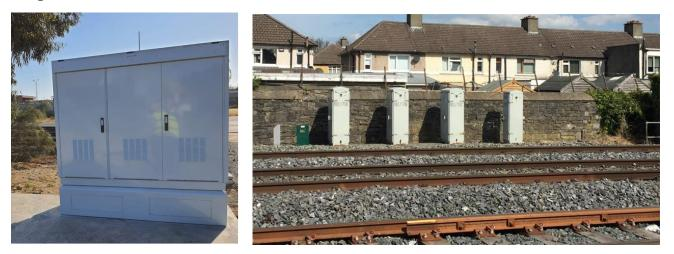
Figure 7-14 Typical Object Controller Cabinet (OBJ) and Location Case
