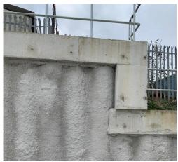
Figure 7-6 Example of a Secant Wall
