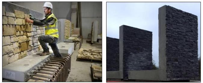
Figure 7-5 Precast panels fully cladded with masonry
