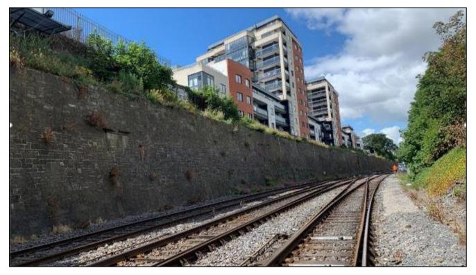
Figure 2-4 Masonry retaining wall along the south side of rail corridor - Facing West
