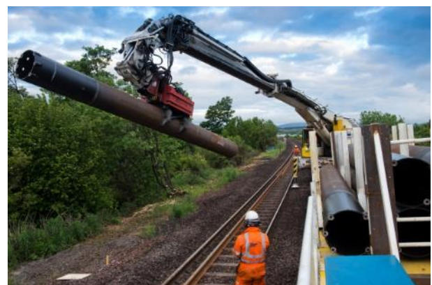
Figure 7-6 Option 1: Steel Pile Driven Foundations
