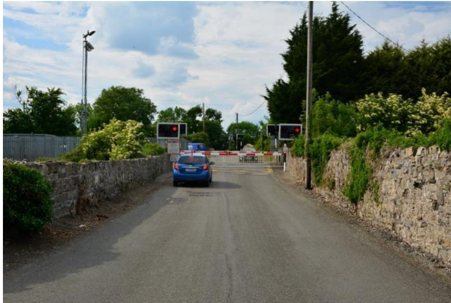
Figure 9-16 Barberstown Level Crossing
