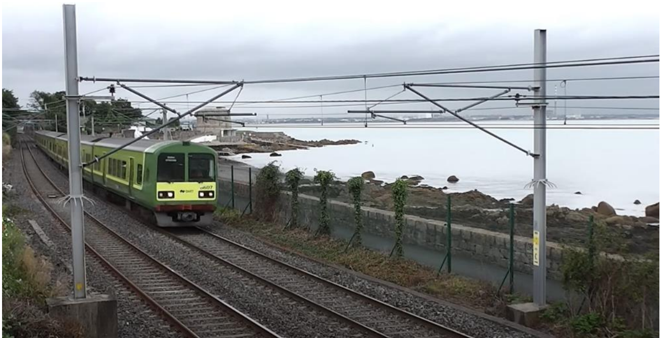
Figure 1-2 View of Typical Electrified section of Southern Line
