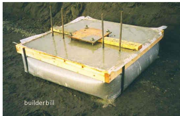
Figure 7-8 Option 3: Concrete PAD foundations
