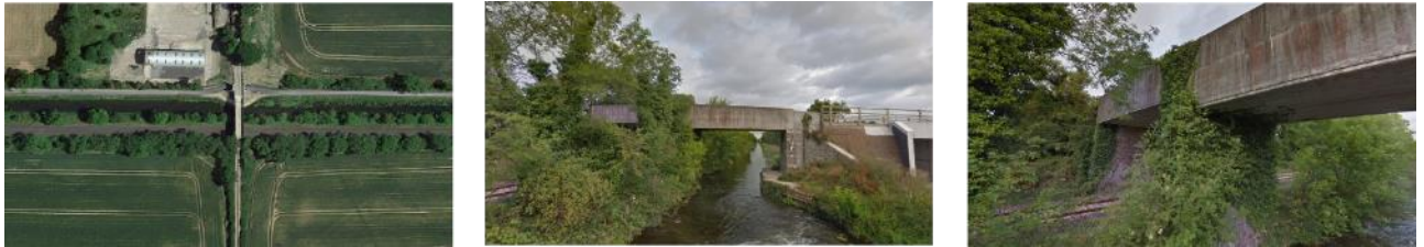
Figure 10-1 Existing OBG24 to be demolished
