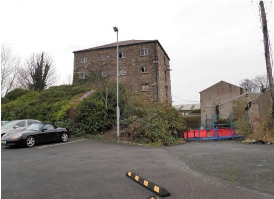
Figure 9-3 View of Old Mill to the southwest of the existing Level Crossing
