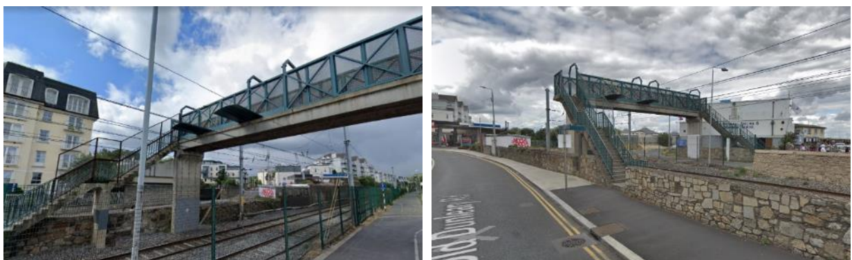
Figure 7-10 OHLE Protection Option 2: Safety Screens
