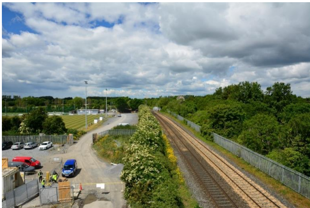
Figure 9-10 Porterstown Level Crossing
