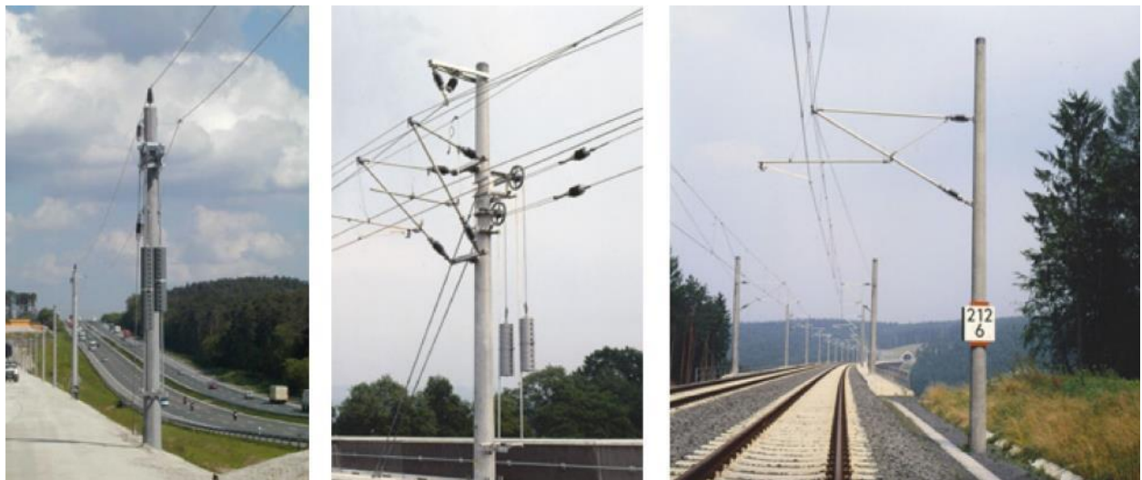
Figure 7-4 OHLE Structure Option 2: Circular Profiles
