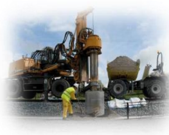
Concrete Bored Pile Foundations
