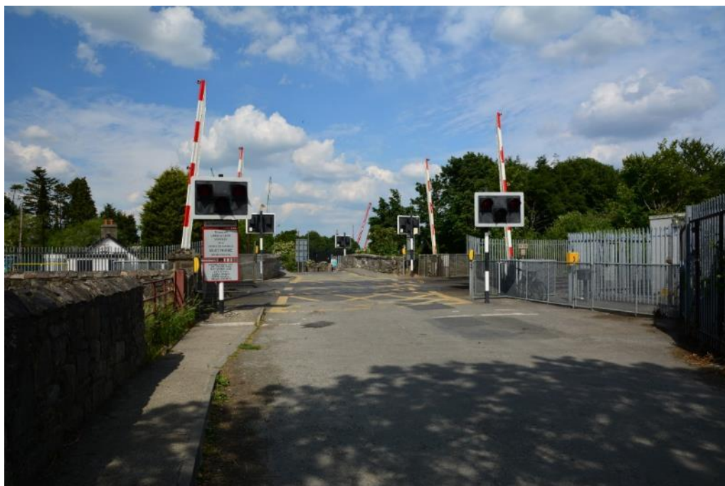
Figure 9-20 Blakestown Level Crossing
