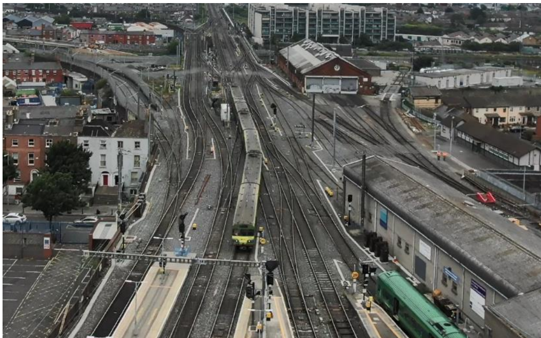
Figure ES-4 Connolly Station looking North
