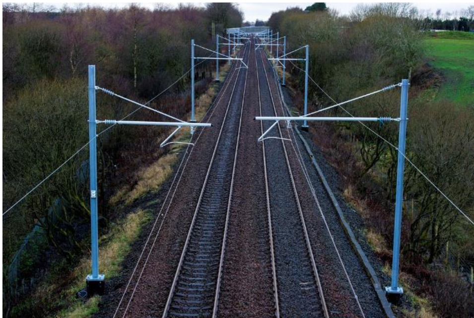
Figure 7-3 OHLE Structure Option 1: HEB Steel Beams
