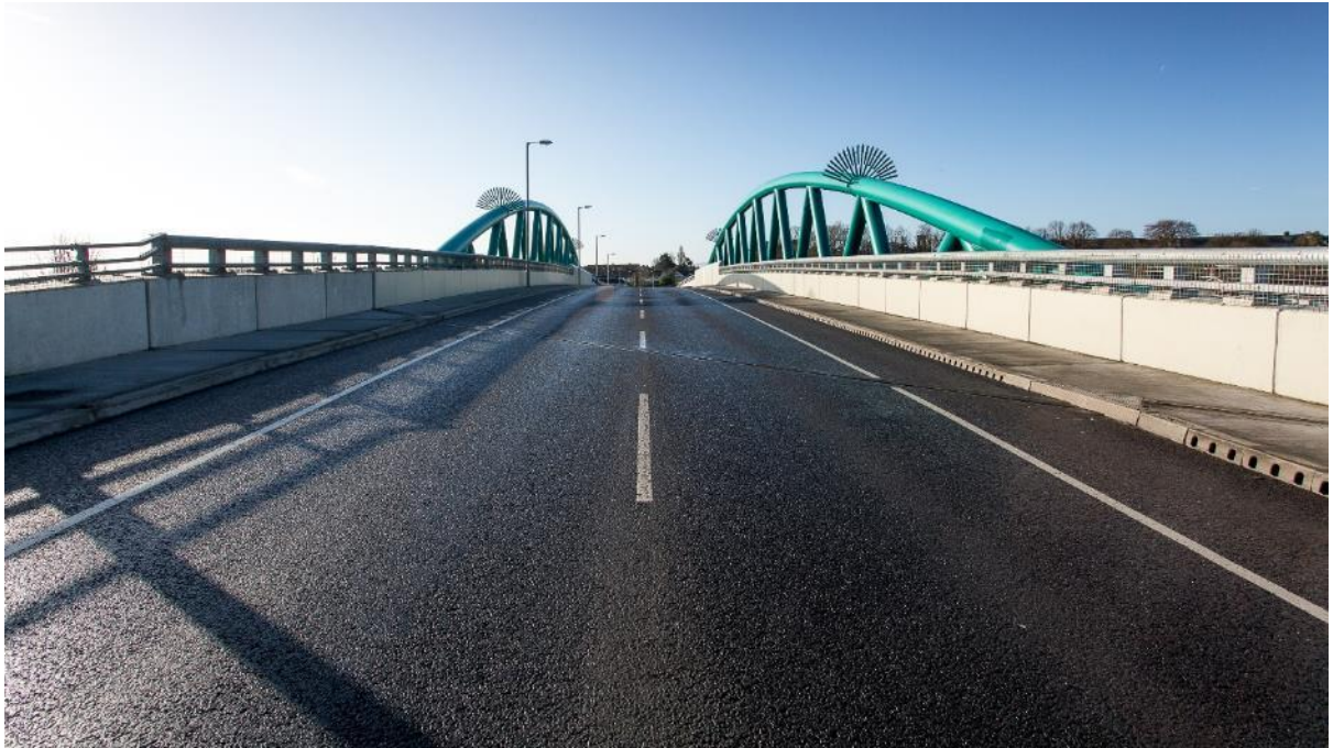
Figure 2-3 After: The overhead bridge constructed at Ratoath Road in 2018
