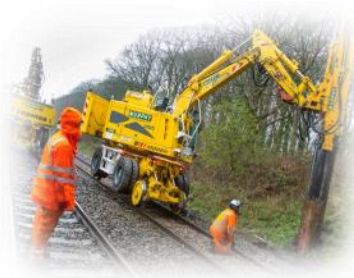
Steel Pile Driven Foundations
