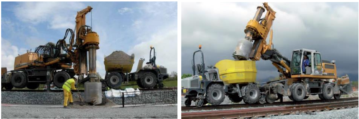
Figure 7-7 Option 2: Concrete Bored Pile Foundations
