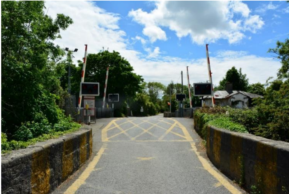
Figure 9-9 Porterstown Level Crossing
