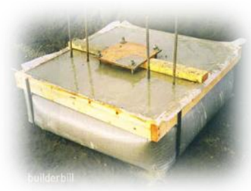
Concrete PAD Foundations
