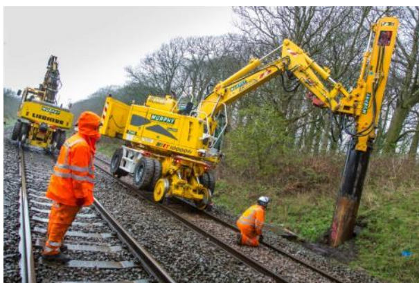
Figure 7-6 Option 1: Steel Pile Driven Foundations
