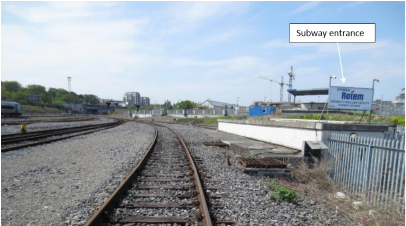
Figure 2-3 Valeting Plant Subway (UBC1A) north entrance
