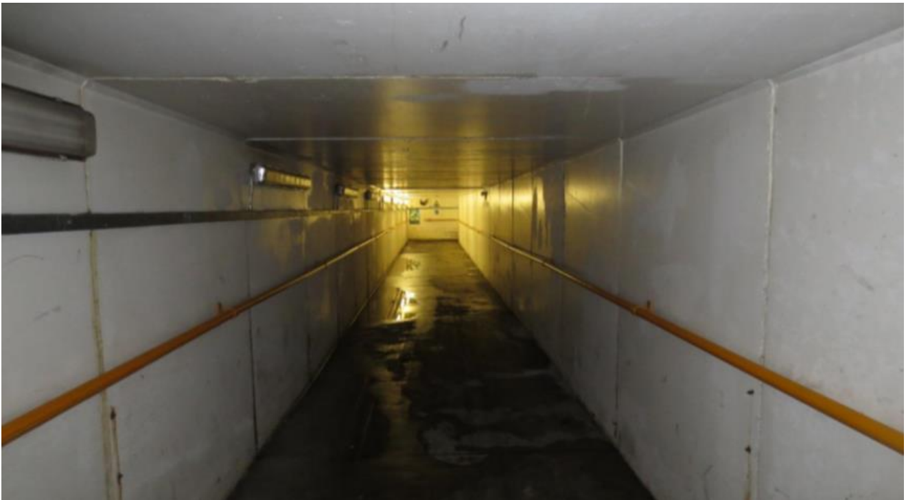
Figure 2-2 Valeting Plant Subway (UBC1A) under the railway tracks
