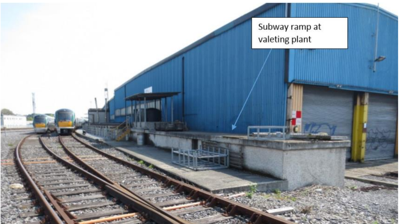
Figure 2-4 Valeting Plant Subway (UBC1A) south entrance
