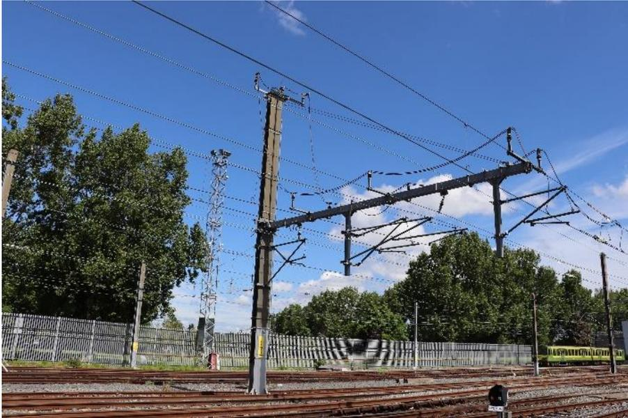
**Figure 3-1: Example of existing OHLE cantilever support**
