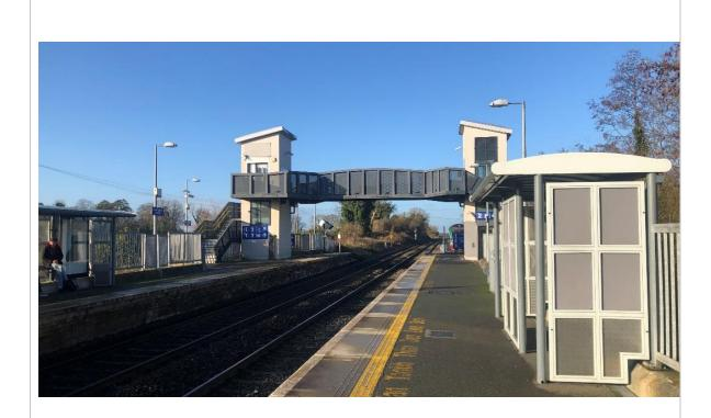
PHOTO 7 - Footbridge connecting both platforms with lifts.
