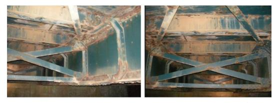
Figure 7-7: Intermediate pier diaphragm with plan bracing (source: Iarnród Éireann)
