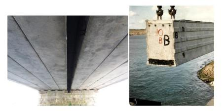
Figure 4-4: UBB36 Erection of precast beams (left) and soffit (right) (Source IÉ)
