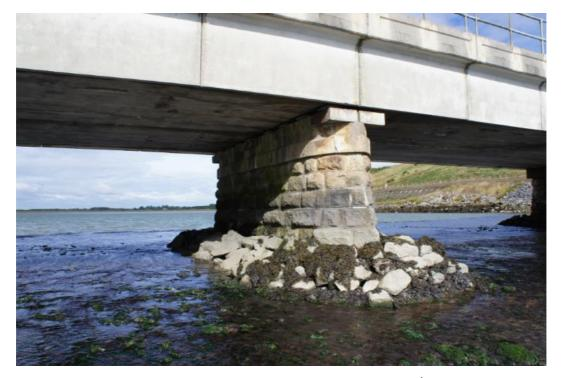
Figure 4-6: UBB36 Protected piers and replaced deck (source: IÉ)
