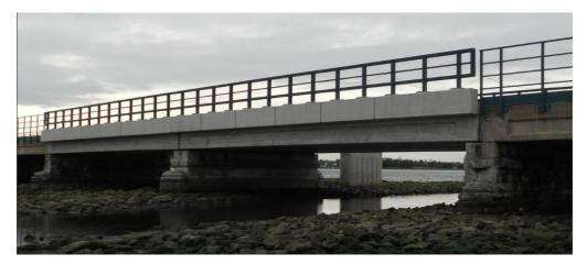
Figure 3-5: UBB30 replaced spans (4 and 5) and reconstructed Pier 4 (source: Iarnród Éireann)
