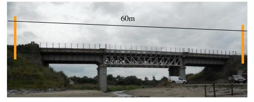
Figure 6-8: Proposed OHLE frame location – arrangement 1 (source: Iarnród Éireann)
