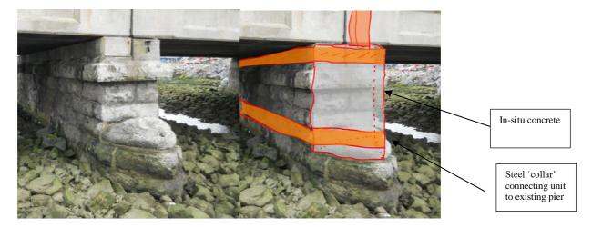
Figure 3-19: Sketches of Option 1 of proposed OHLE transverse arrangement (source: Iarnród Éireann)
