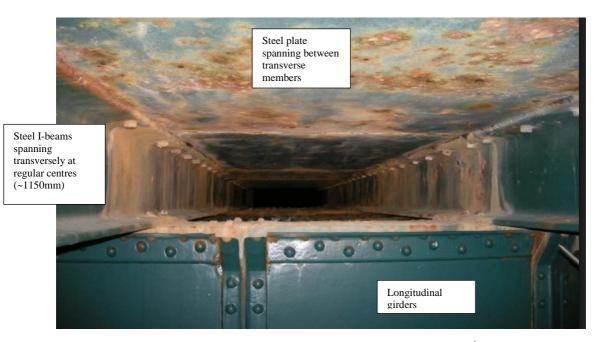
Figure 7-3: UBB72 deck steelwork arrangement (source: Iarnród Éireann)
