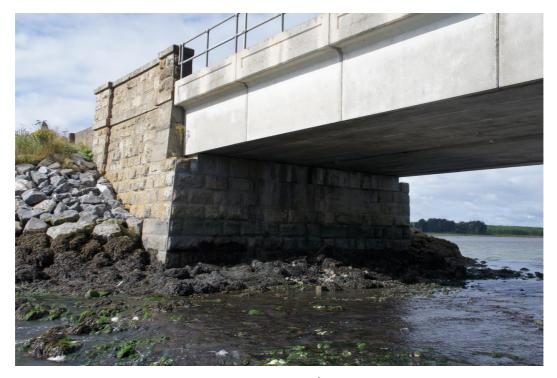
Figure 4-3: UBB36 Abutment (source: Iarnród Éireann)
