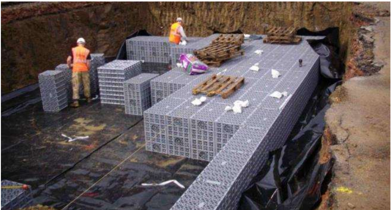
Figure 5-8 Typical Modular Attenuation Tank
