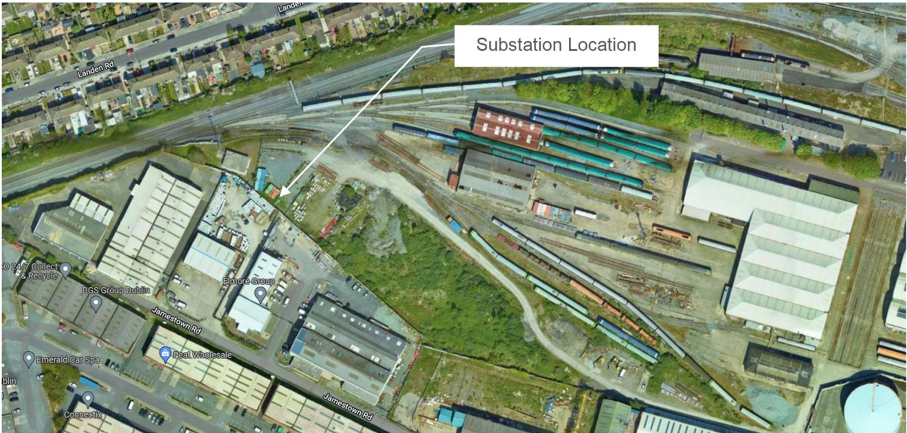
Figure 5-72 Kylemore Substation Location
