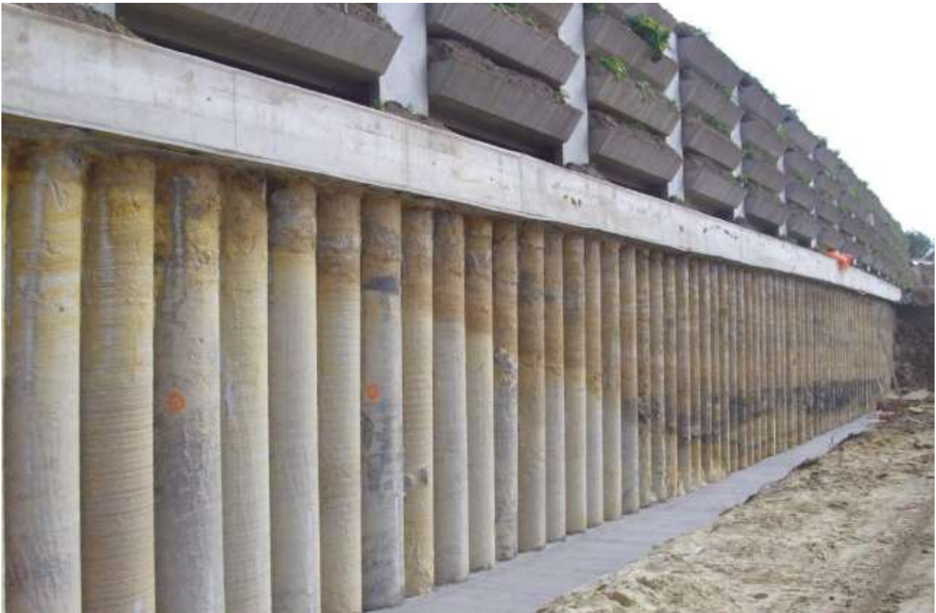
Figure 5-2 Example of a Bored Pile Wall
