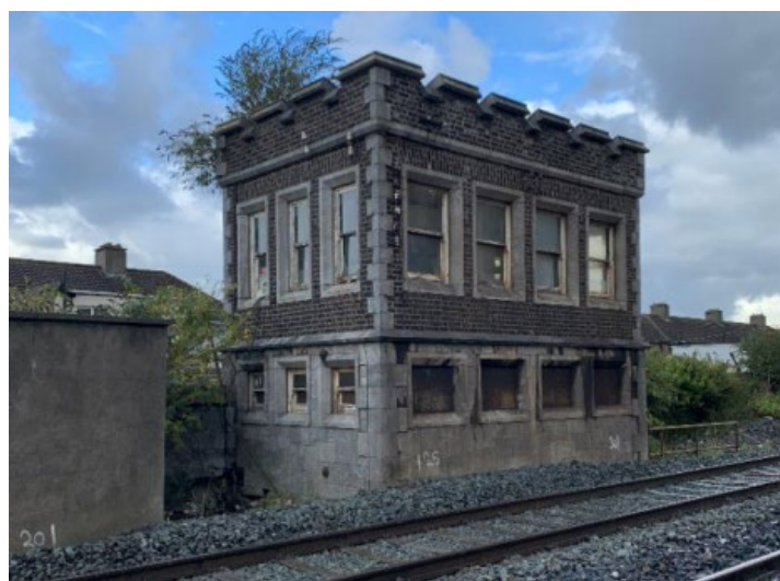
Figure 4-20 Old Signal Box - Inchicore Depot
