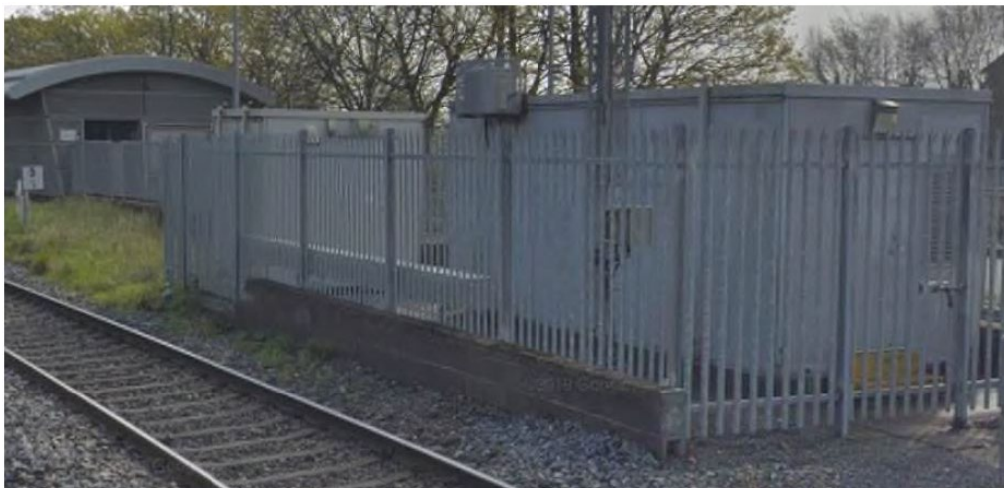
Figure 4-8 Typical Telecom Equipment Building
