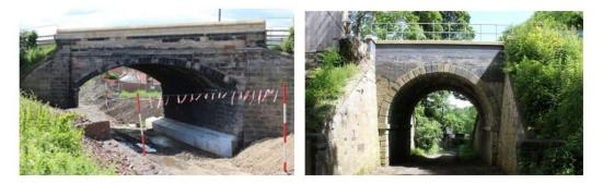
Figure 4-2: Raised parapet wall on masonry arch bridge (Borders Railway Project, Newtongrange to Eskbank)
