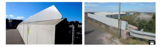
Figure 4-5: Non-transparent parapet extensions (Steel – Bury's Bridge, UK and GFRP example (source www.duracomposites.com)
