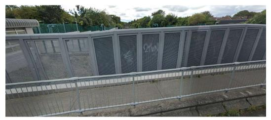
Figure 4-8: Steel panels added to outer face of existing mesh screens (Middle Third Bridge, Killester)
