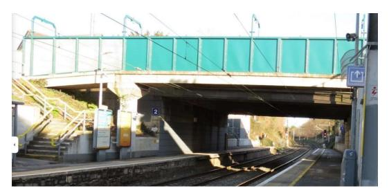
Figure 4-7: Mesh infill replaced with solid steel panels (Raheny Station footbridge)
