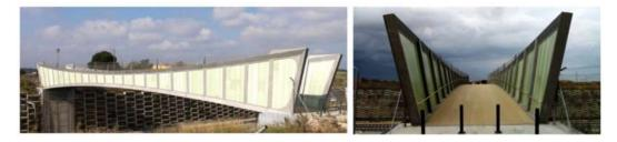
Figure 4-11: GFRP panels between chords of Vierendeel truss (Vilafant footbridge, Spain)
