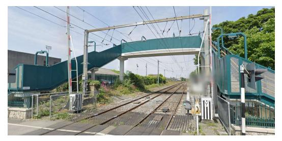
Figure 4-9: Solid steel panels on pedestrian bridge (OBR141, Bray)
