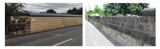
Figure 4-3: Coping extension (GFRP coping – Stockton on Tees Junction (source:www.evergrip.com) and precast concrete – Borders Railway Project, Bonnyrigg Road Bridge)
