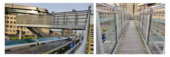
Figure 4-10: Clear panels on pedestrian bridge (Grand Canal Dock Station)
