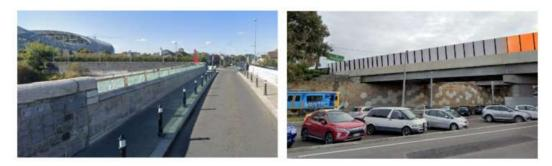
Figure 4-6: Transparent or opaque parapet extensions (Glass – Dodder Bridge, Ringsend and Polycarbonate or Acrylic – Eastlink, Australia). Note that Section 4.3 of this report discusses relevant materials and recommends against the use of glass.
